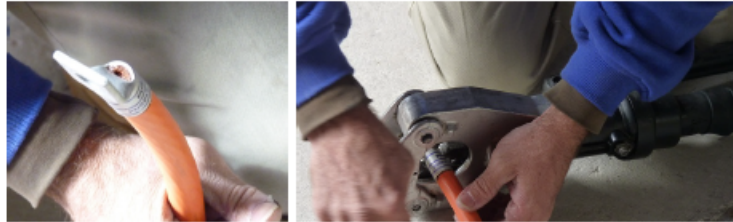
Figure 3-2. Installing Compression Lugs
