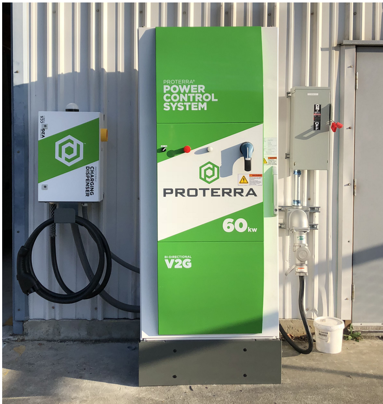
Figure 2-1. Charge System Equipment Installation Overview
