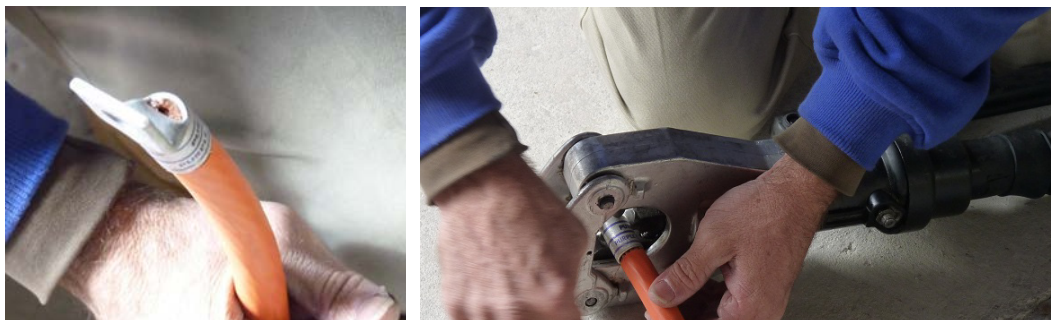
Figure 3-2. Installing Compression Lugs
