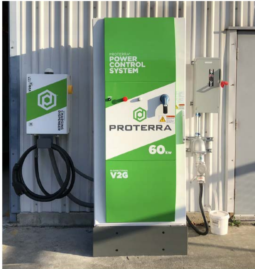
Figure 2-1. Charge System Equipment Installation Overview
