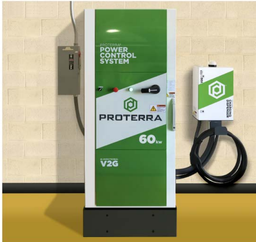
Figure 2-2. Typical Installation of PCS
