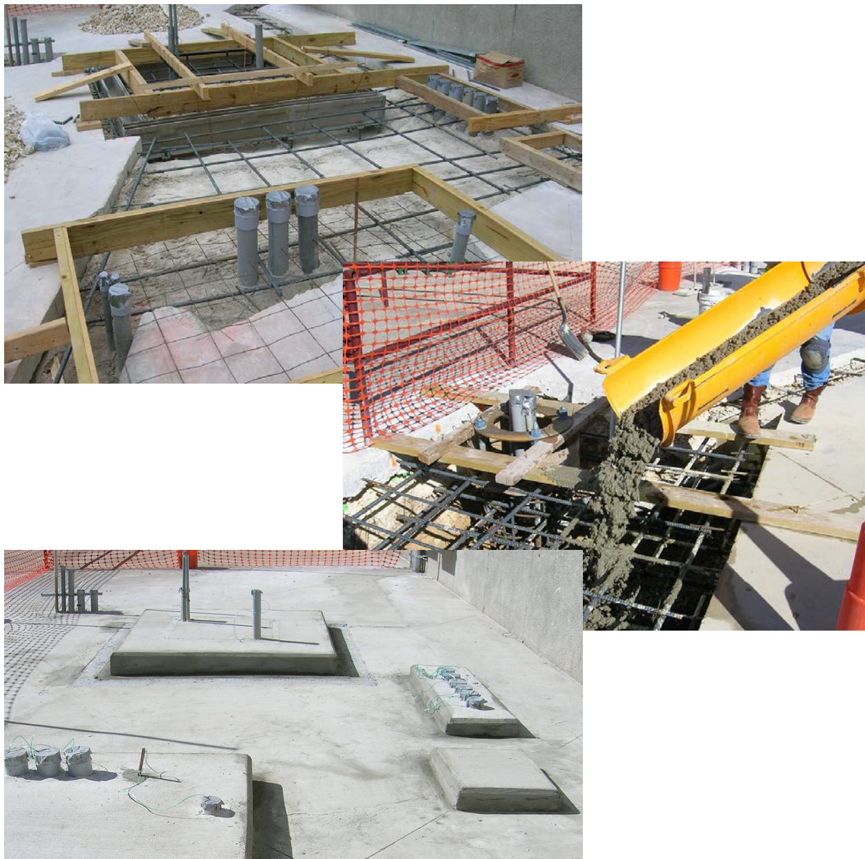
Figure 1-5. Site Preparation Work
