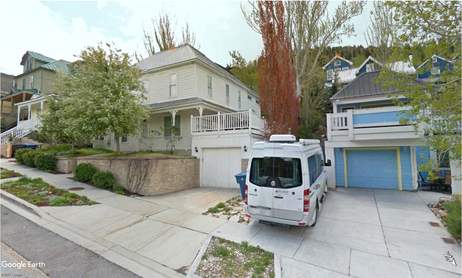
WITHOUT APPROVED STRUCTURE
