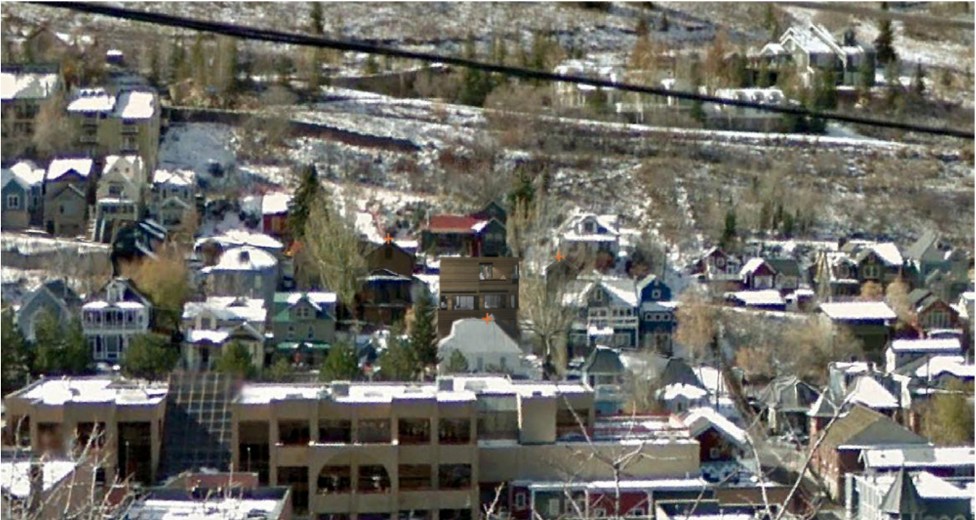
VIEW OF APPROVED STRUCTURE FROM ACROSS THE CANYON
