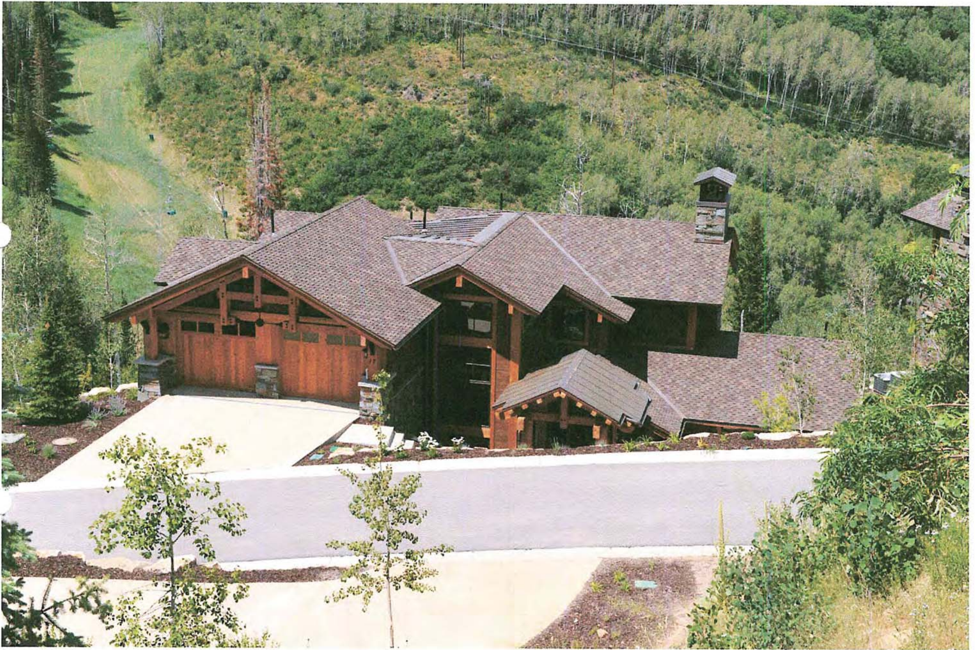
Unit 7 (17 Nakoma Terrace) – looking northwesterly
