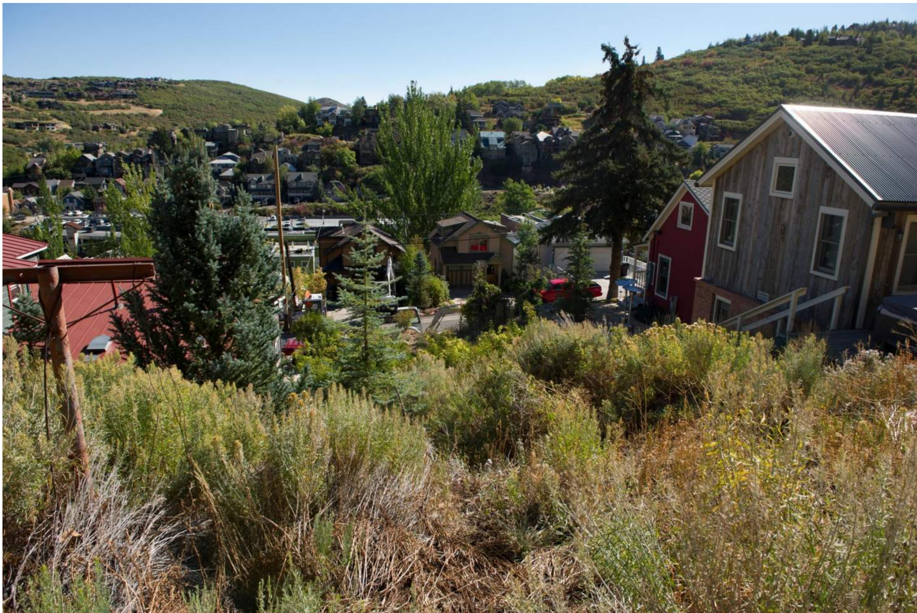
341 Woodside Avenue - looking easterly
