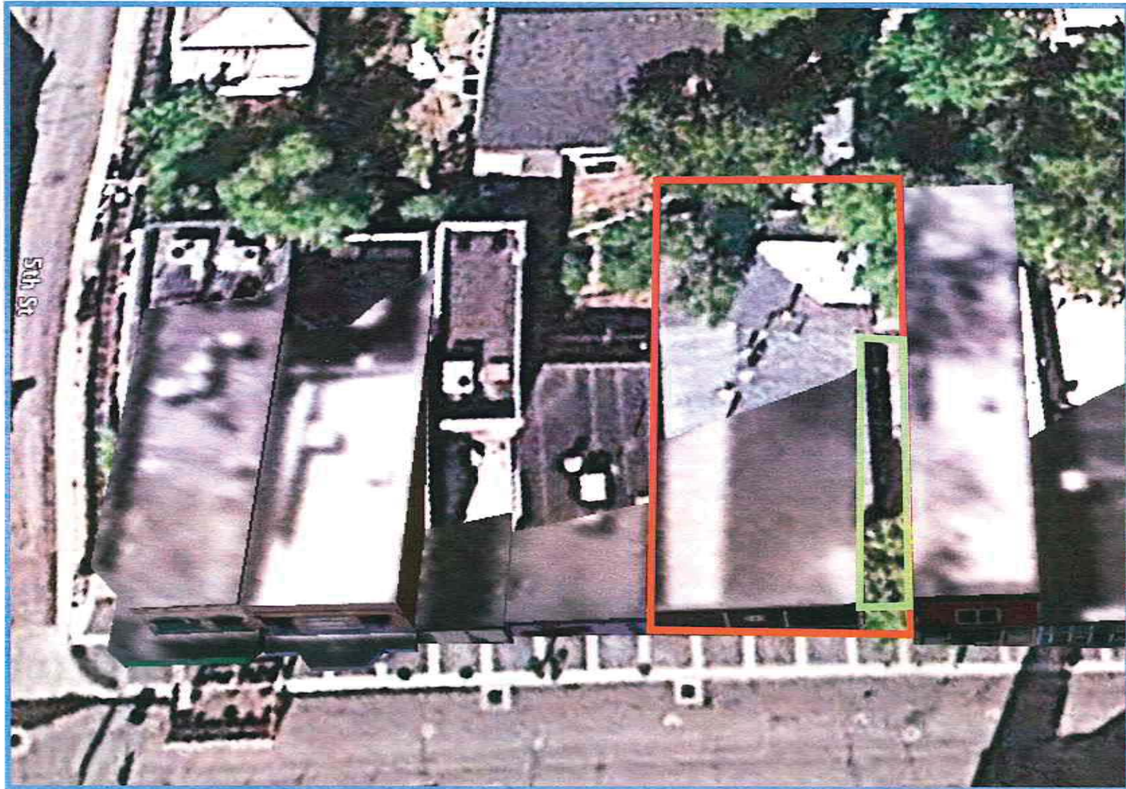
515 Main Street Property Courtyard
