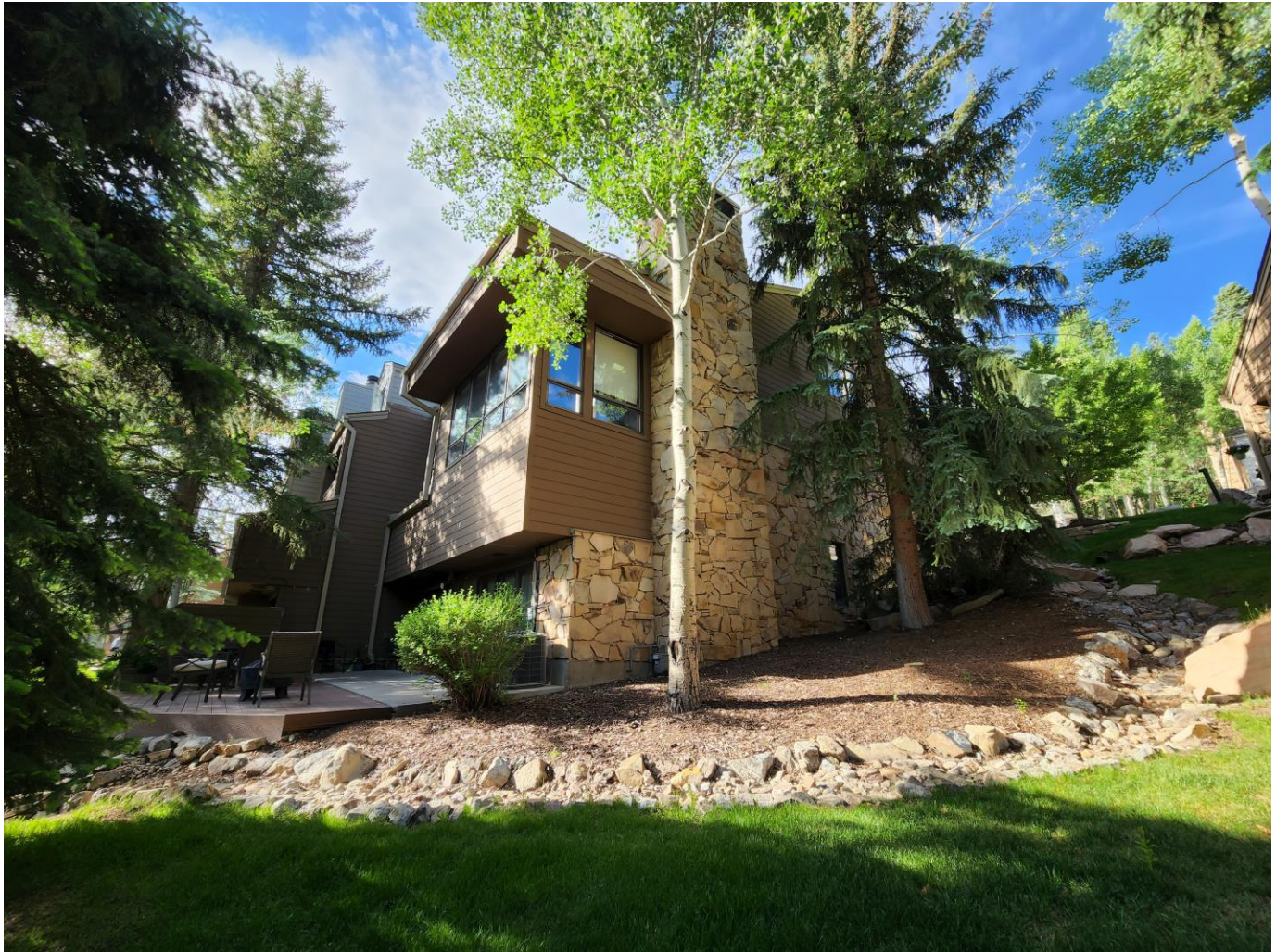
Unit 14F from the Northeast Corner of Unit 13F Looking Southeast
