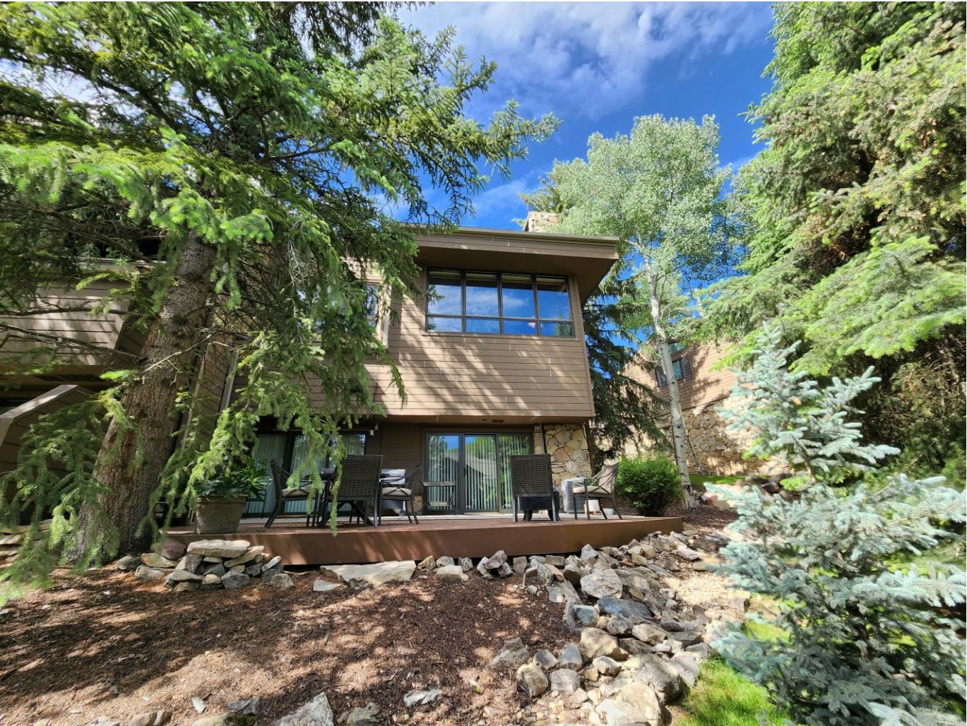
Unit 14F from the north Looking Southerly
