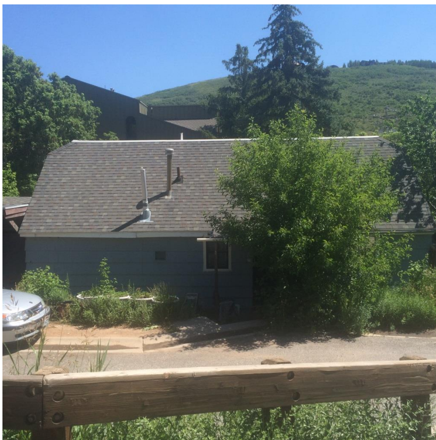
1302 Norfolk Avenue. West Elevation. June 2016.
