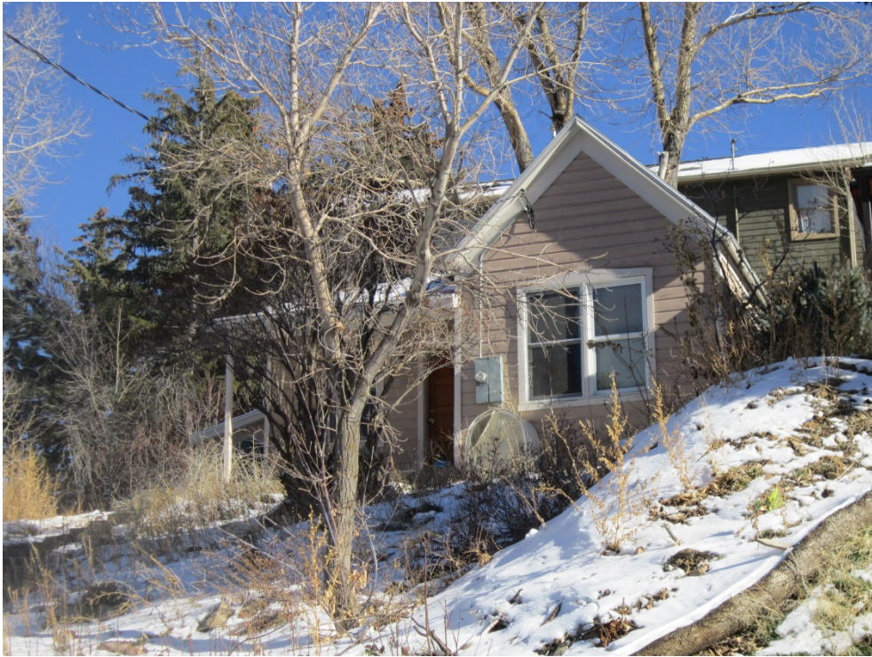
316 Ontario Avenue. Southwest oblique. November 2013.
