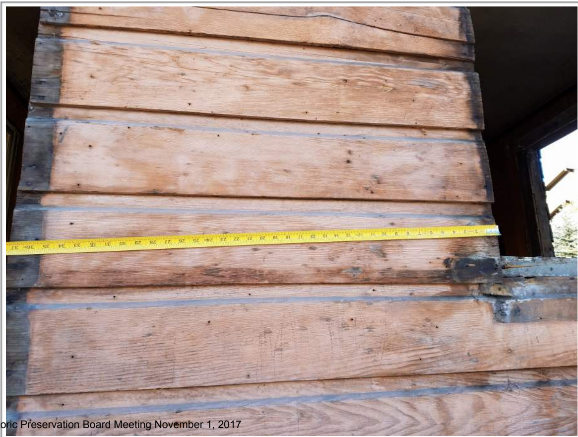
Photo #18: Typical Measurement to Determine Front Window Location
