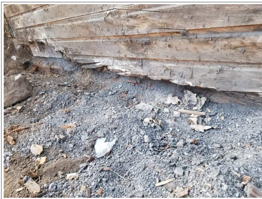
Photo #13: Deteriorated Foundation and Ash Mixture
