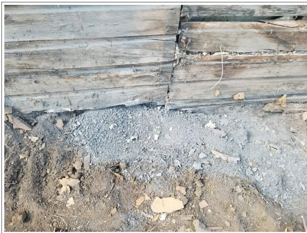
Photo #13: Deteriorated Foundation and Ash Mixture
