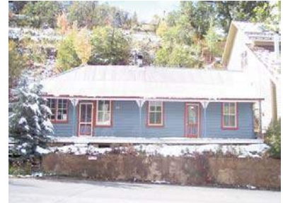
118 DALY AVENUE (pre-partial Reconstruction) Significant Site
