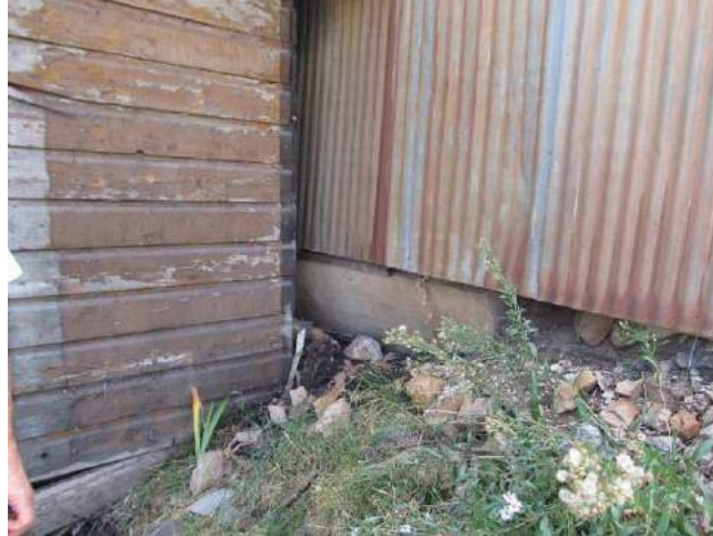
The wall on the left is the original wall between the house and sleeping porch. Note how the garage is pulling away from the wall of the house.
