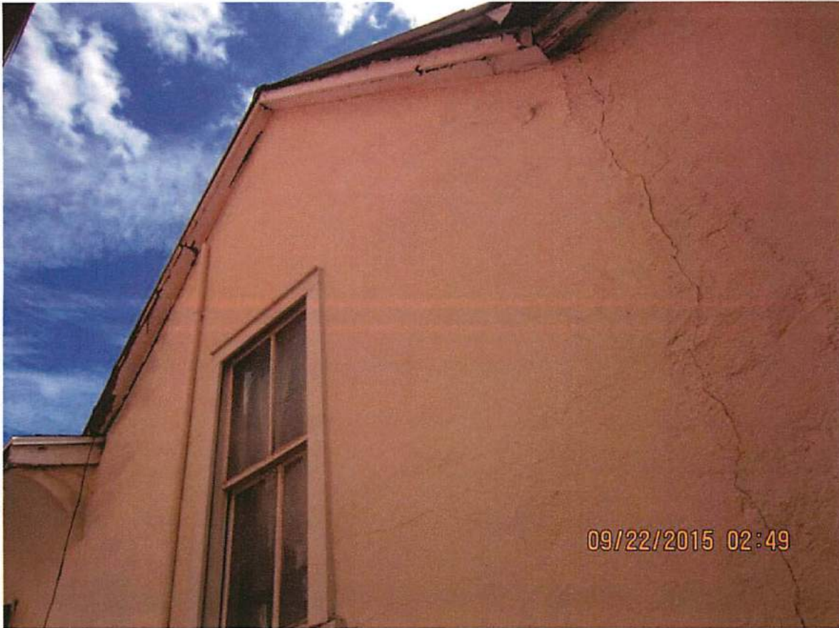
Photo 34 The "above and "below" photos represent the continuation of a structural crack that is consistent with a rubble and dirt foundation. Structural deviations are difficult to see on wood framed construction. At least 30 of the building is wood framed
