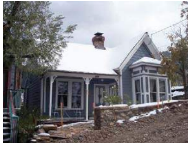
59 PROSPECT STREET Landmark Site
