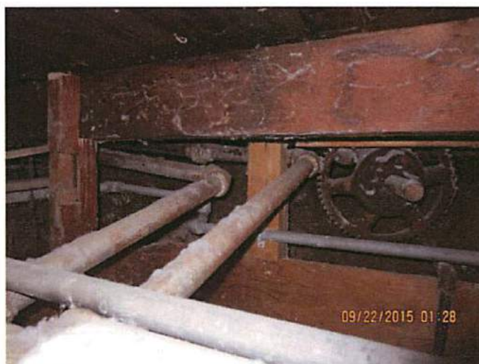
Photo 4 Unsecured gas lines, unknown valves that are not properly maintained or marked
