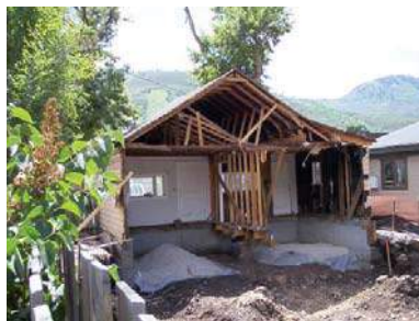
1326 PARK AVENUE (rear-during construction)
