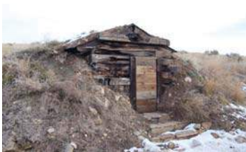
2414 MONITOR DRIVE Structure
