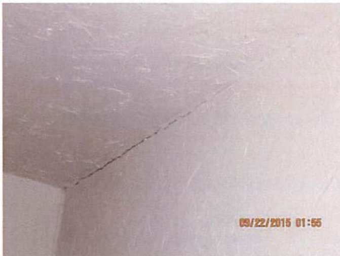
Photo 13 Structural separation in second floor bedroom. Consistent with missing point loads and missing foundation
