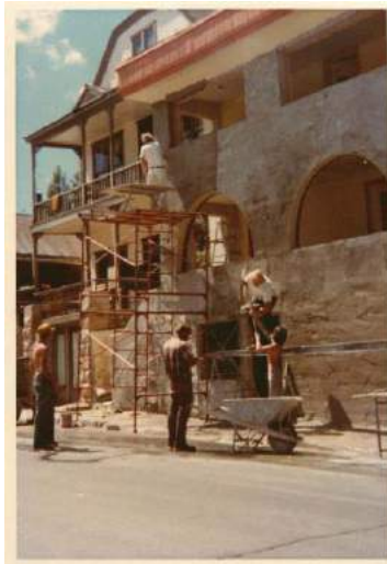
c.1976 photo of Rixies remodeling the front of the building.
