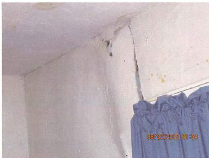
Photo 24 Decay and deterioration noted throughout the building, cause appears to be lack of proper maintenance and infiltration of water from damaged roof
