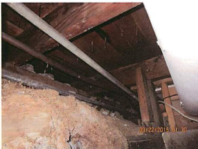
Photo 3 There are numerous pipes consisting of potable water, heating water lines and gas lines that are in direct contact with soils and not properly secured. Decay and deterioration of piping is noted throughout the underground area
