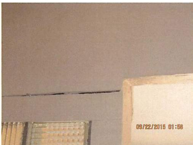
Photo 15 Structural separation in second floor bedroom. Consistent with missing point loads and missing foundation
