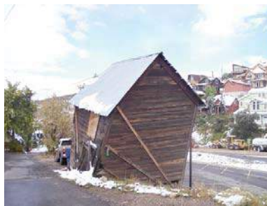
156 SANDRIDGE AVENUE Accessory Building
