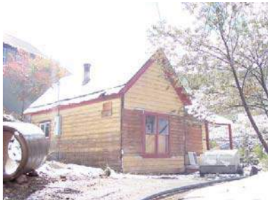
68 PROSPECT STREET Landmark Site
