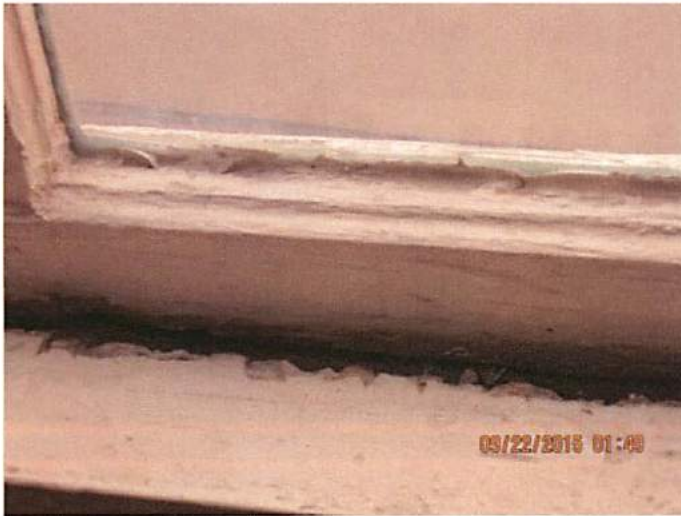
Photo 17 Several windows on the second floor have separated and have been nailed shut. This is consistent with wracked and warped walls due to structural stability of the building
