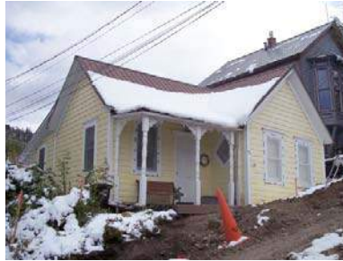
51 PROSPECT STREET Landmark Site
