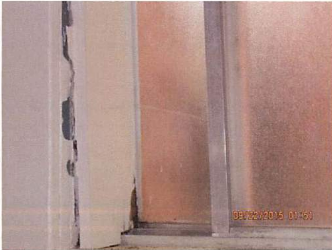
Photo 11 Noted settling around the bathroom window on the second floor. Consistent with improperly installed support beam on third floor.
