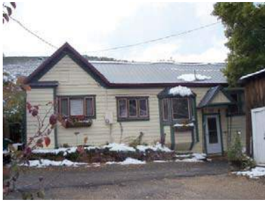
130 SANDRIDGE AVENUE Landmark Site
