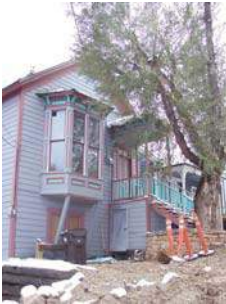
57 PROSPECT STREET Landmark Site
