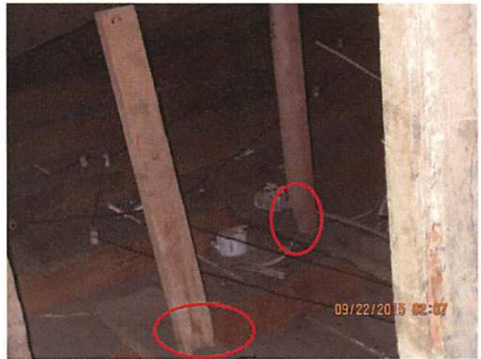
Photo 6 Support members not fastened and are not perpendicular to the load they serve
