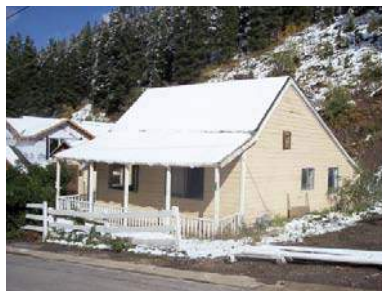
309 DALY AVENUE Significant Site
