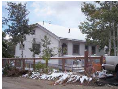
101 PROSPECT STREET Landmark Site
