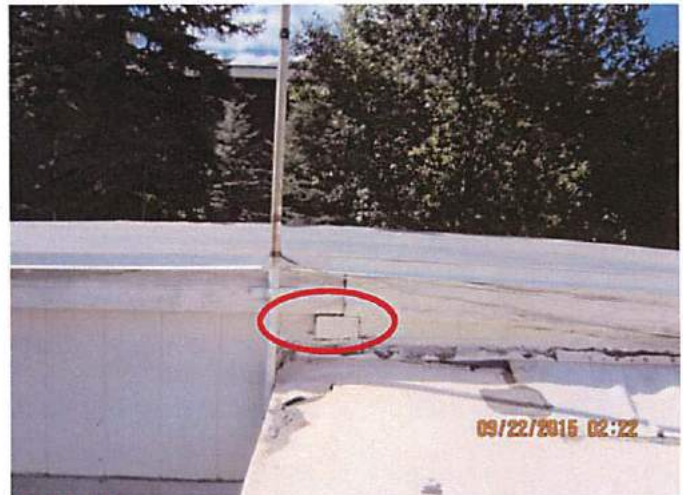
Photo 8 Note structural beam. Refer to photo 9
