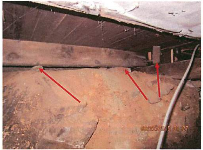
Photo 24 The addition of bracing and shims to prevent settling of the building. Cannot have bearing directly on soils. All bearing is directly on soils. Engineer to justify
