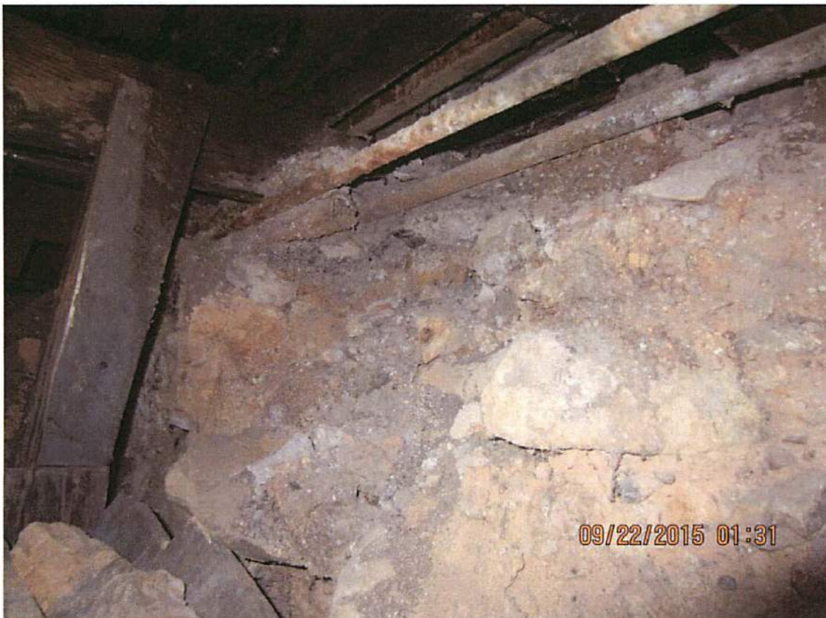
Photo 34 The "above and "below" photos represent the continuation of a structural crack that is consistent with a rubble and dirt foundation. Structural deviations are difficult to see on wood framed construction. At least 30 of the building is wood framed
