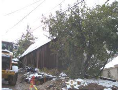
9 HILLSIDE AVENUE (pre-reconstruction)
