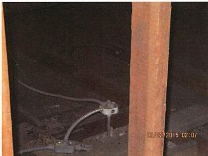
Photo 20 Open electrical boxes noted throughout the building. Electrocutation hazard, fire hazard. Located in attic
