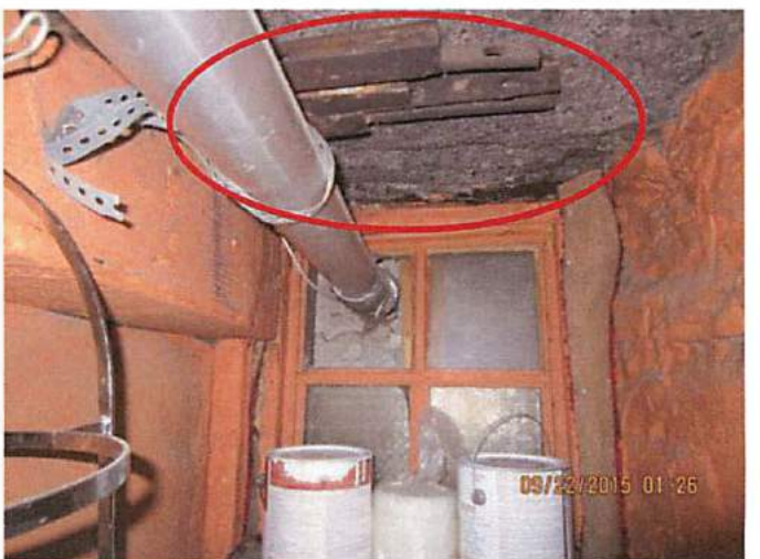
Photo 28 Rail road rails being used as shims for floor above. This area would be Approximately 18 feet into front entry main level.
