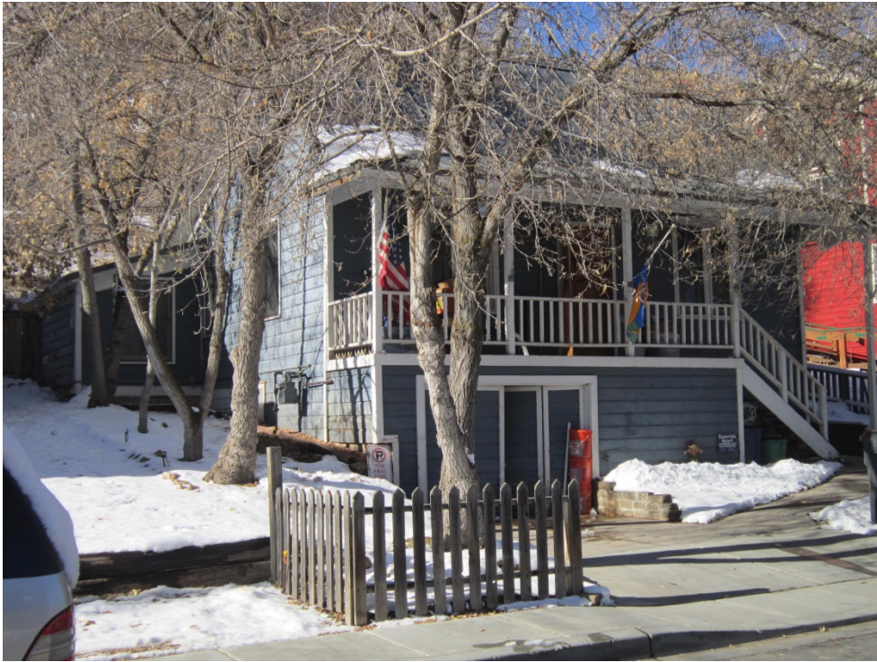
161 Park Avenue. Southeast oblique. November 2013.
