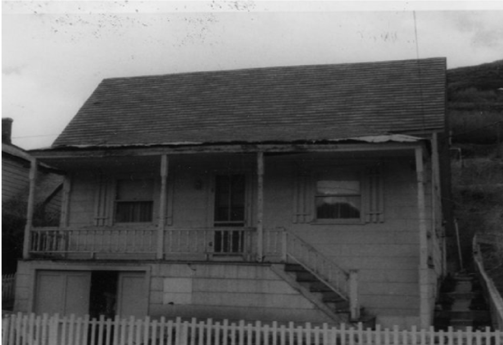
Photo # 2010.24.36 – undated photo east elevation “110 Block Park Ave “Dunsmore. Henry Knight” estimated 1945 – when Knight purchased the house from Dunsmore
