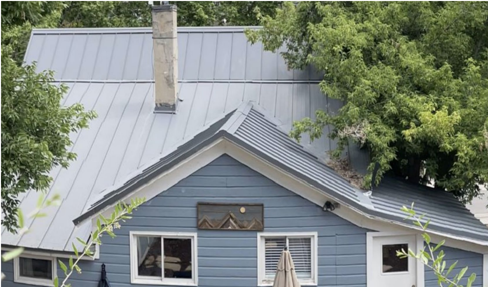
Photo 18.1 – West Elevation Roof
