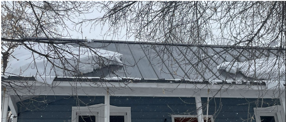
Photo 18.3 – east view roof
