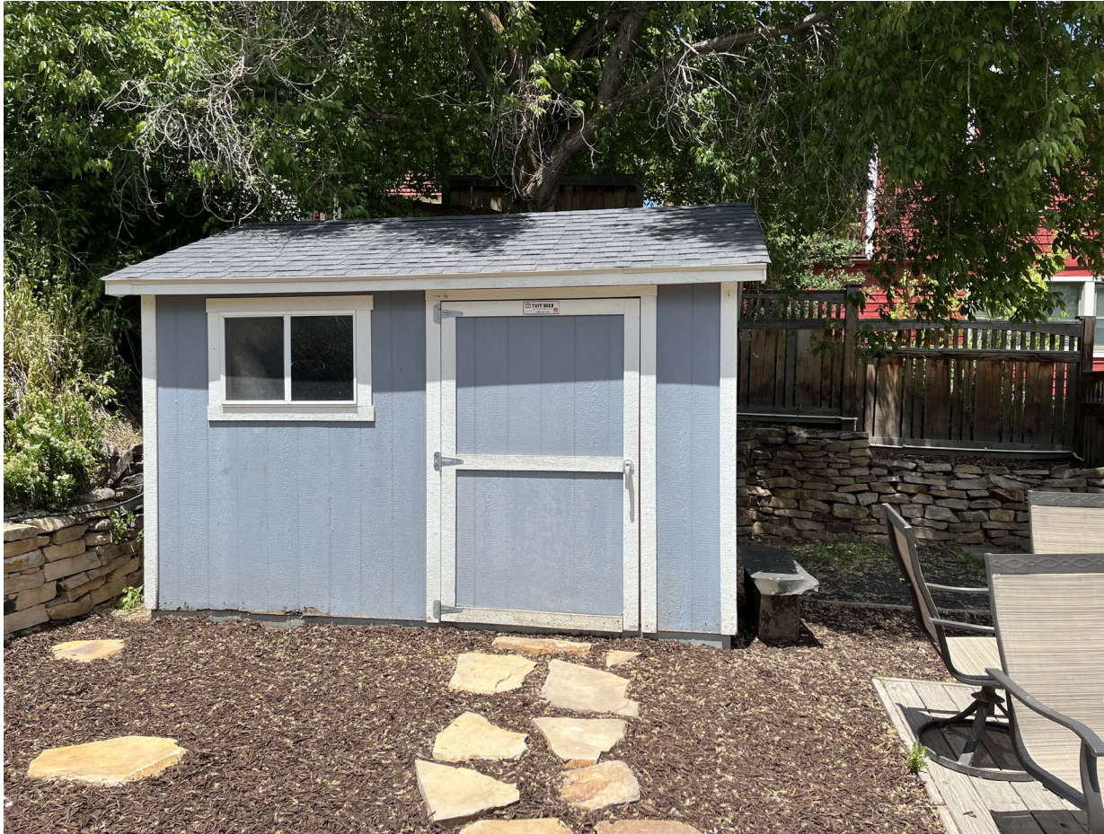
Photo #20: West Elevation – Accessory Building
