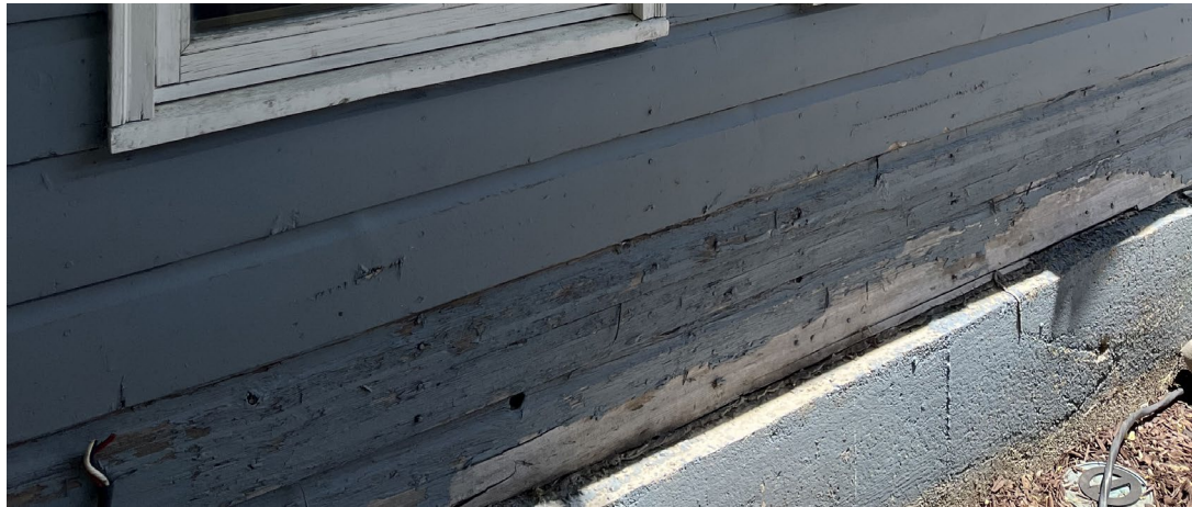
Photo 18.2 – Foundation rear corner
