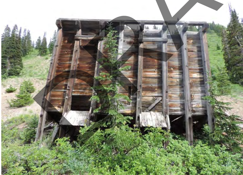
Jupiter Mine Ore Bin. From northwest. July 2016.
