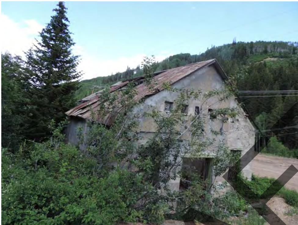
Alliance Tunnel pump house. From west. July 2016.
