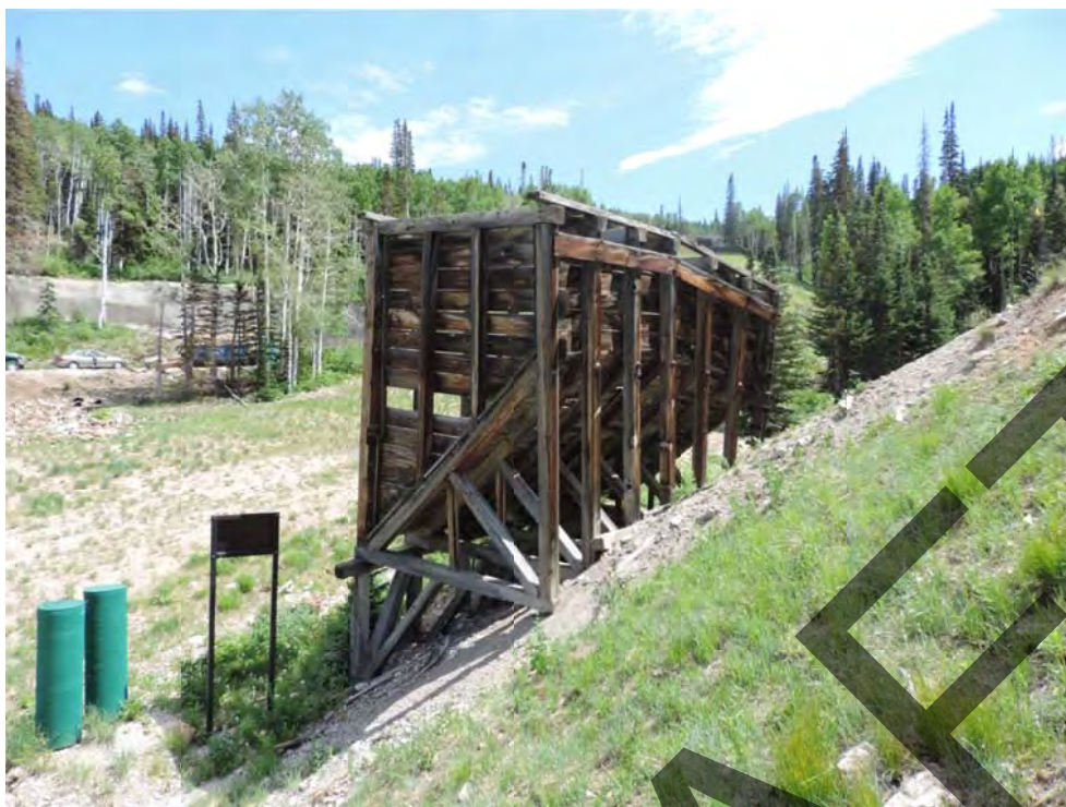
Little Bell Ore Bin. From northwest. June 2016.
