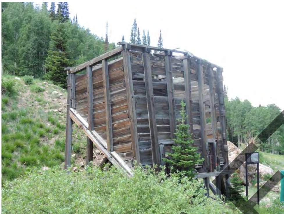
Little Bell Ore Bin. From southeast. June 2016.
