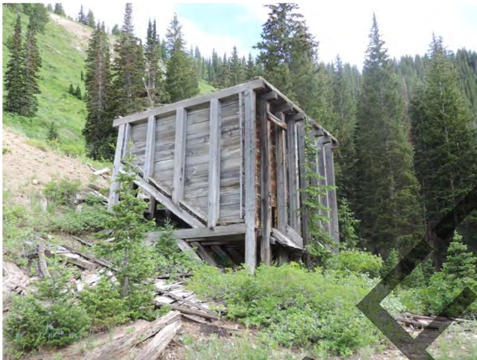
Jupiter Mine Ore Bin. From north. July 2016.
