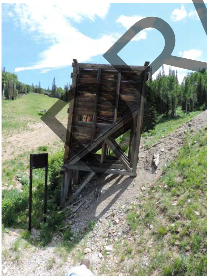
Little Bell Ore Bin. From north. June 2016.
