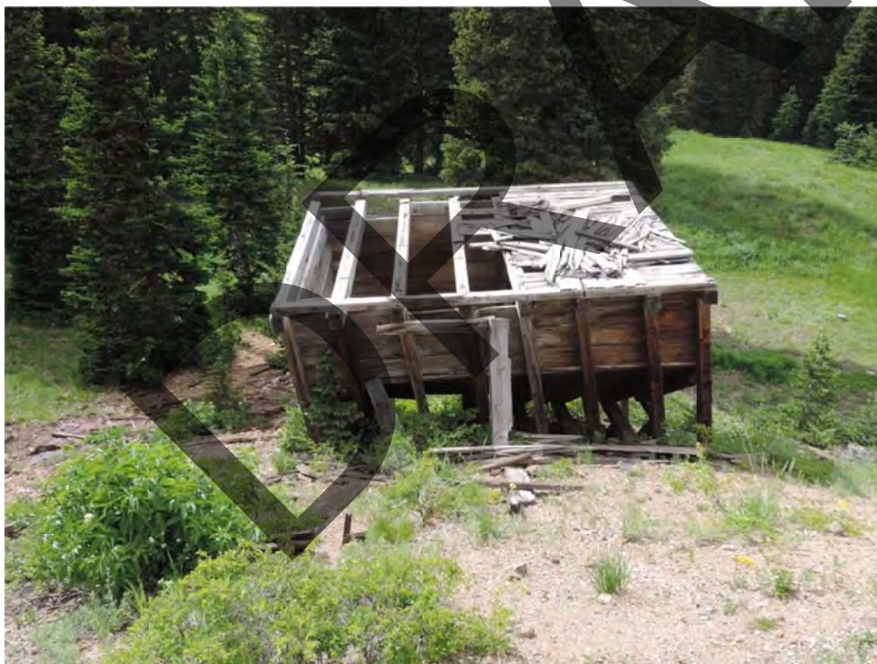
Jupiter Mine Ore Bin. From southeast. July 2016.
