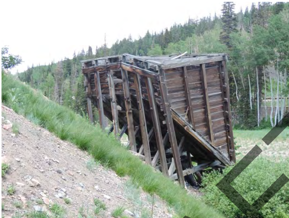
Little Bell Ore Bin. From southwest. June 2016.
