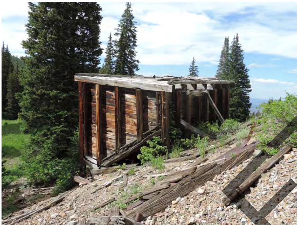
Jupiter Mine Ore Bin. From south. July 2016.
