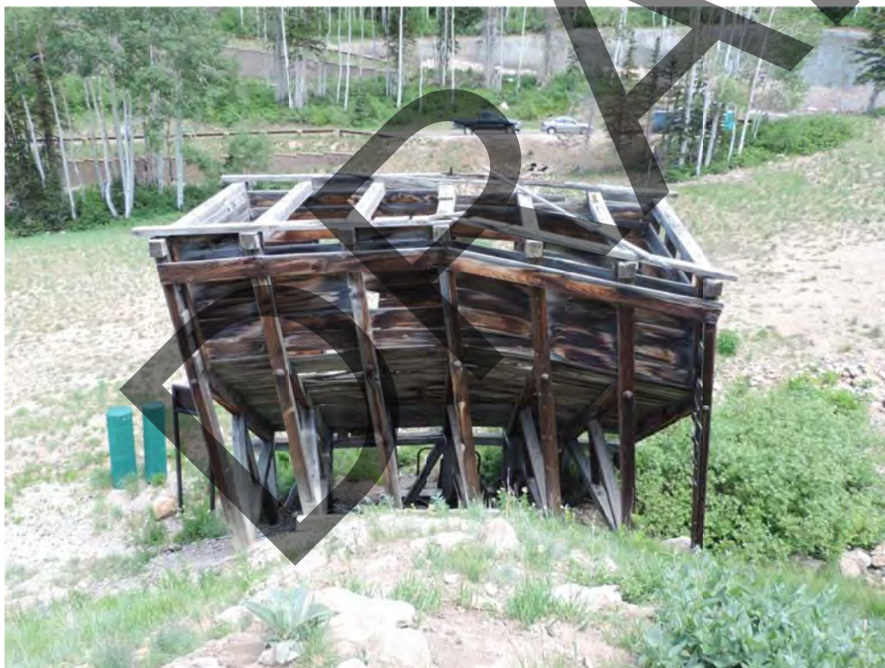
Little Bell Ore Bin. From west. June 2016.
