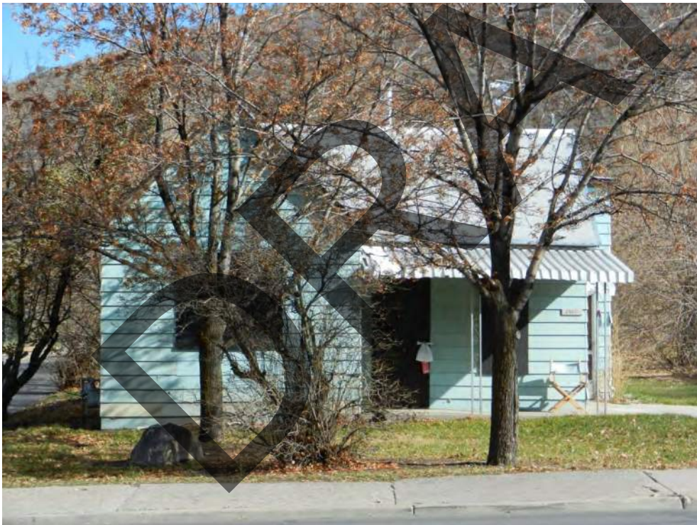
1460 Park Avenue. West elevation. November 2013.
