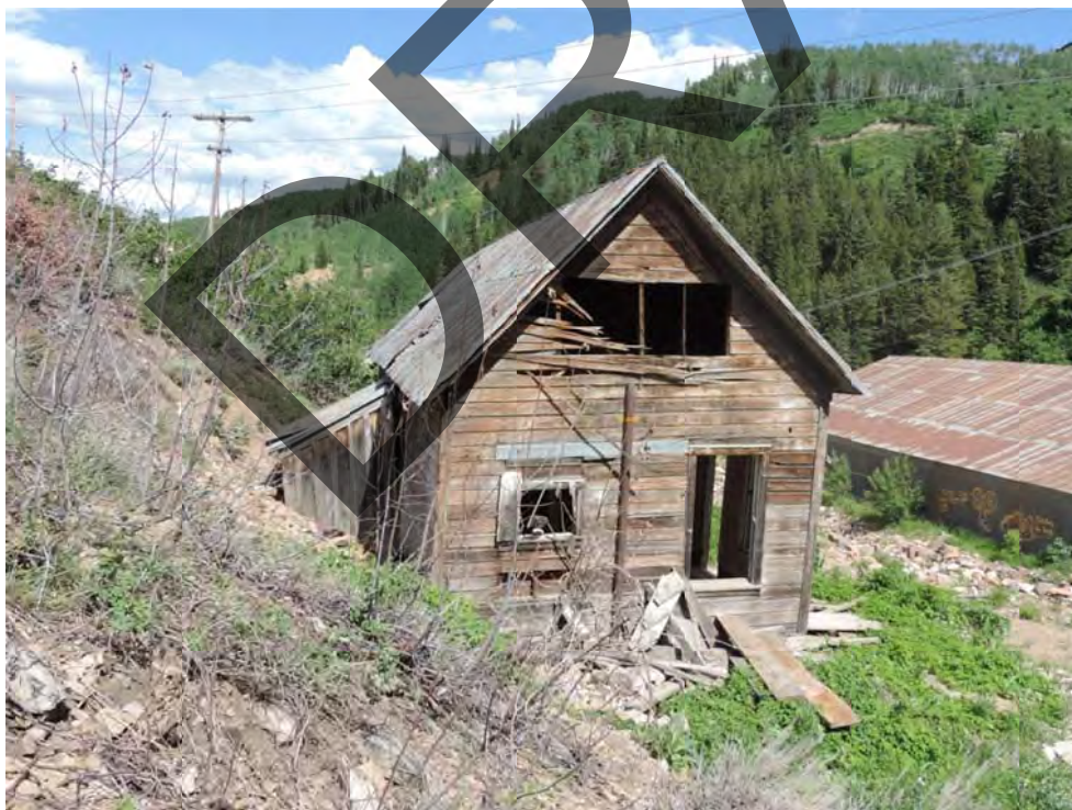
Alliance Tunnel office-dwelling. From northwest. July 2016.
