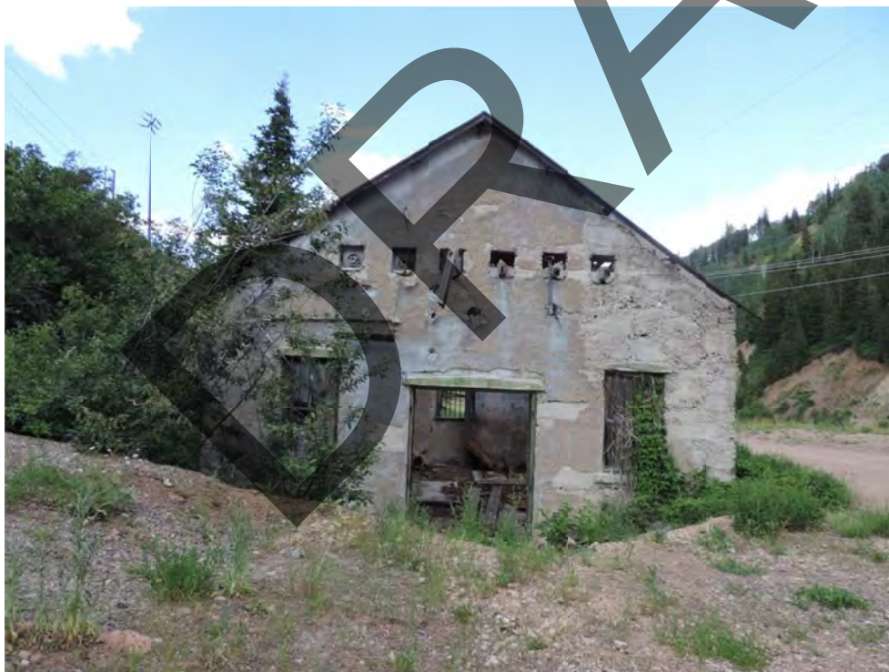
Alliance Tunnel pump house. From southwest. July 2016.
