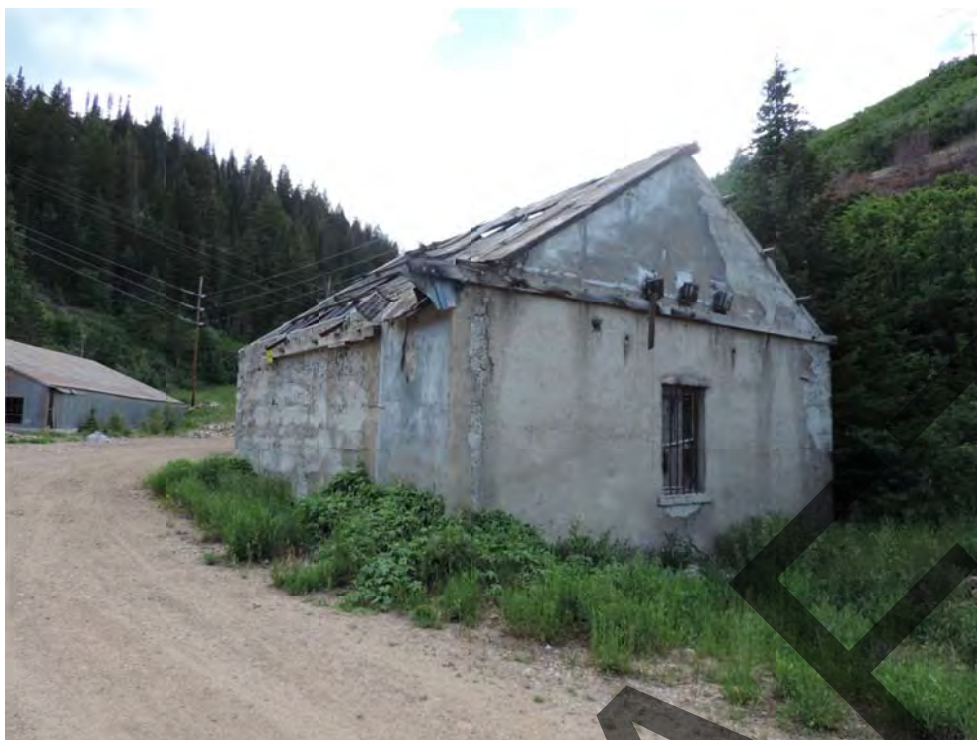
Alliance Tunnel pump house. From east. July 2016.
