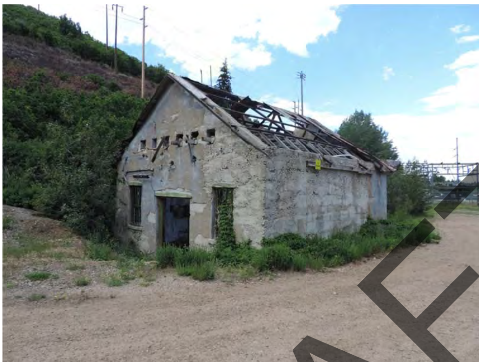
Alliance Tunnel pump house. From south. July 2016.
