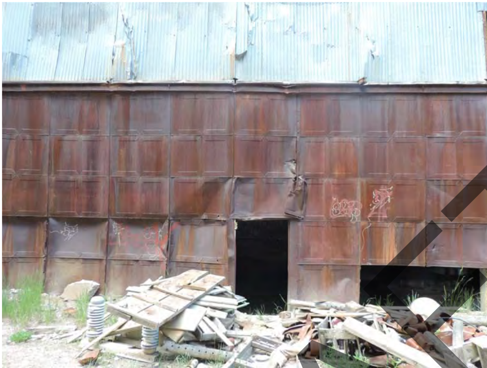
Alliance Tunnel change room. From south. July 2016.
