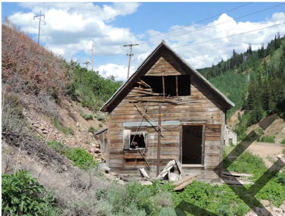
Alliance Tunnel office-dwelling. From west. July 2016.
