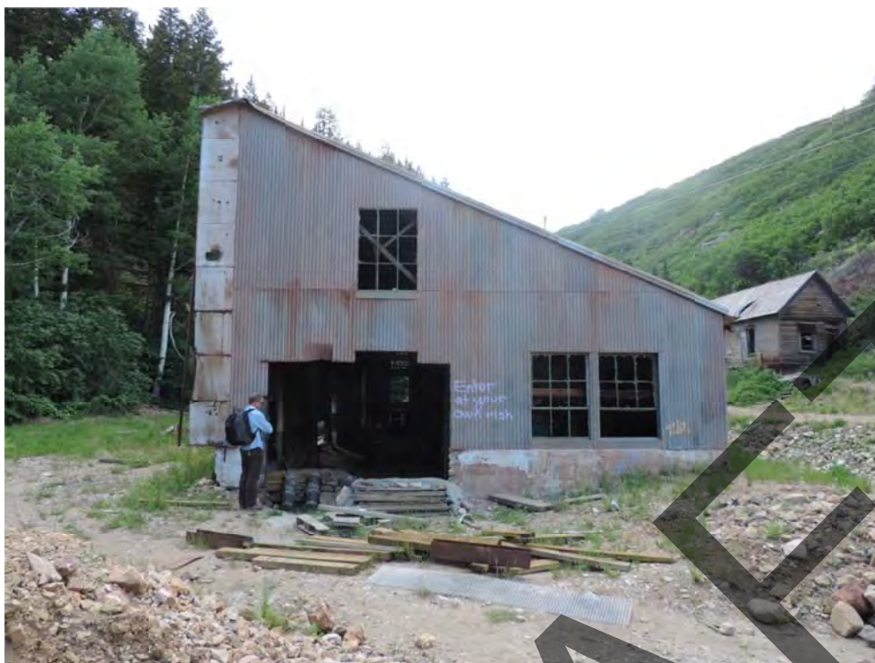
Alliance Tunnel change room. From east. July 2016.
