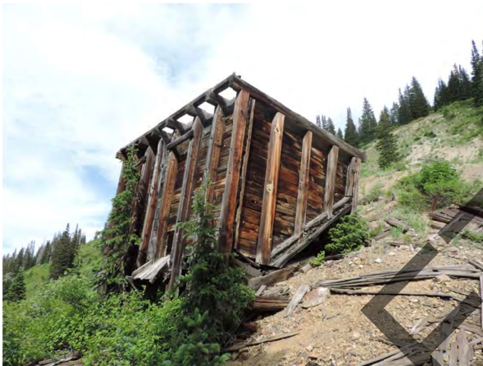
Jupiter Mine Ore Bin. From west. July 2016.
