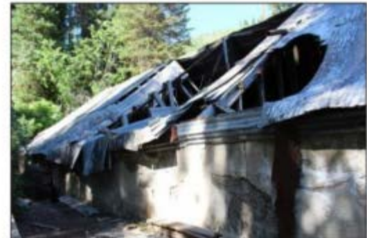
Figure 9. Southeast side of Judge Mining and Smelting Company Office, facing west. Note collapsed roof and spalling concrete of wall.
