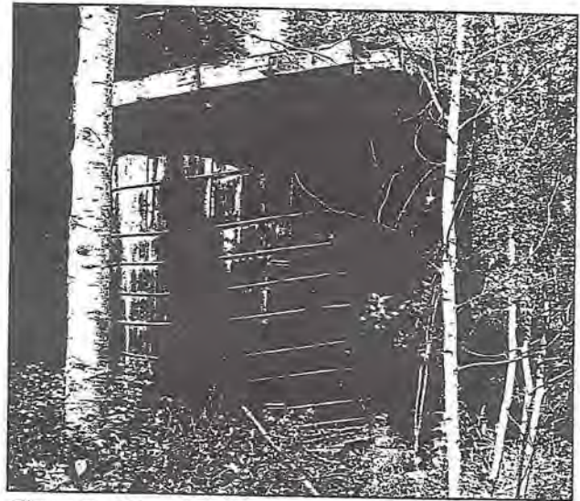
Figure 8 – Water Tank E.
