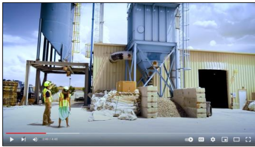
Video: Glass Recycling Facility Link: https://youtu.be/gWxyxYXlv9A
