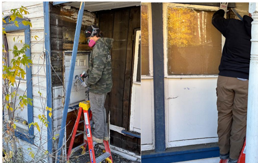
Image 1: Onsite deconstruction, images taken by Stantec while on site.
