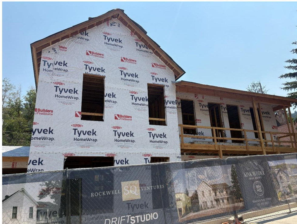
Image 2: Framed Structure, image taken in August of 2026.
