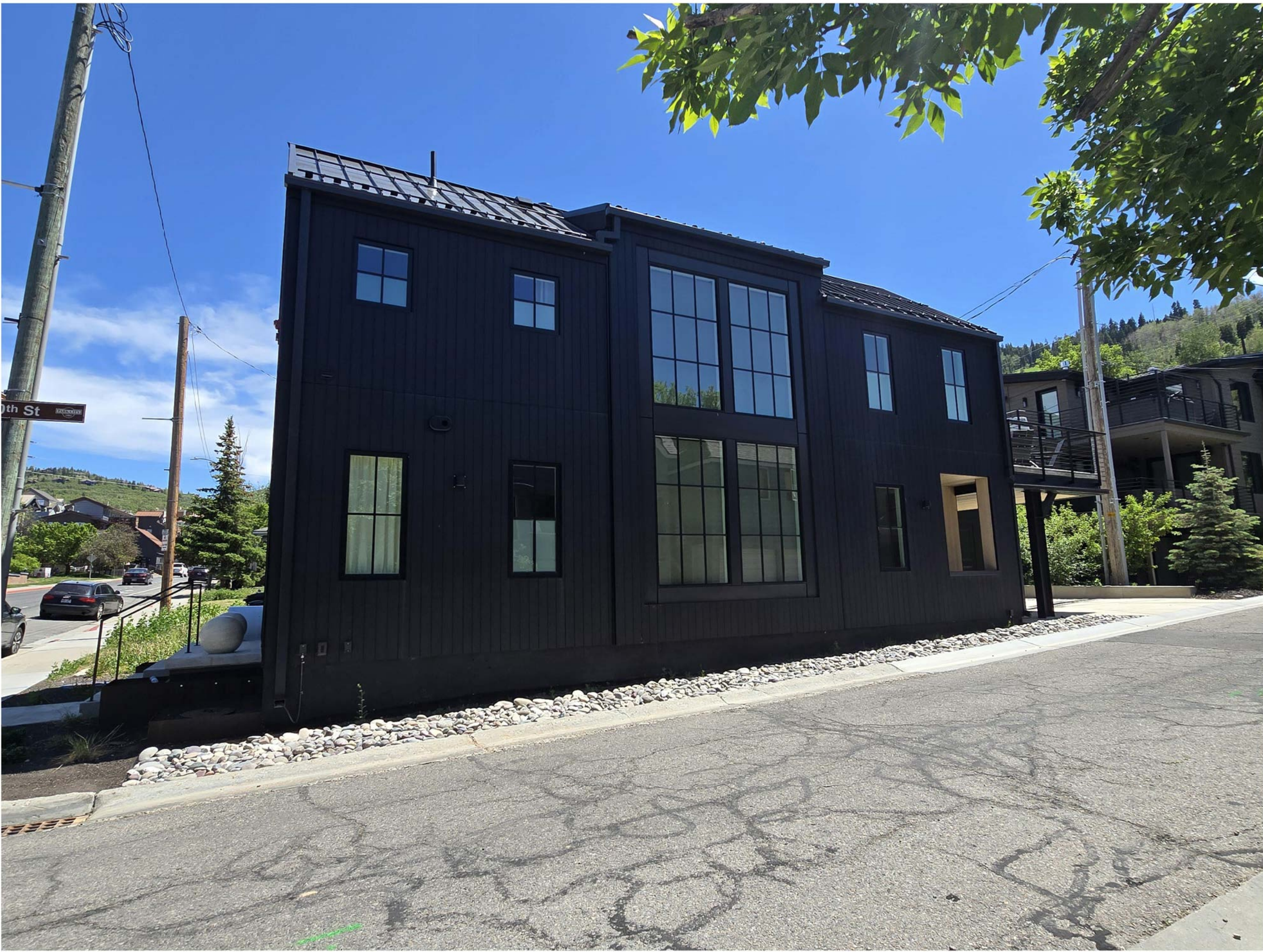
961 Park Ave - 10th Street Facade
