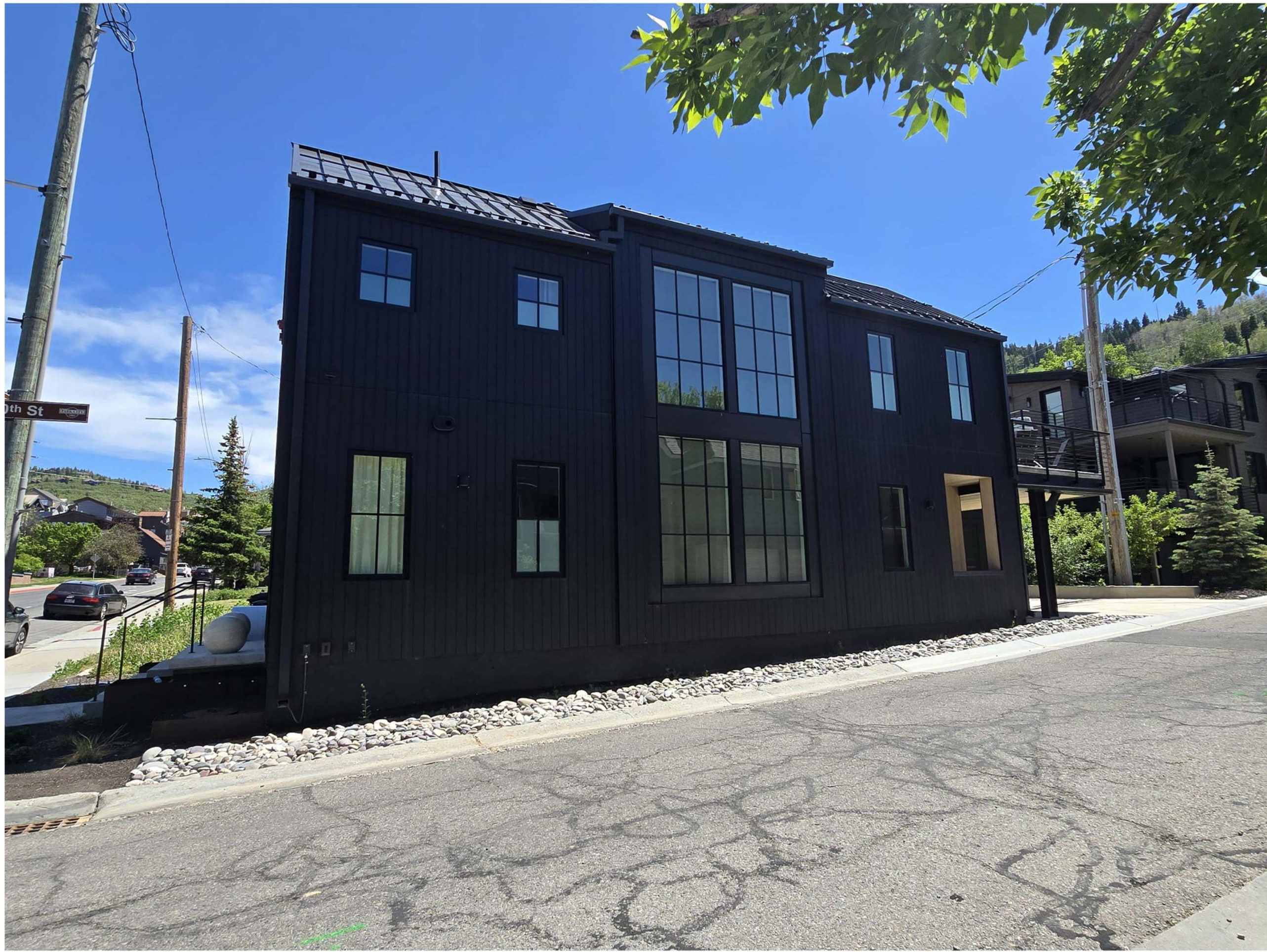
961 Park Ave - 10th Street Facade
