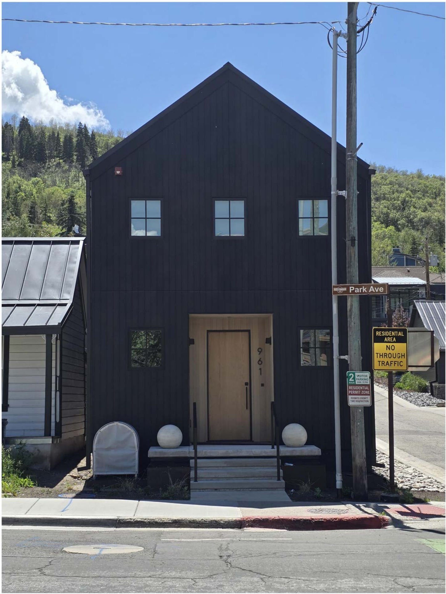
961 Park Ave - Park Ave Facade
