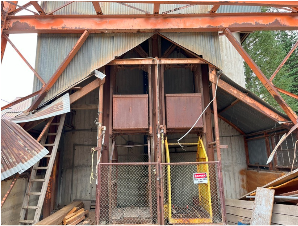
Figure 4: Thaynes Hoist House Mine shaft and cages pictured in 2025
