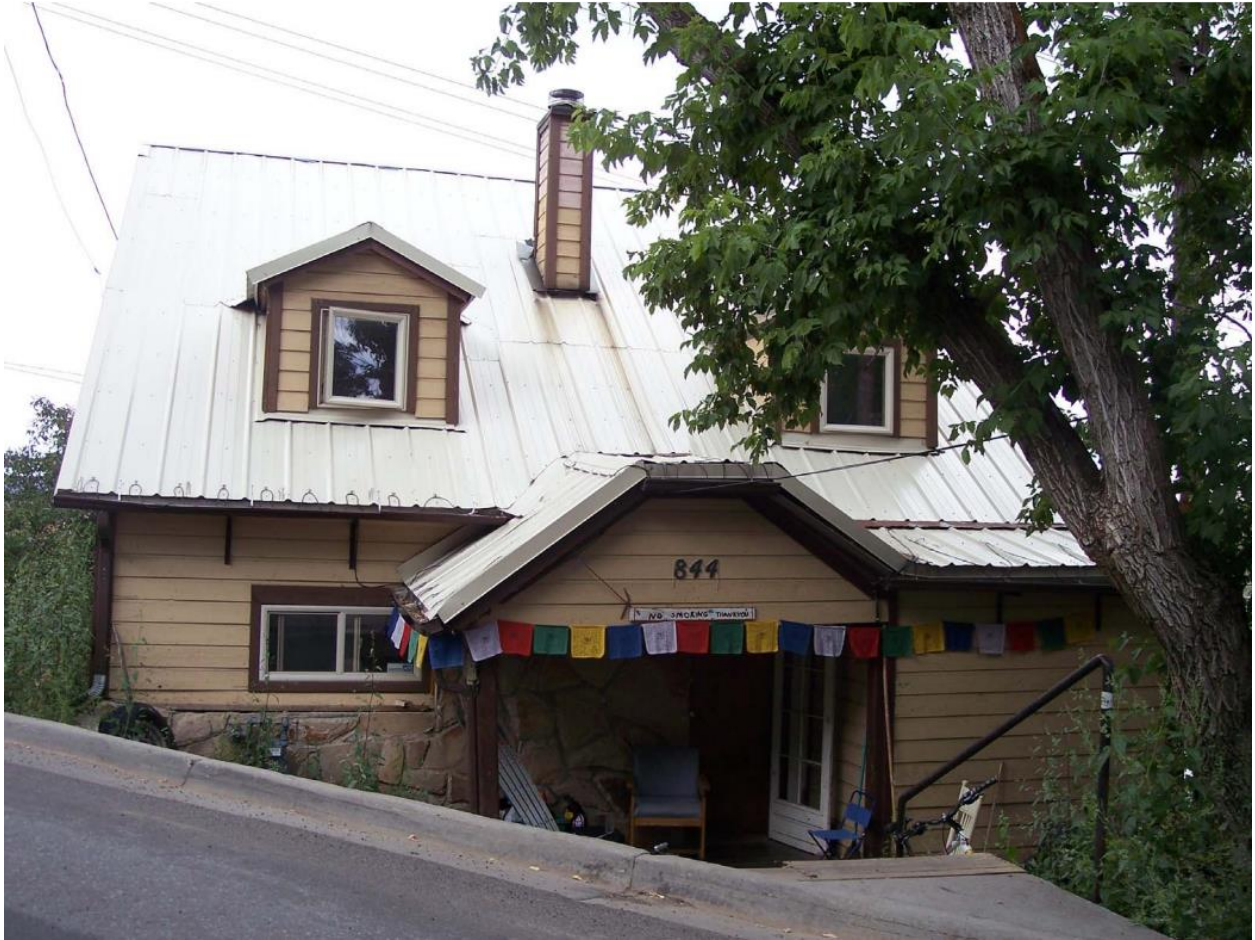
Figure 4: Current conditions view of rear (south) façade of 844 Empire Avenue, looking north from Crescent Tram Road.
