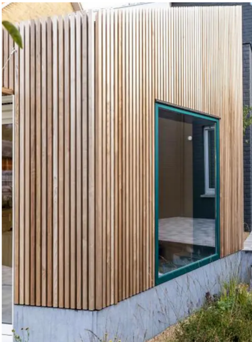
Figure 2: Rainscreen cladding with narrow vertical slats
