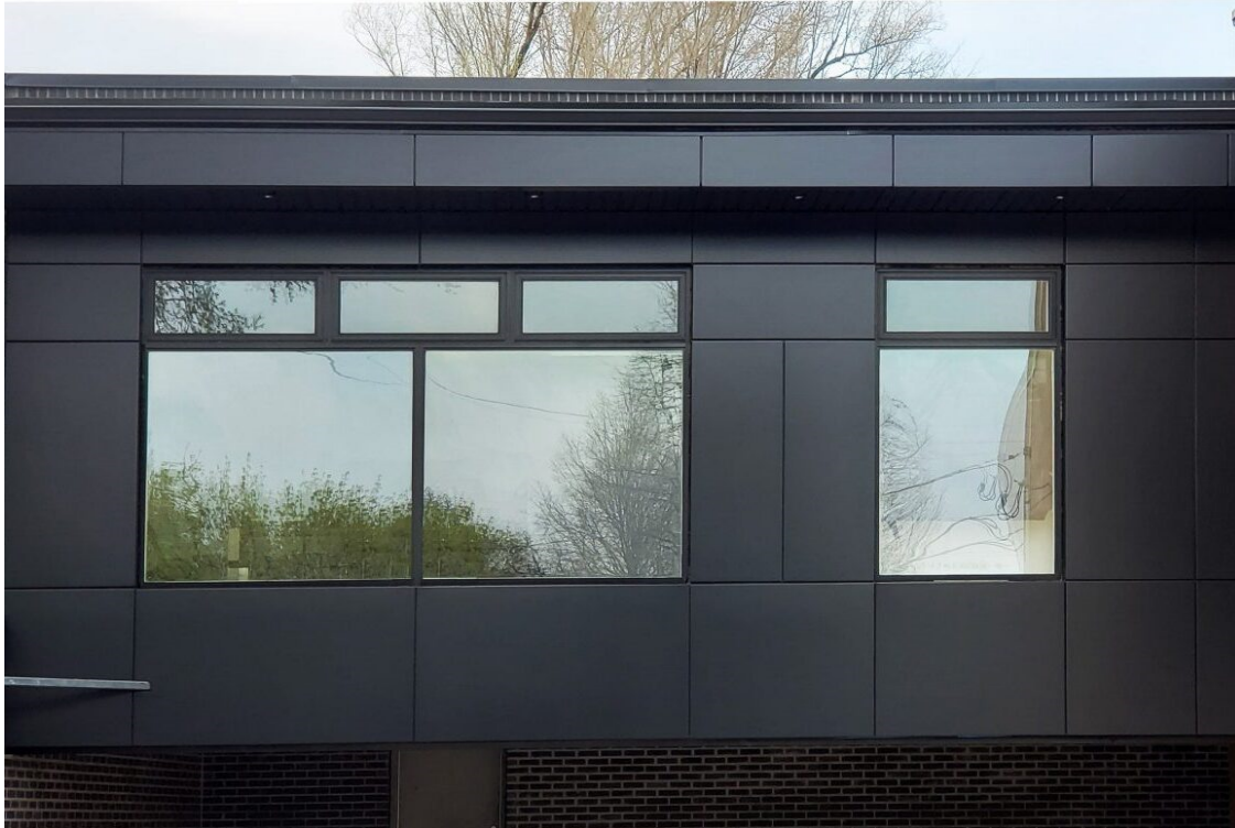
Figure 3: Example of Aluminum Composite Panels (ACM) in various dimensions
