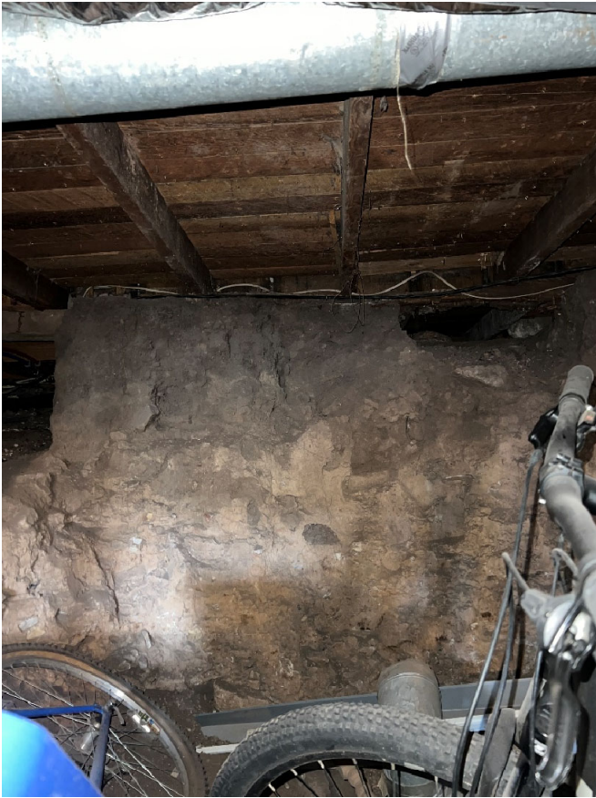
Crawl space photos, via JSARC Architects
