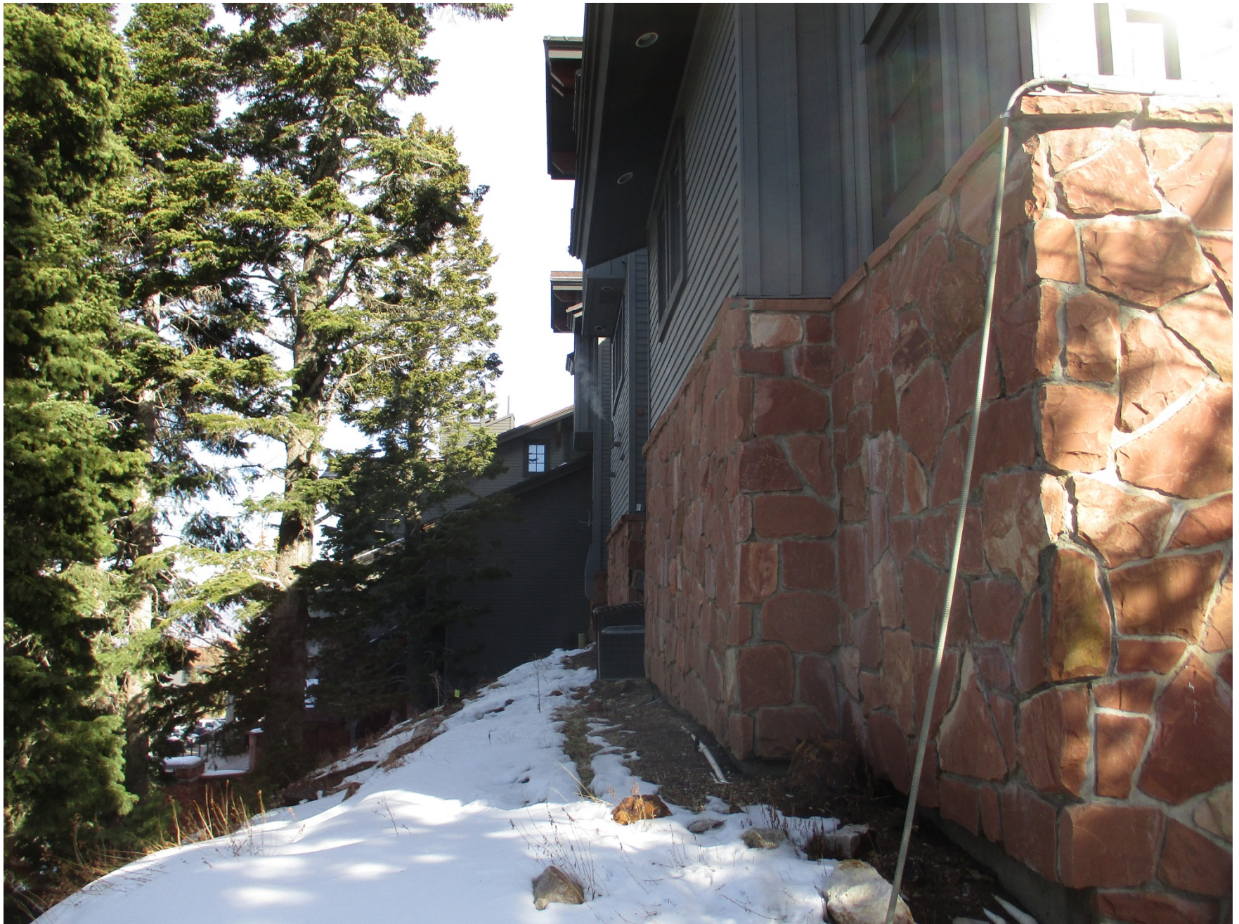
Stag Lodge Unit 41 – looking northeasterly
