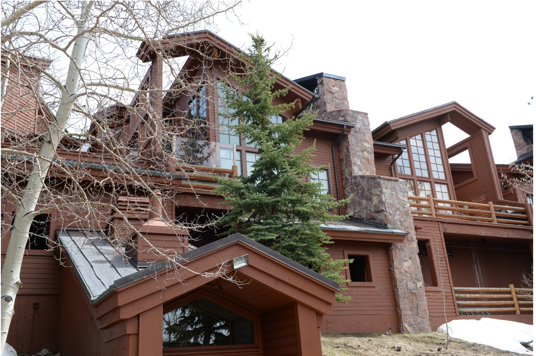
Stag Lodge Unit 10 – looking northwesterly
