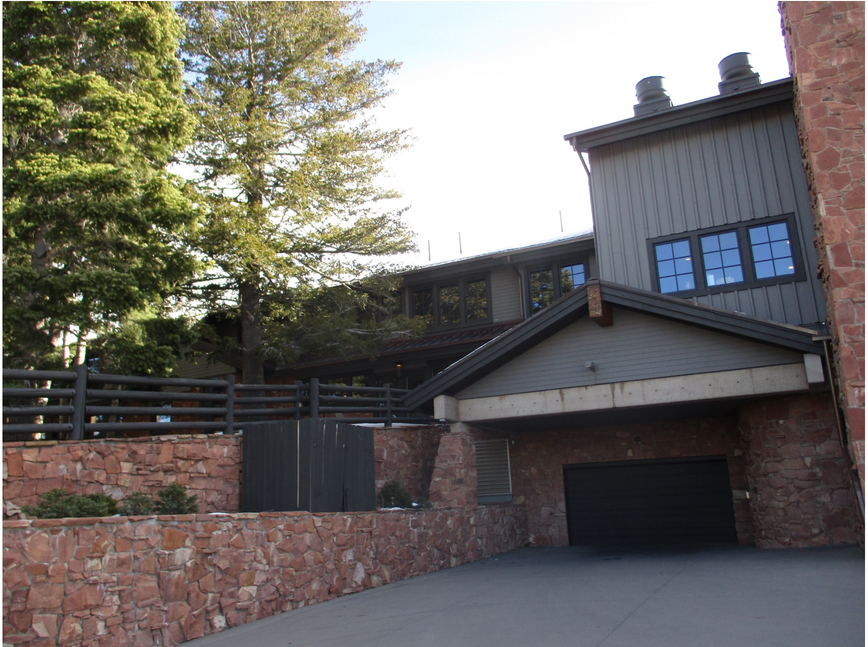
Stag Lodge Unit 10 - looking northeasterly
