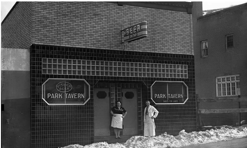
Figure 2: During the 1940s and 1950s, Mike Safianides ran the Park Tavern out of 322 Main Street. The signs were converted to windows, and the building was clad in masonry veneer and tile. Source: Town Lift: Park City News, https://townlift.com/2022/06 .
