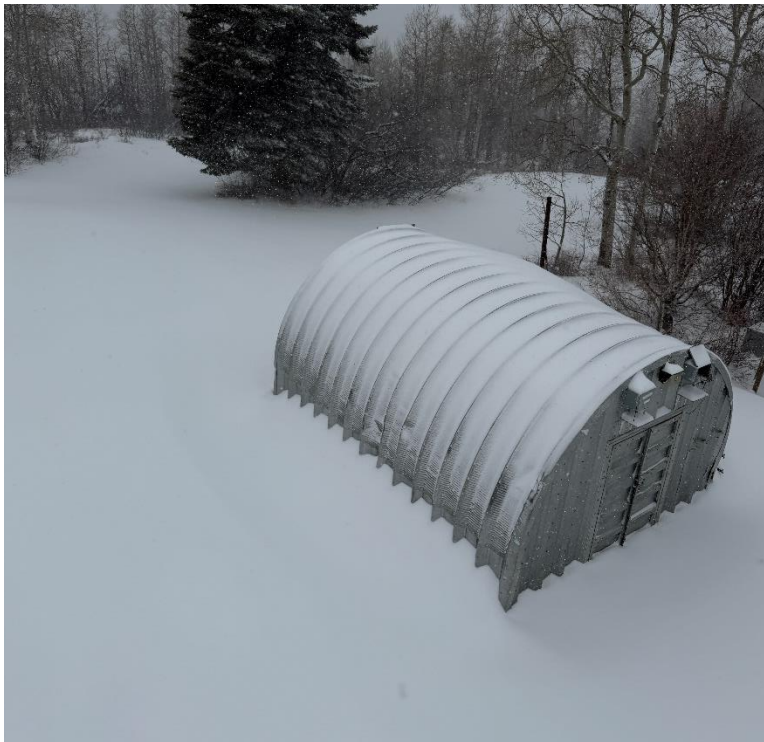
Figure 2: Existing Conditions (Winter) Photo of Sled Storage, Looking Northwest
