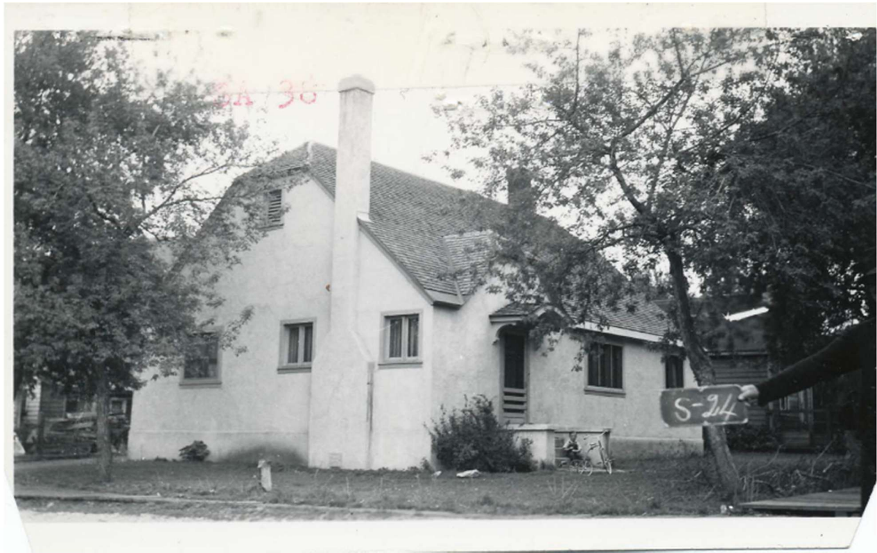
Figure 1. 1940 Tax Photo of 1066 Woodside Avenue. Vents at the upper story and lack of windows indicate that it was not a living space. Source: Park City Municipal Corporation, ILS Form.
