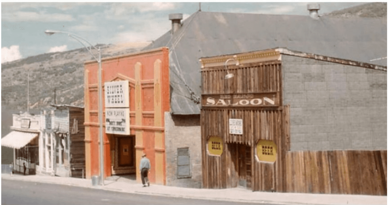
Figure 4. Colorized historic photograph of 322 Main Street. This is likely from the 1960s after the Red Banjo saloon opened. The adjacent Silver Wheel appears to have been operated at this time. Source: Town Lift: Park City News, https://townlift.com/2022/06/red-banjo-celebrates-60-years/ .
