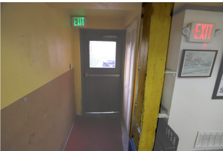
LEVEL 0 COLUMN IN REAR (EAST)
