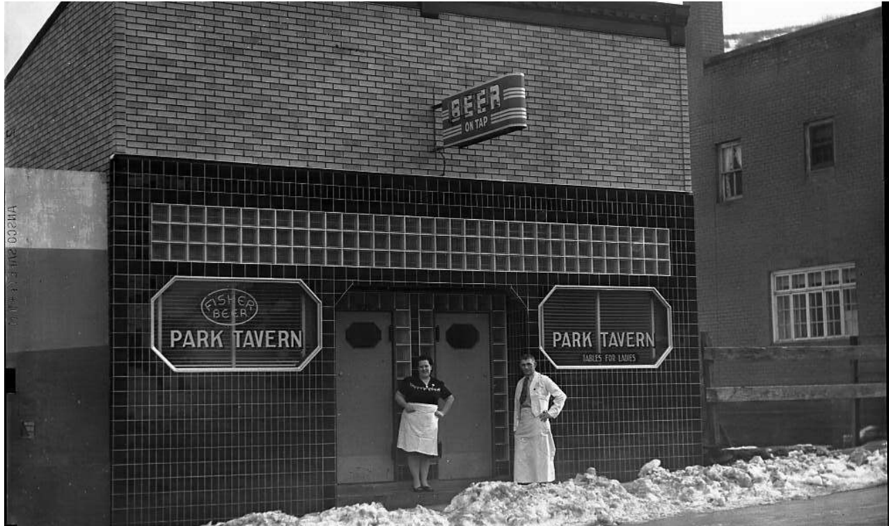
Figure 2. During the 1940s and 1950s, Mike Safianides ran the Park Tavern out of 322 Main Street. The signs were converted to windows, and the building was clad in masonry veneer and tile. Source: Town Lift: Park City News, https://townlift.com/2022/06/red-banjo-celebrates-60-years/ .
