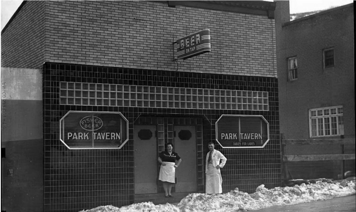
Figure 12: Structure in the 1940s and 1950s showing the storefront windows were reduced in size and the transom windows were replaced with a horizontal span of extensive glazing
