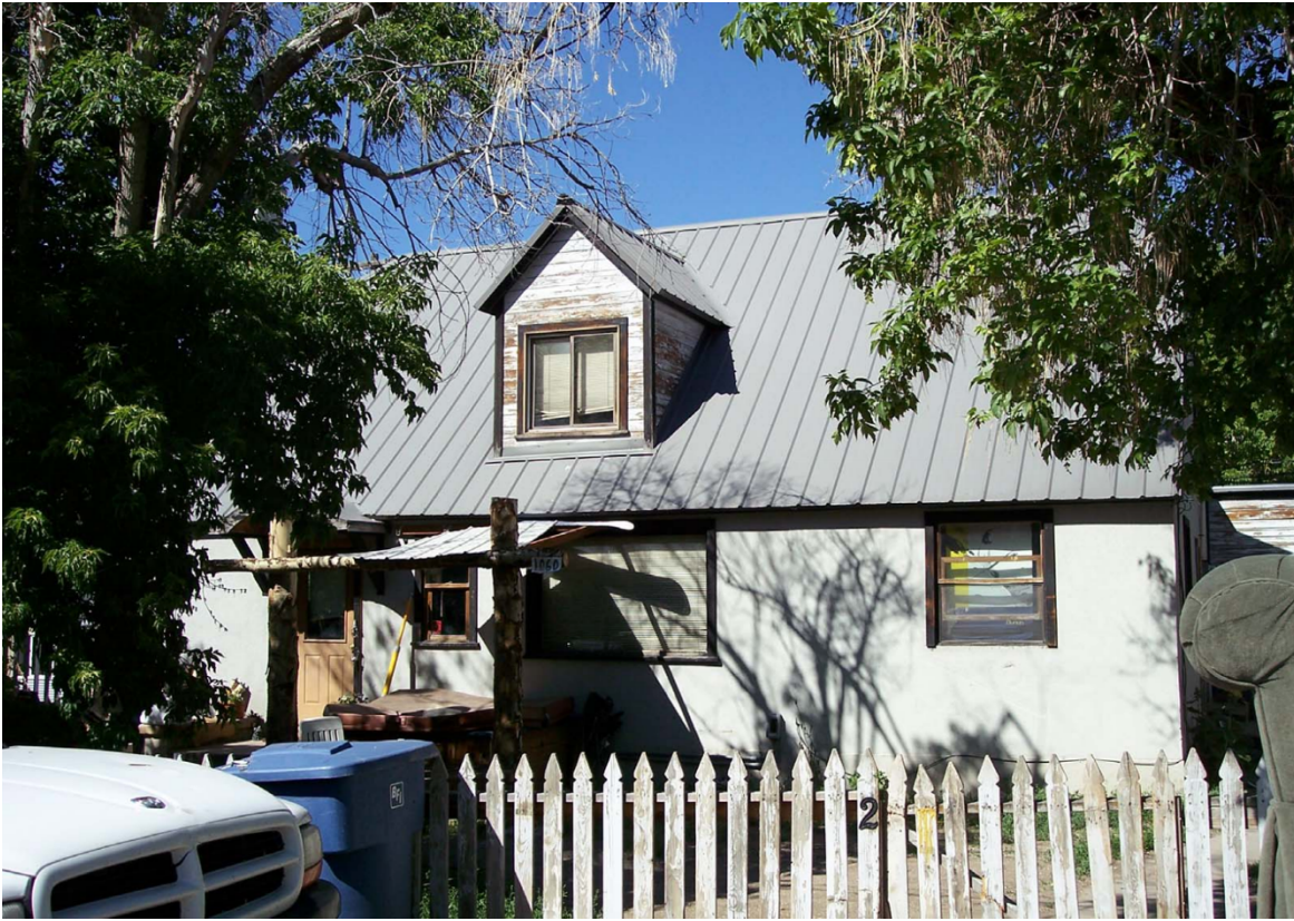
Photo 5: 1060 Woodside Avenue. West elevation. 2006
