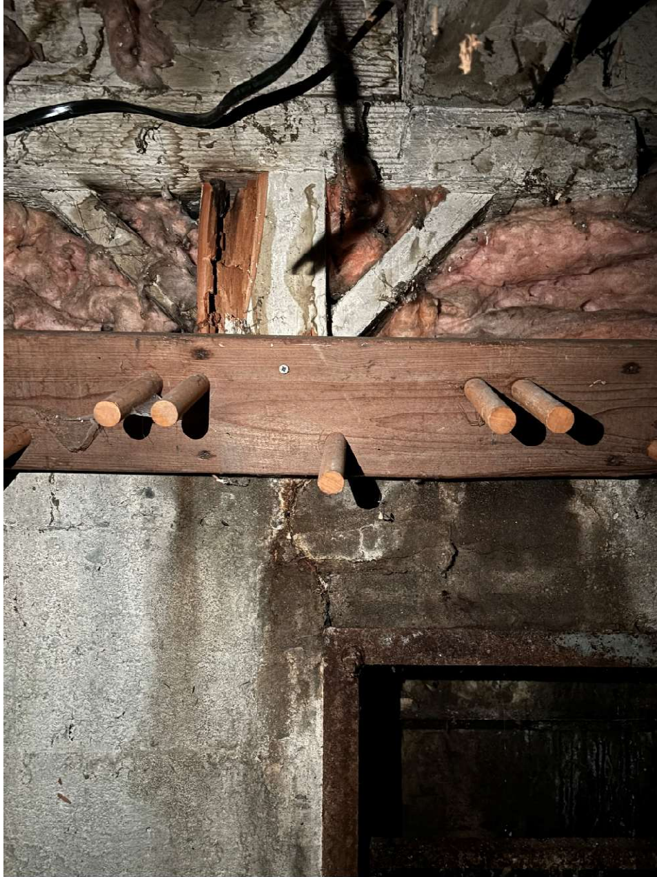
Figure 7. The floor and foundation structure is visible in the basement.
