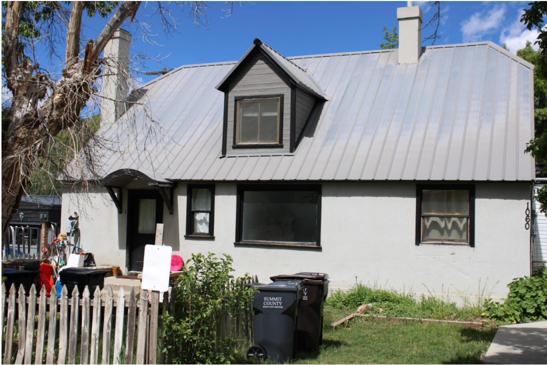
Photo 1: 1060 Woodside Avenue. West elevation. 2020
