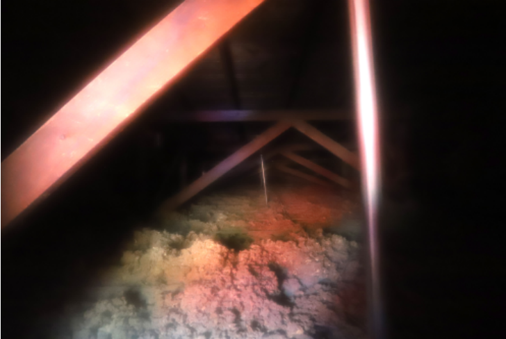
INSULATED ROOF / TRUSSES
