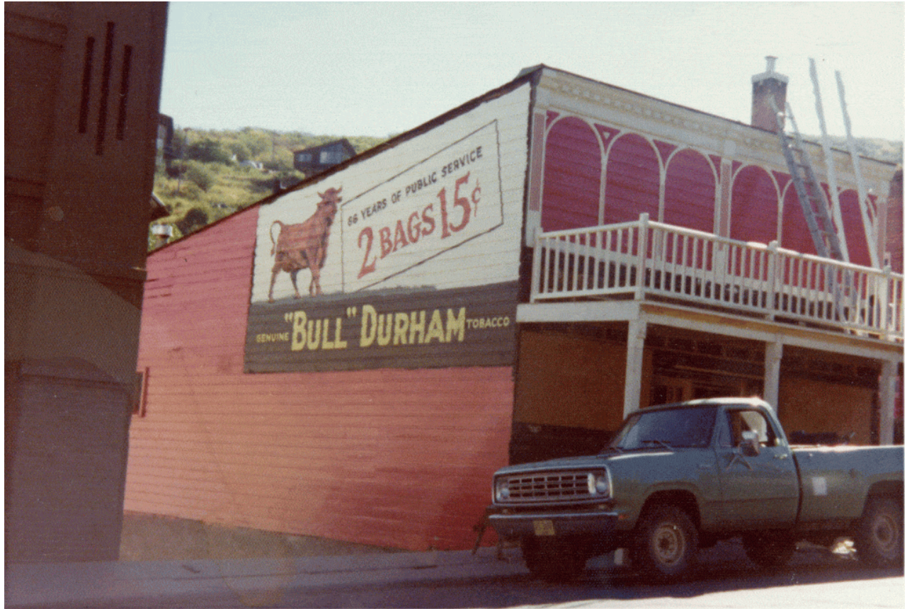
Figure 6. 322 Main Street in the late 1970s. The "Bull" Durham sign was uncovered during the 1976 renovations. The building appears to be under construction in this photograph. Source: Park City Museum, https://parkcityhistory.org/vanishing-bull-the-saga-of-a-celebrated-sign/ .
