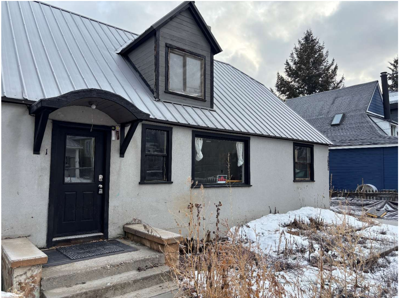
Figure 2. Modifications to the primary (west) façade include removal of the hipped roof at the entry, addition of a window opening south of the primary entrance, addition of a roof dormer, and roof cladding replacement.
