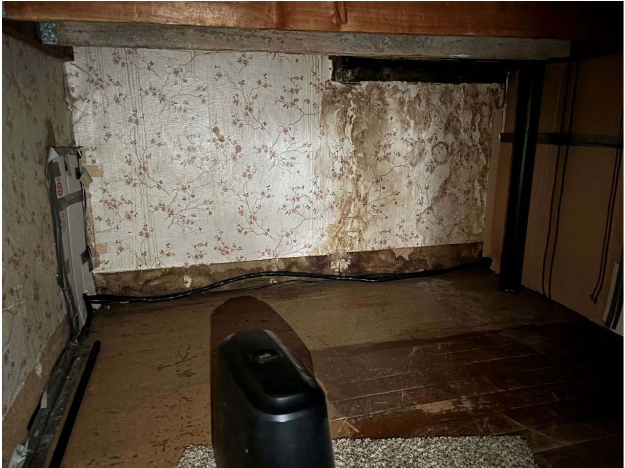
Figure 5. The original flooring appears to be extant in this closet.
