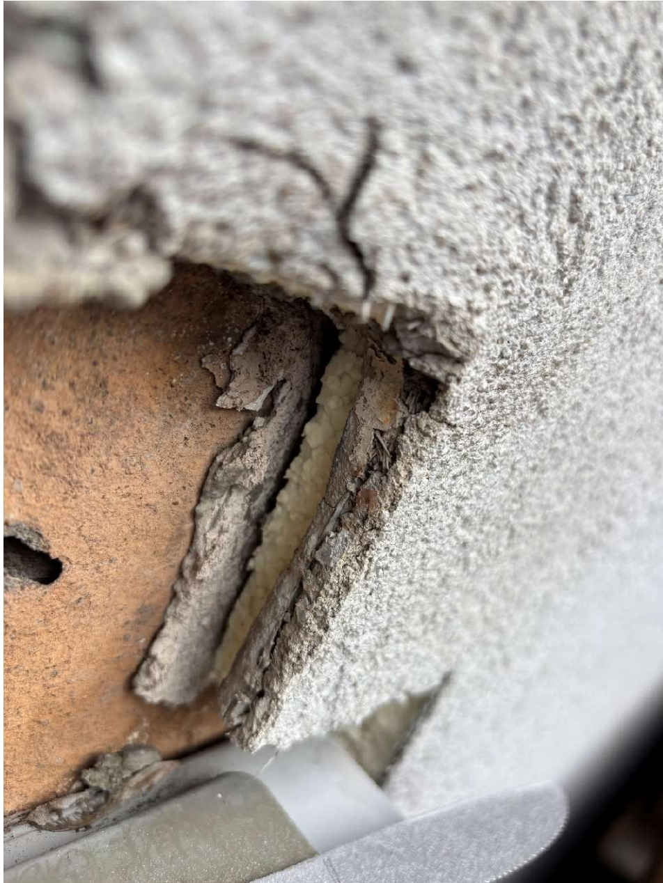
Figure 3. The exterior of the original building has been re-clad in EIFS. The addition is clad in EIFS.
