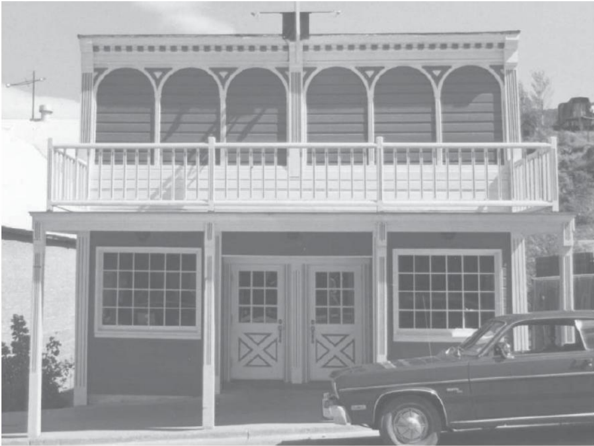
Figure 14: 1970s façade modifications with the 1899 arches on the second story and reduced storefront glazing. The transom windows are not replaced but a deck/balcony is added.
