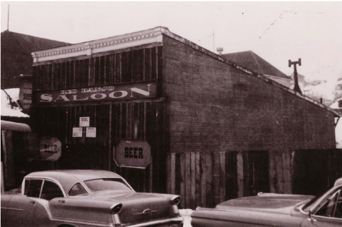
Figure 5: Photo of 322 Main Street likely from the 1960s showing a transition from brick and tile to a vertical wood facade
