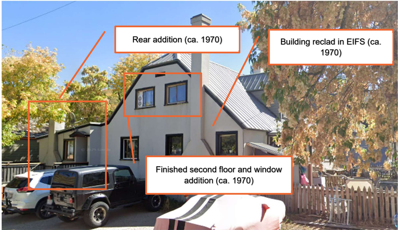
Figure 10. Building modification analysis, side (north) elevation. Source: Google StreetView 2024.
