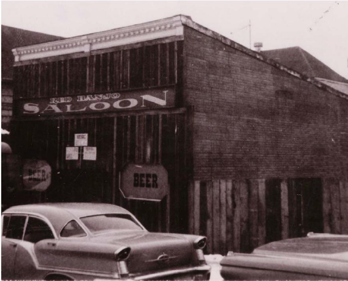
Figure 13: 1960s photo with horizontal expanse of glazing removed
