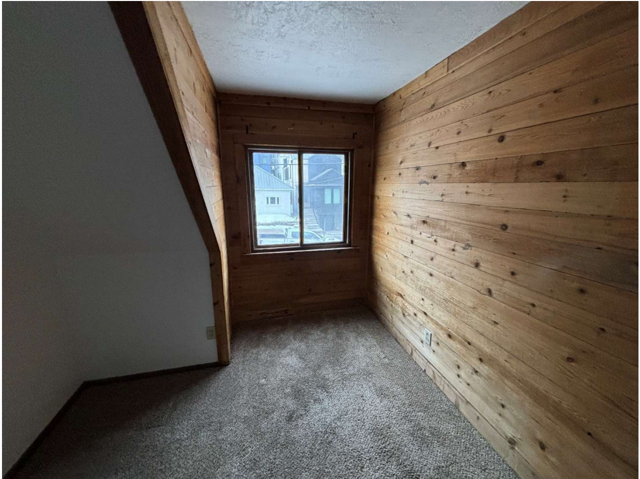
Figure 4. Interior modifications include a finished upper floor, new finishes to walls and flooring, and additional windows, including dormers and gable-end windows at the upper floor.
