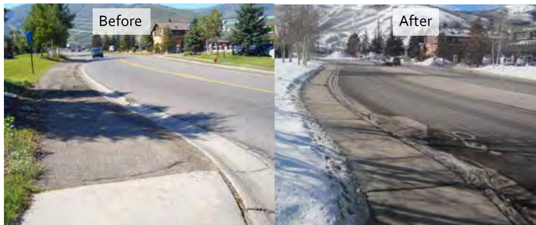
The 2012 renovations of Bonanza Drive introduced complete streets concepts with improved pedestrian crossing, turning lanes, bus pull-off areas, pedestrian signalization, and bike lanes.
