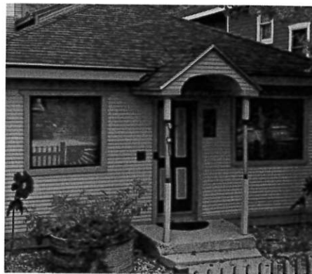
Existing wood posts.
