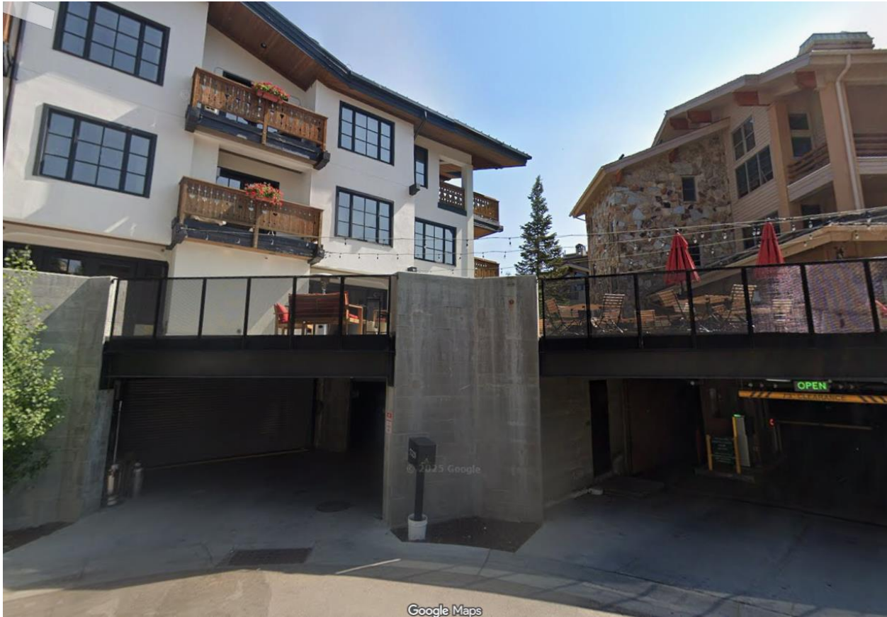
Figure 5: An image showing the patio is located above Grade on top of the Parking Garage.
