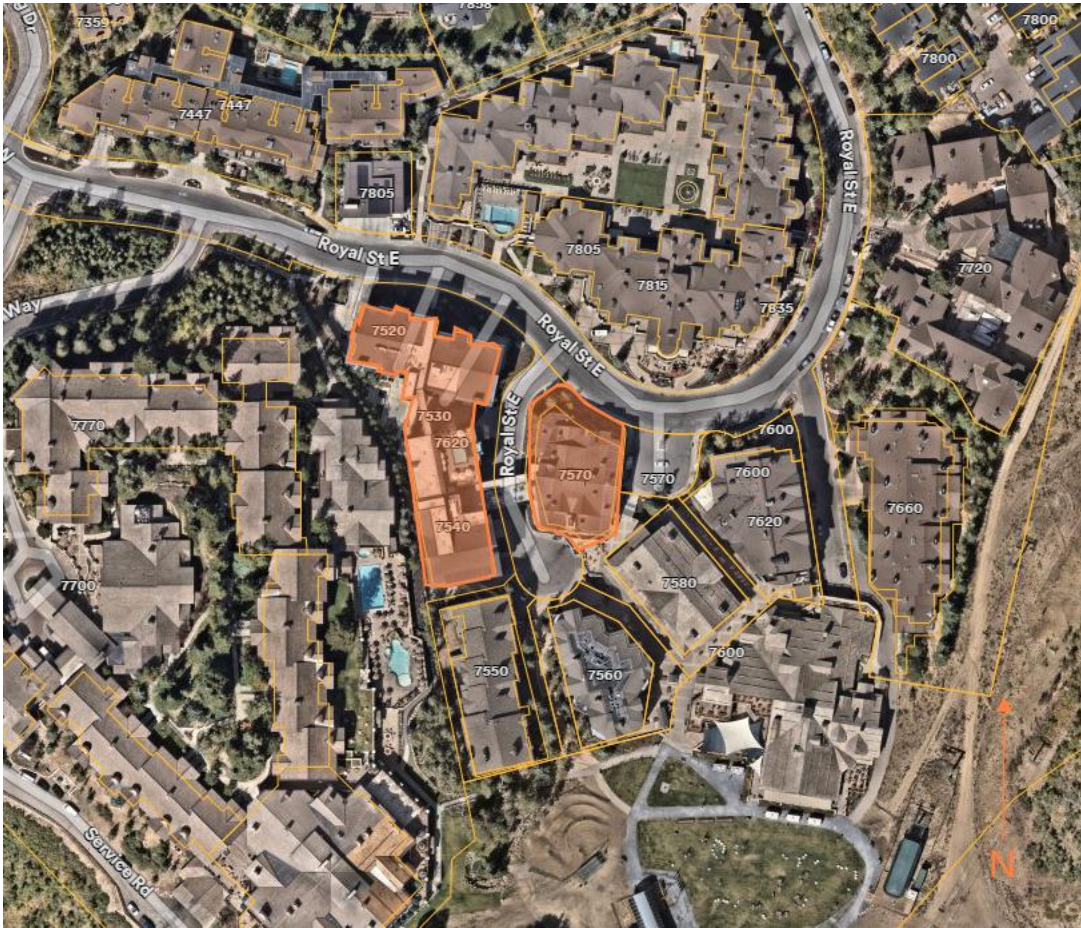
Figure 1: The Goldener Hirsch is highlighted in orange. To the north is the Park City Fire District Station and The Chateaux. To the south is Deer Valley Resort and the Silver Lake Lodge.
