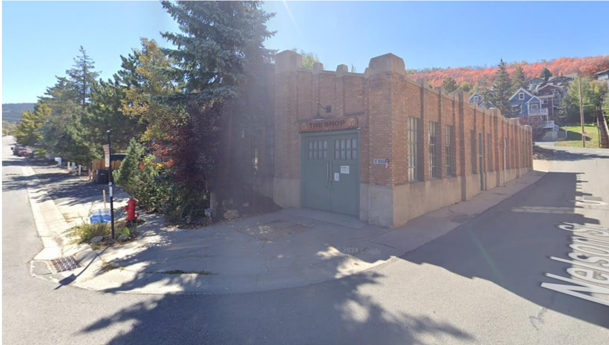
Figure 1: 1167 Woodside Ave Viewed from the Northeast Corner
