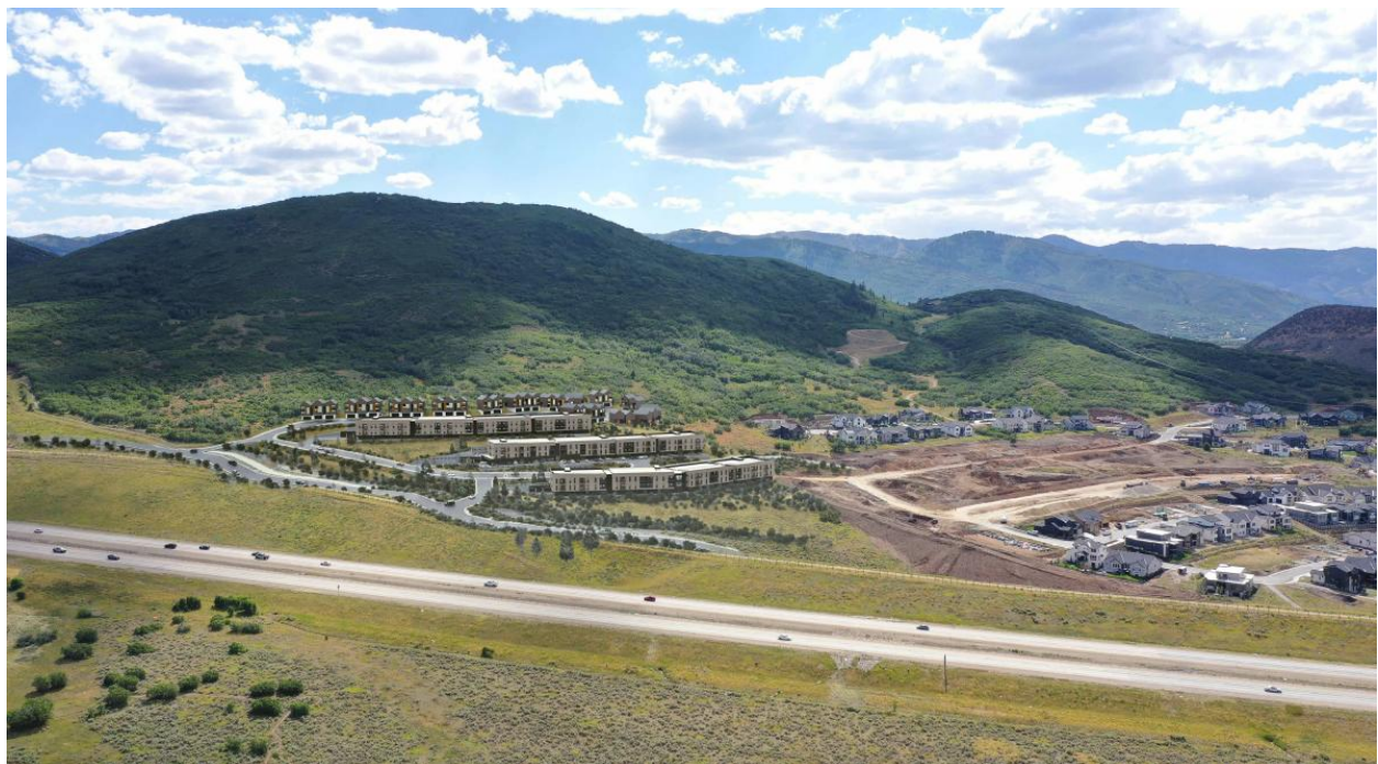
Figure 8: Proposed development viewed across HWY 40 provided by the Applicant.
