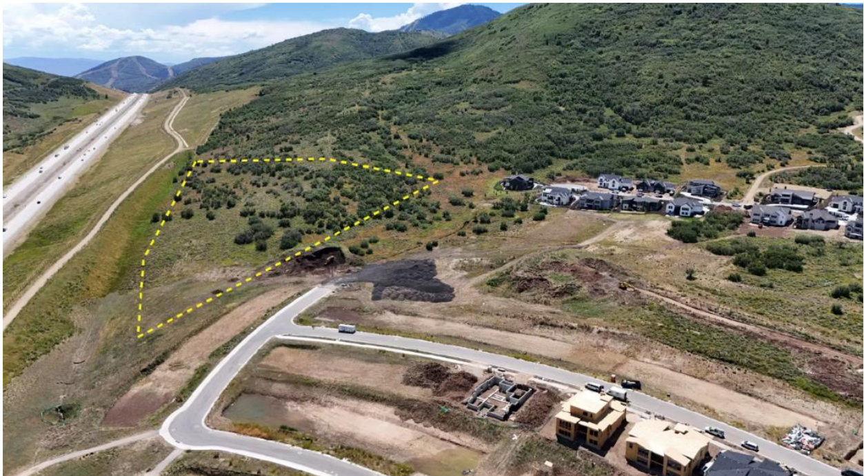
Figure 4: The area proposed within the Clark Ranch property for the affordable housing development.
