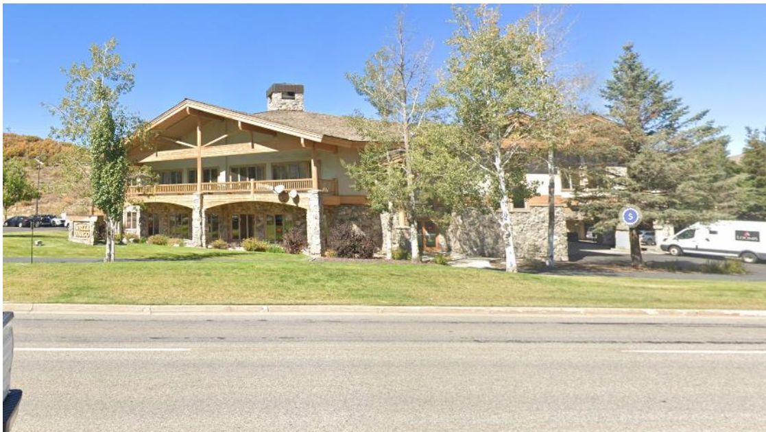
Figure 18: Wells Fargo Building, Image from Google Street View
