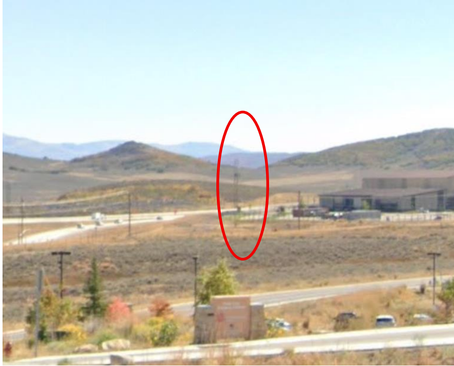
Figure 9: Image from Google Streetview with the Telecommunication Facility shown in red. Located at the roundabout at the Park City Hospital (900 Round Valley Drive) Vantage Point.
