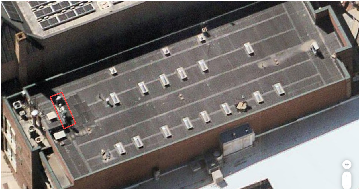
Figure 2: Nearmap oblique view of the 340 Main Street roof; the Telecommunications equipment is within the red rectangle.
