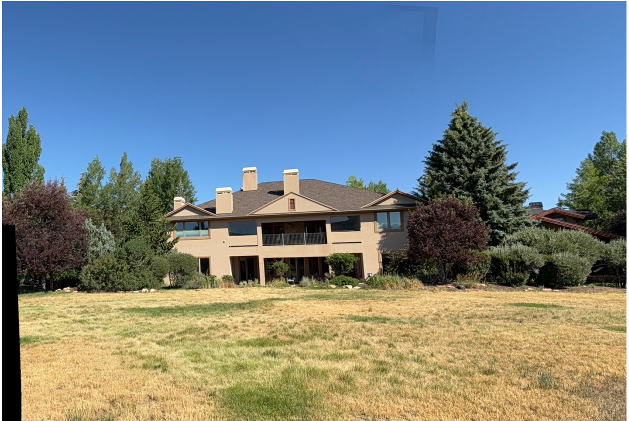
Rear of the house. East Facing.
