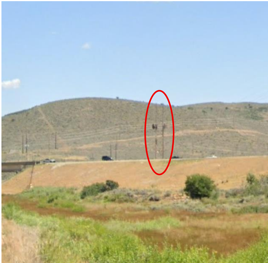
Figure 8: Image from Google Streetview with the Telecommunication Facility shown in Red. Located at the intersection of the Rail Trail and Richardson Flat Road Vantage Point.
