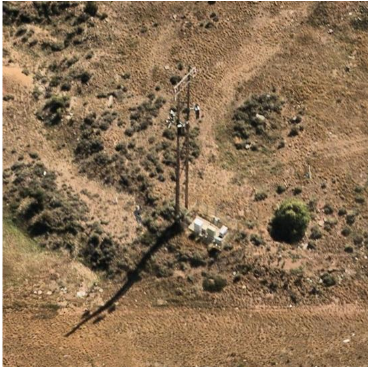
Figure 3: Oblique aerial view of the Telecommunications Facility.
