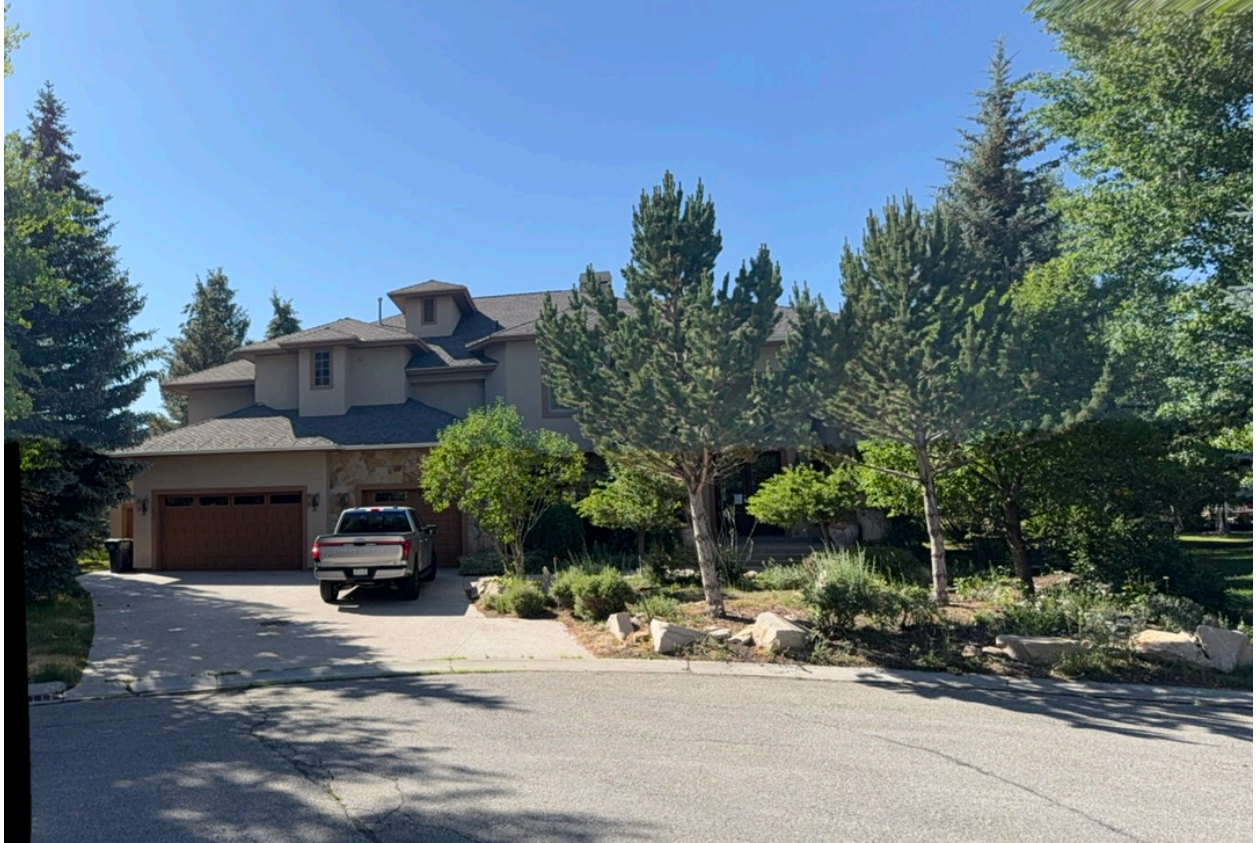
Front of the House. West Facing
