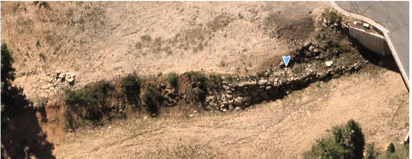
Figure 2: Oblique view showing the topography along the northeast property boundary between the Sunrise Ski Run and 7955 Red Tail Ct. The existing rock retaining walls can be seen at the center right.
