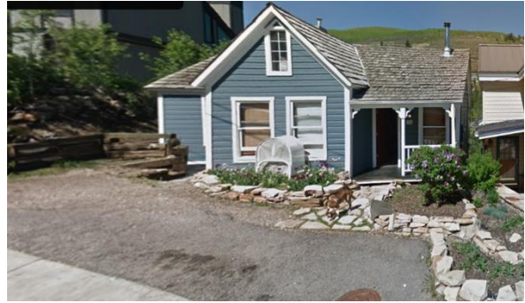
Figure 1: 36 Prospect Avenue viewed from Prospect Avenue, image from Google Maps.
