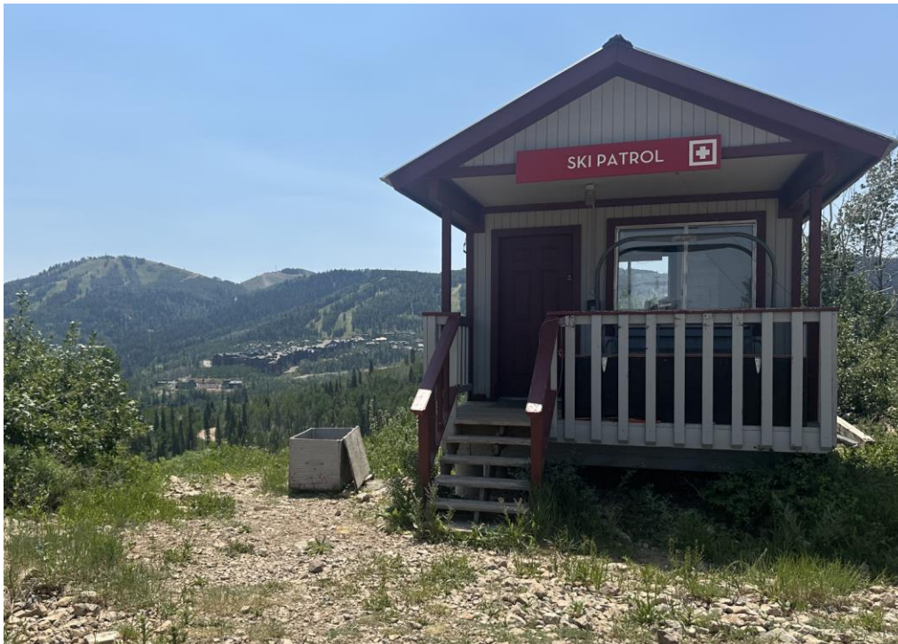
Figure 5: The existing ski patrol hut. Empire Pass can be seen in the background. Photo provided by Applicant (Exhibit B).
