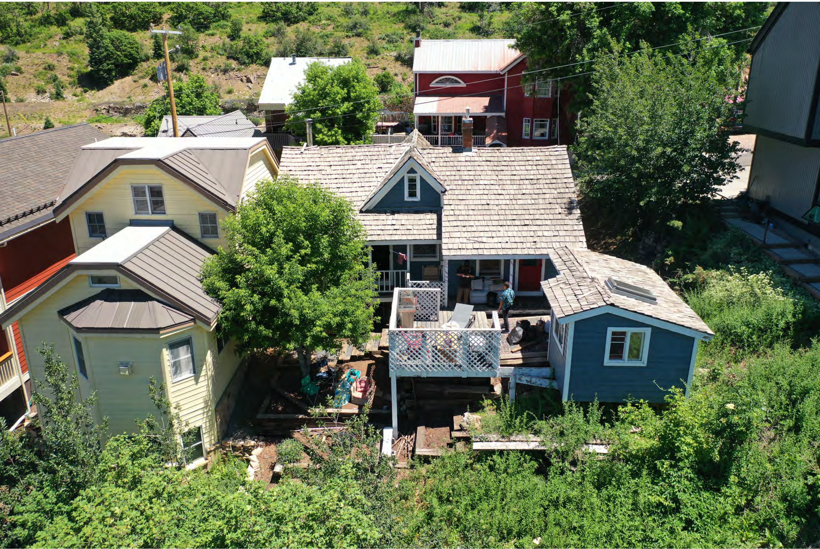
WEST VIEW OF PROJECT LOCATION
