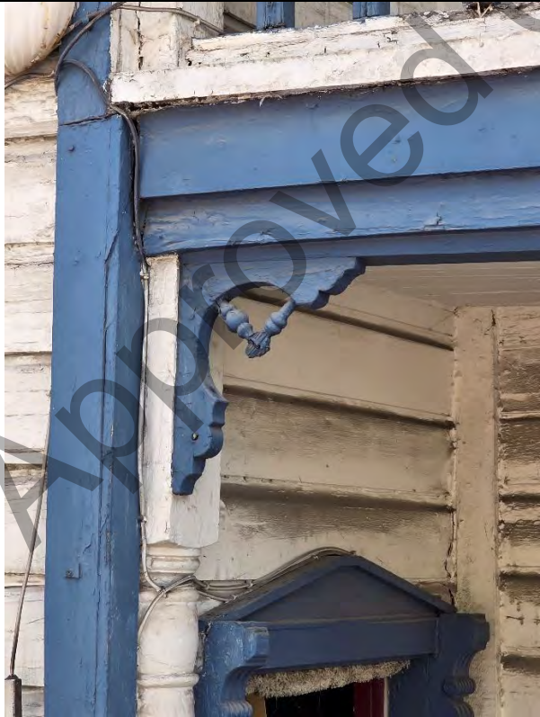
Lead exterior trim
