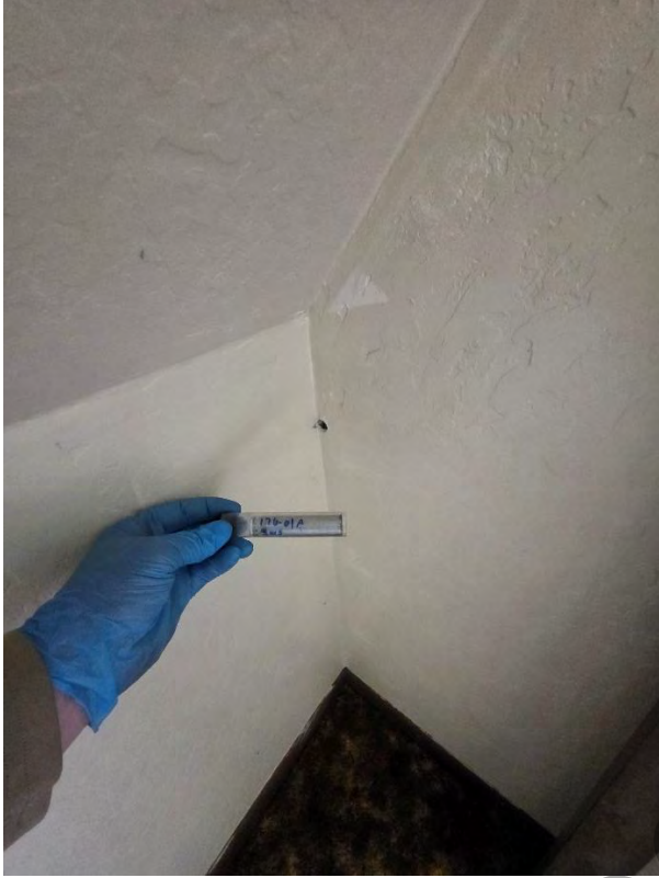
176 – 01A Sheetrock Wall System
