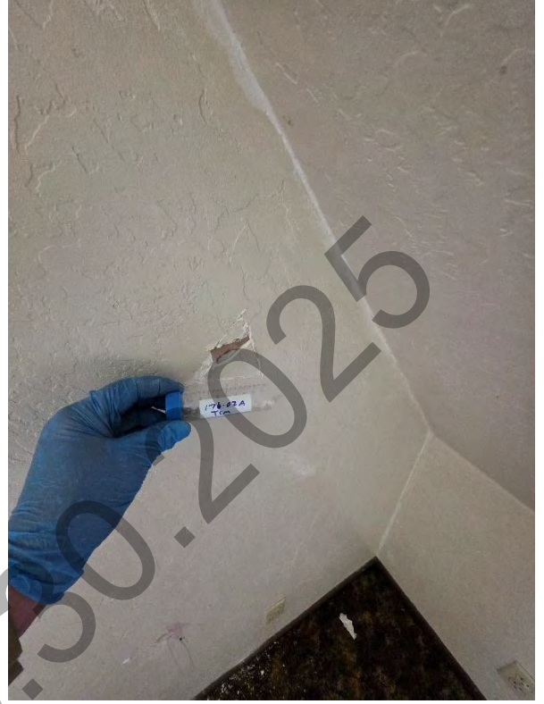
176 – 02A Textured Wall/Ceiling Material
