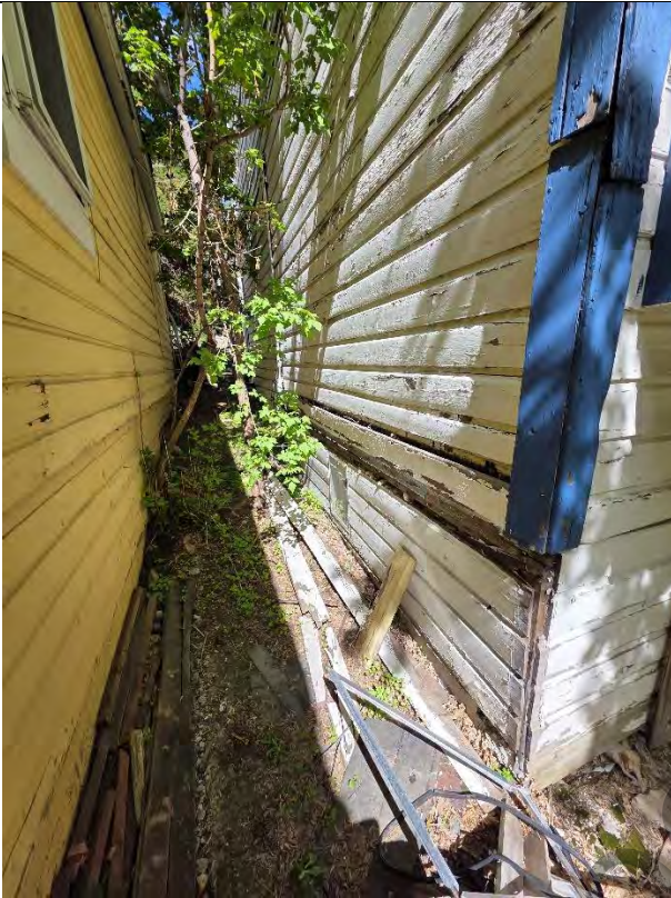
Lead exterior siding and trim
