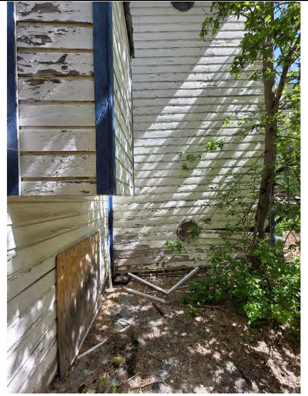
Lead exterior siding and trim
