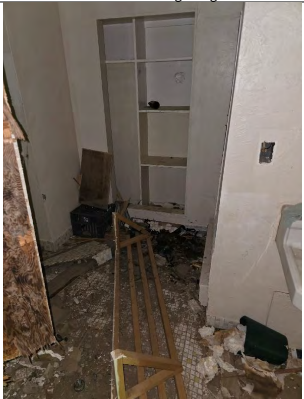
Basement South Apartment bathroom
