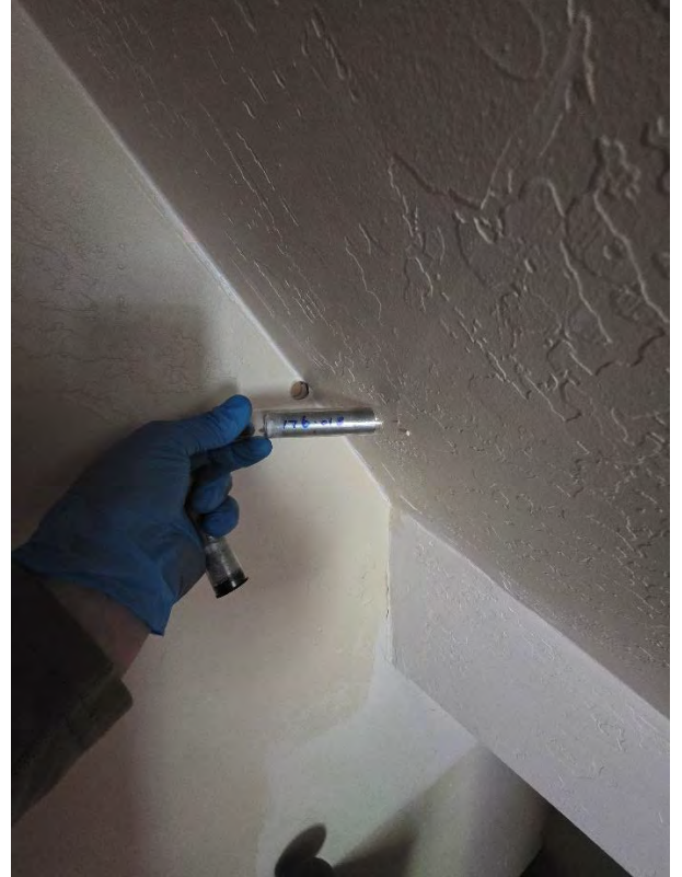
176 – 01B Sheetrock Wall System
