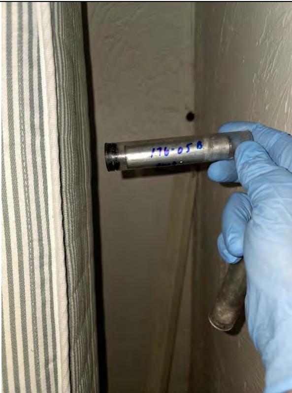
176 – 05B Sheetrock Wall System
