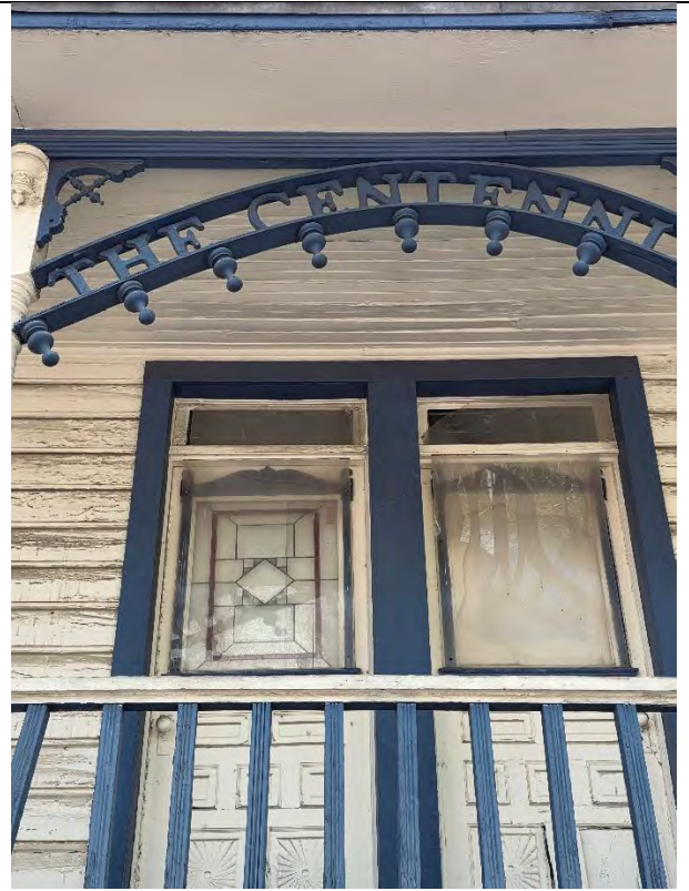
Exterior window frame, stair stringers and trim
