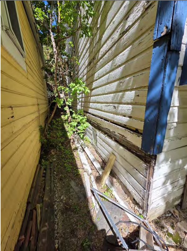
Lead exterior siding and trim
