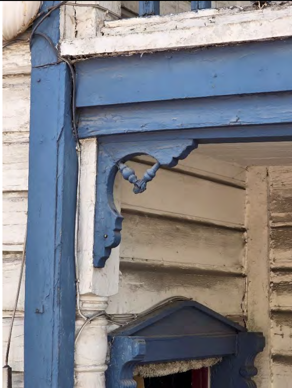
Lead exterior trim
