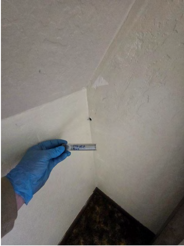
176 – 01A Sheetrock Wall System
