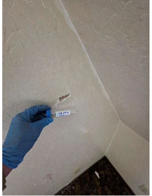
176 – 02A Textured Wall/Ceiling Material
