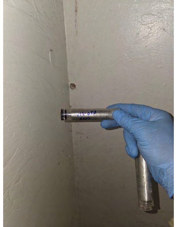
176 – 05A Sheetrock Wall System
