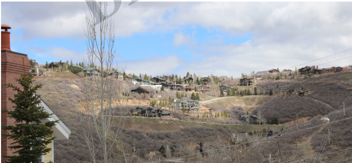
View of the neighborhood
