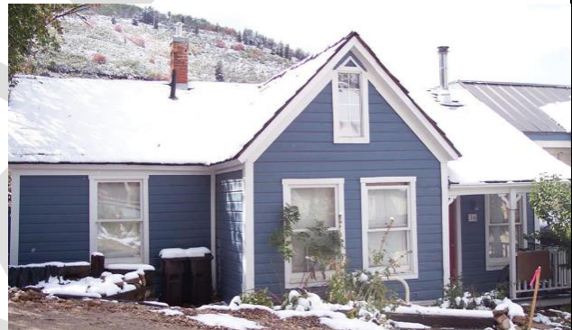
Figure 14: Recent photo provided by Applicant showing exterior changes.
