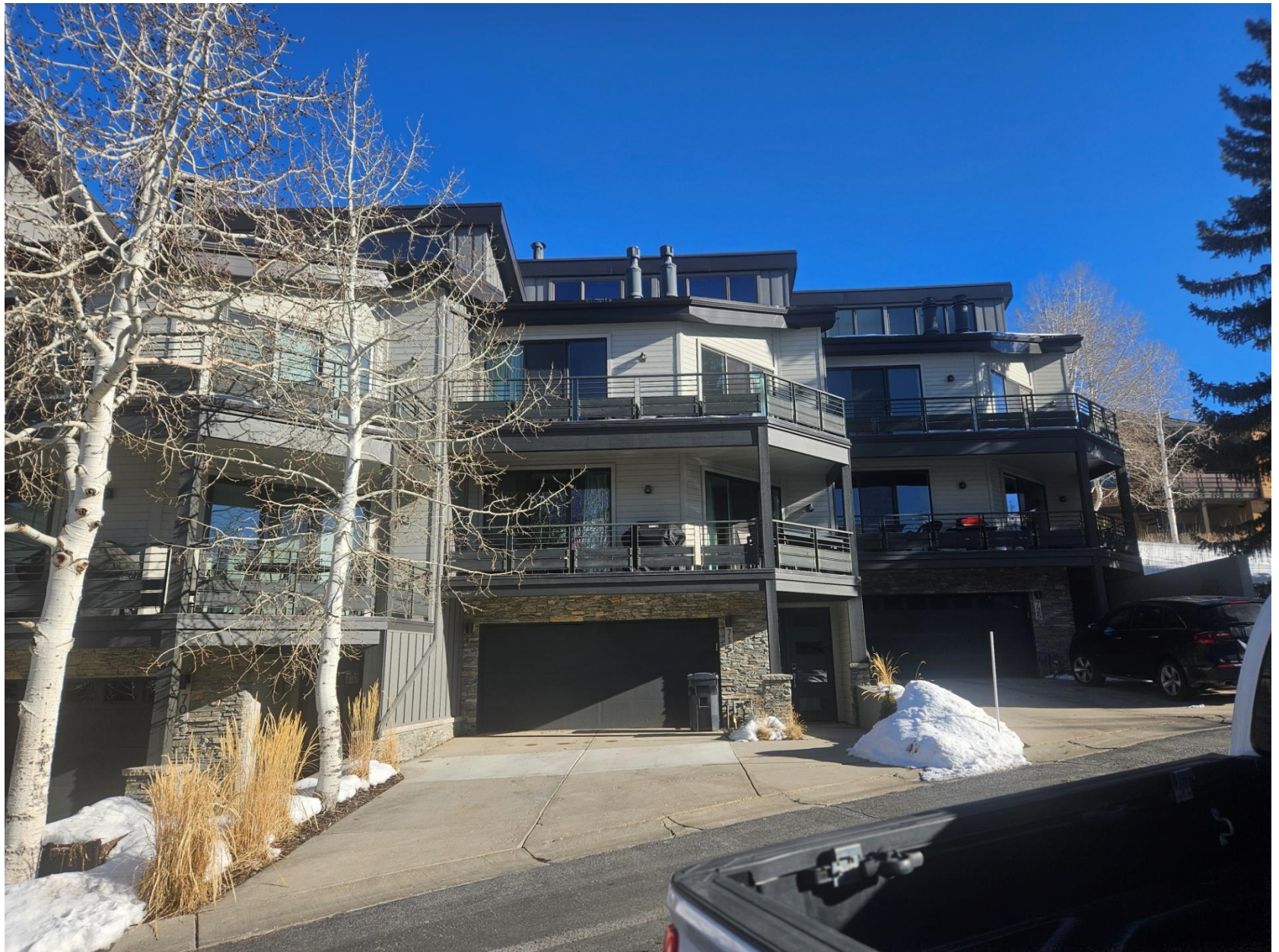
715 Saddle View Way – Looking northeast
