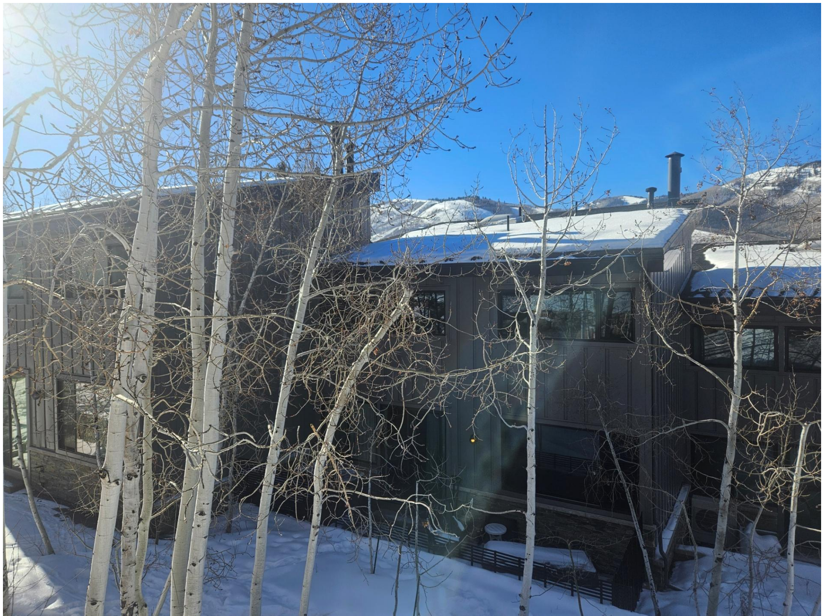
715 Saddle View Way – Looking southerly
