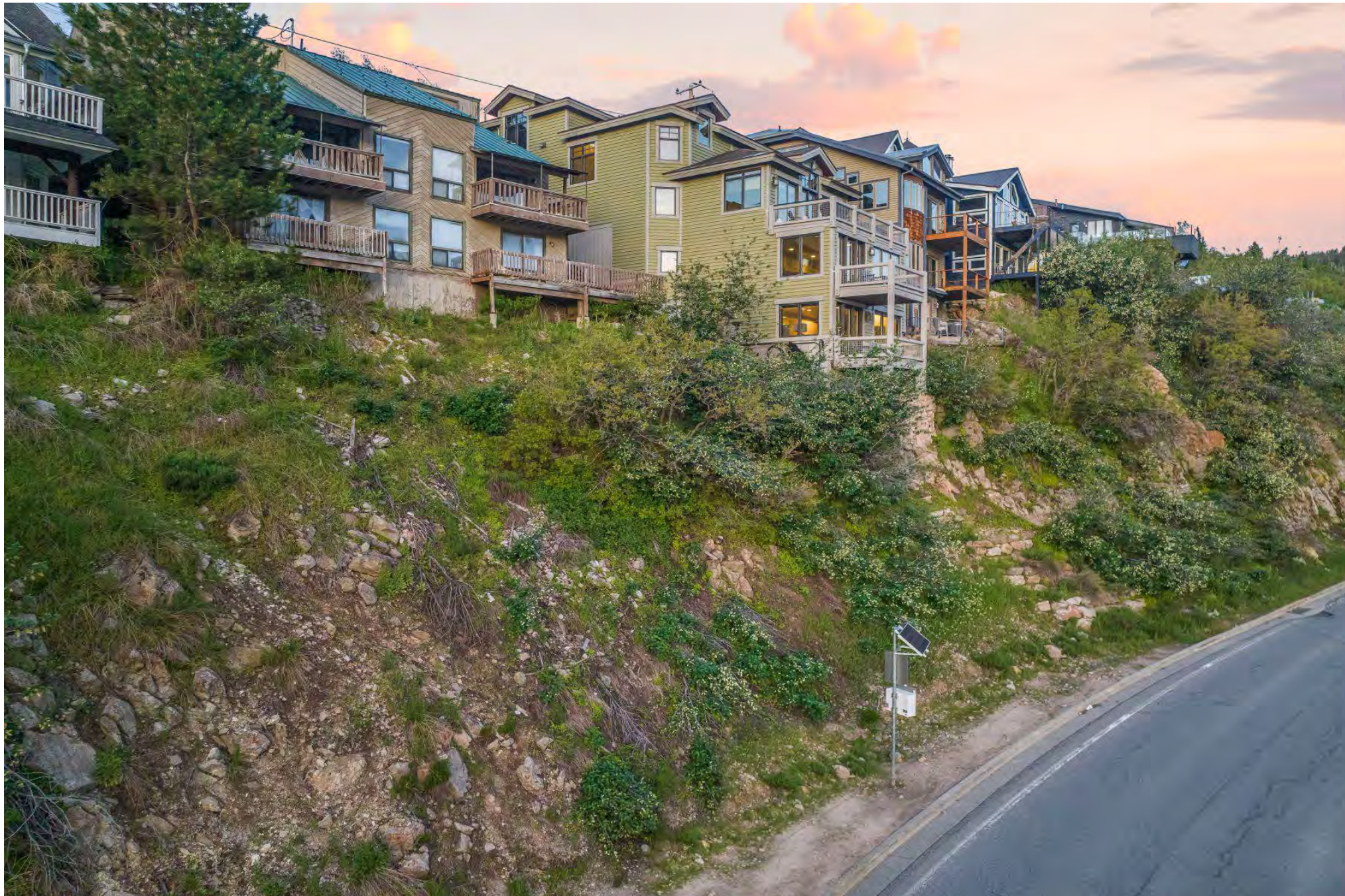
06 - View South towards project site
