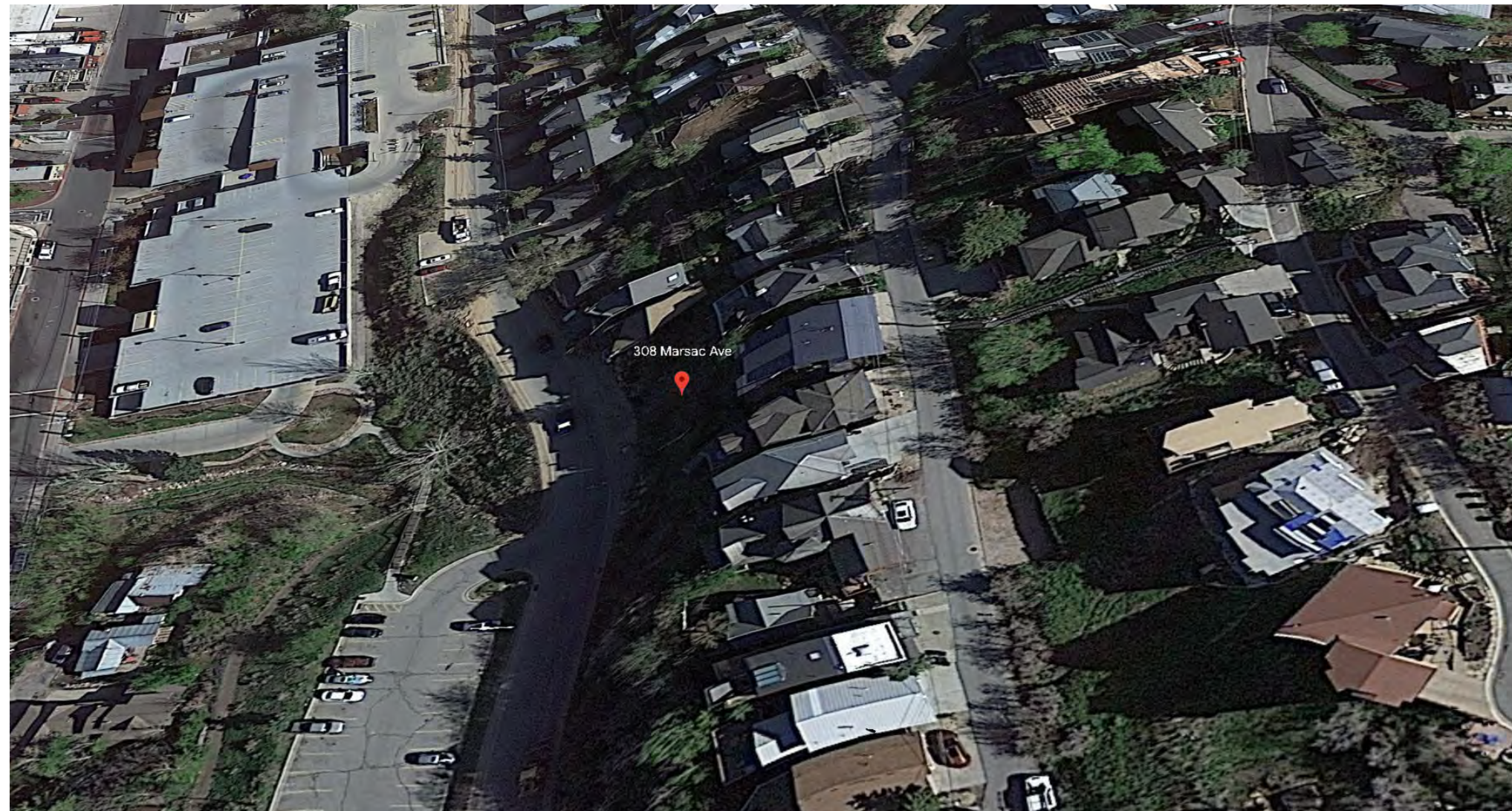
S - View towards project site from South
