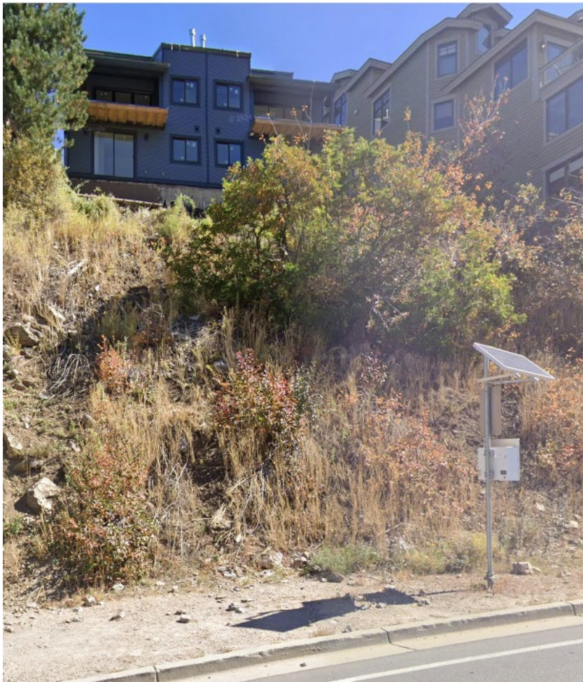
Figure 3: The Duplex at 301 and 303 Ontario Avenue that encroaches onto 301 Marsac Avenue visible from Google
