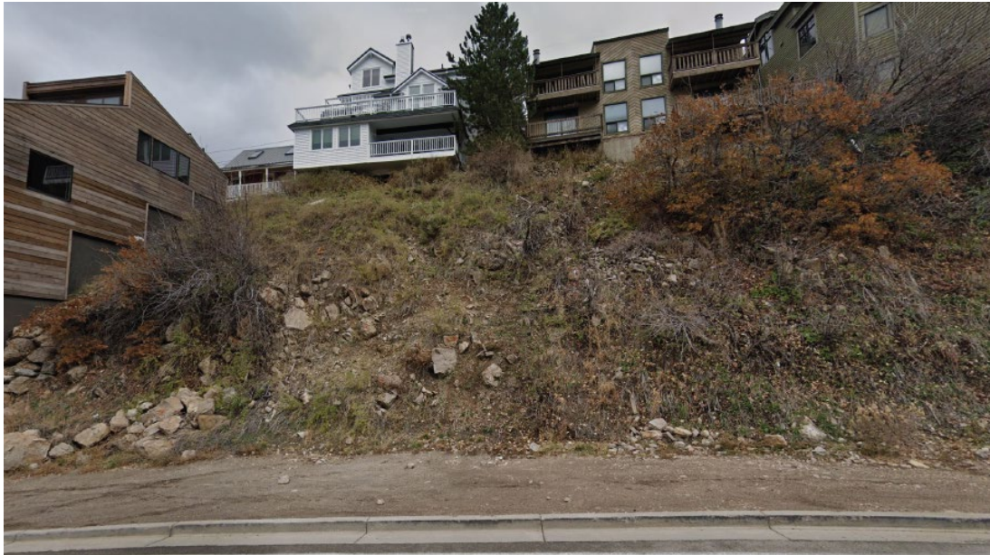
Figure 4: Image from Applicant's submittal showing the Very Steep Slopes at 301 Marsac Avenue.
