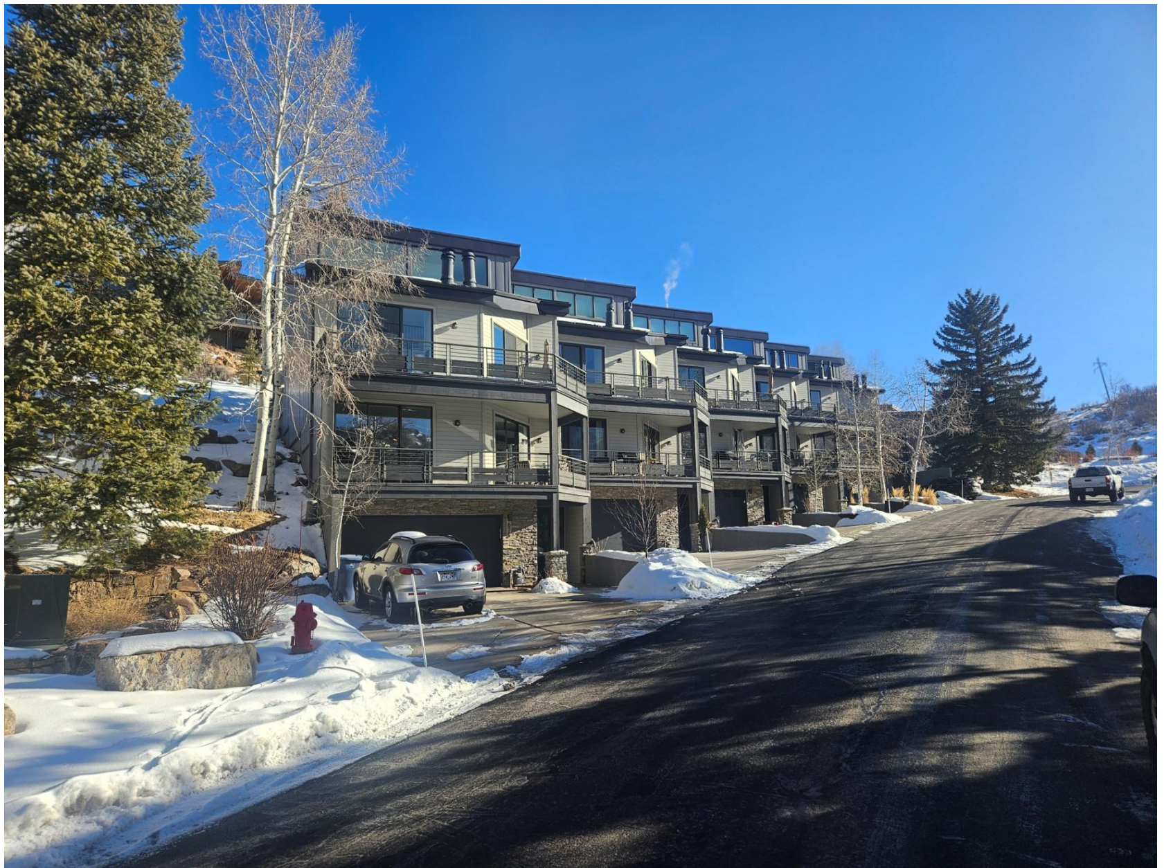
685 Saddle View Way – Looking easterly
