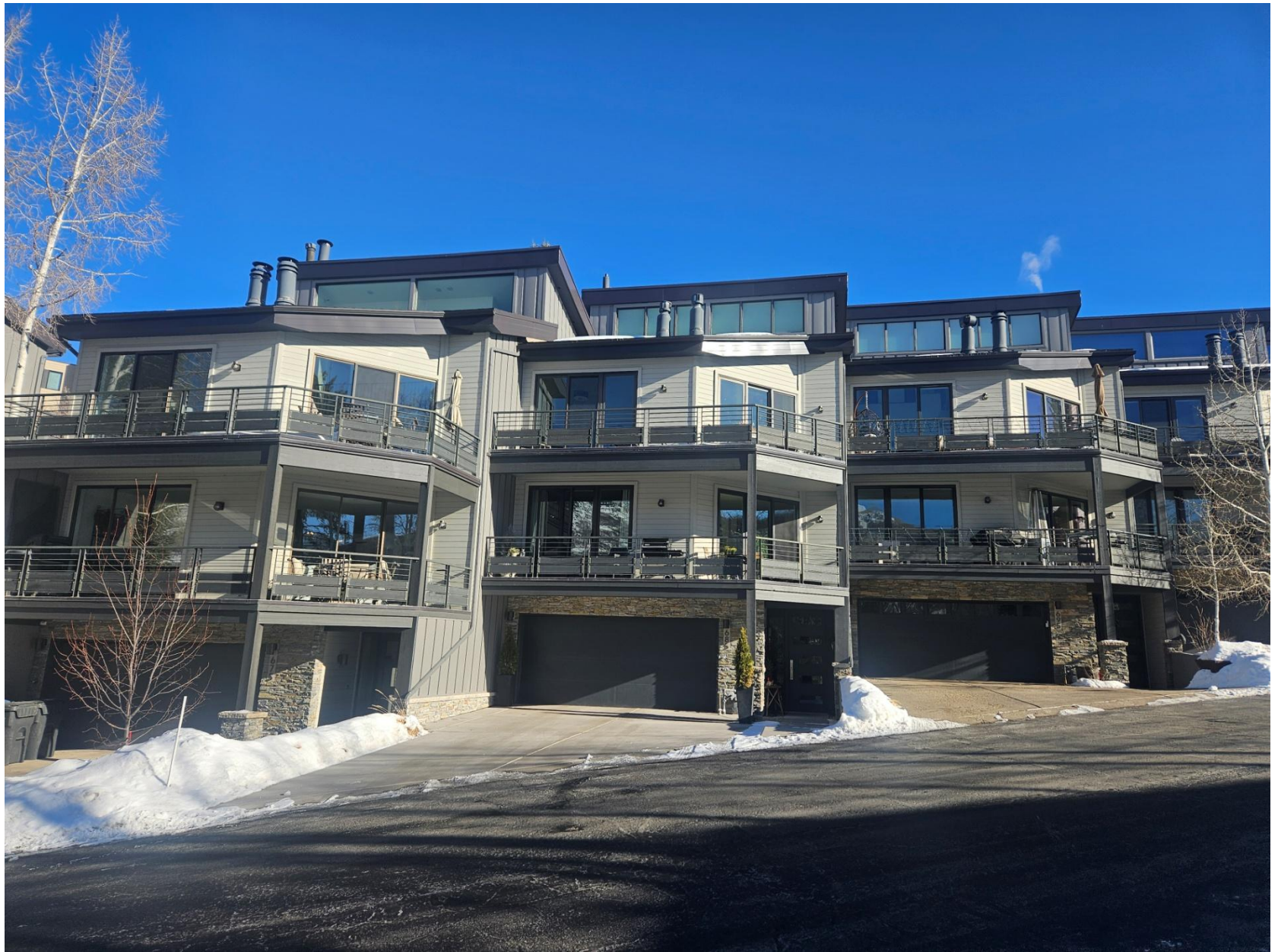
685 Saddle View Way - Looking northeast
