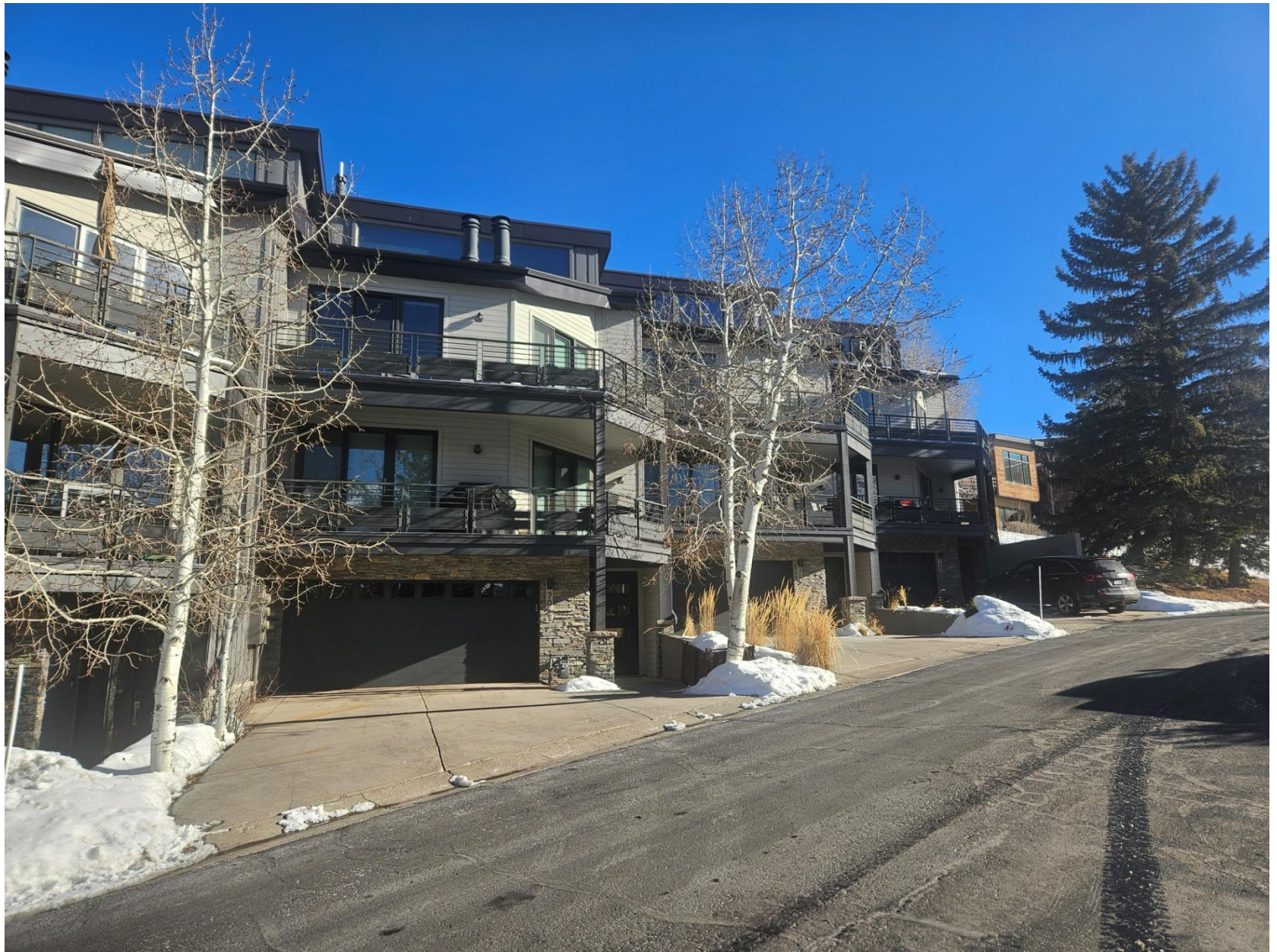
715 Saddle View Way – Looking east
