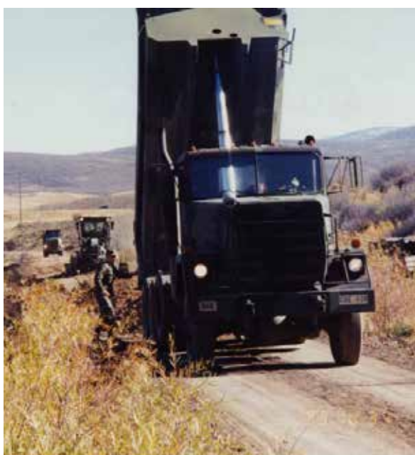
Construction of the Rail Trail
