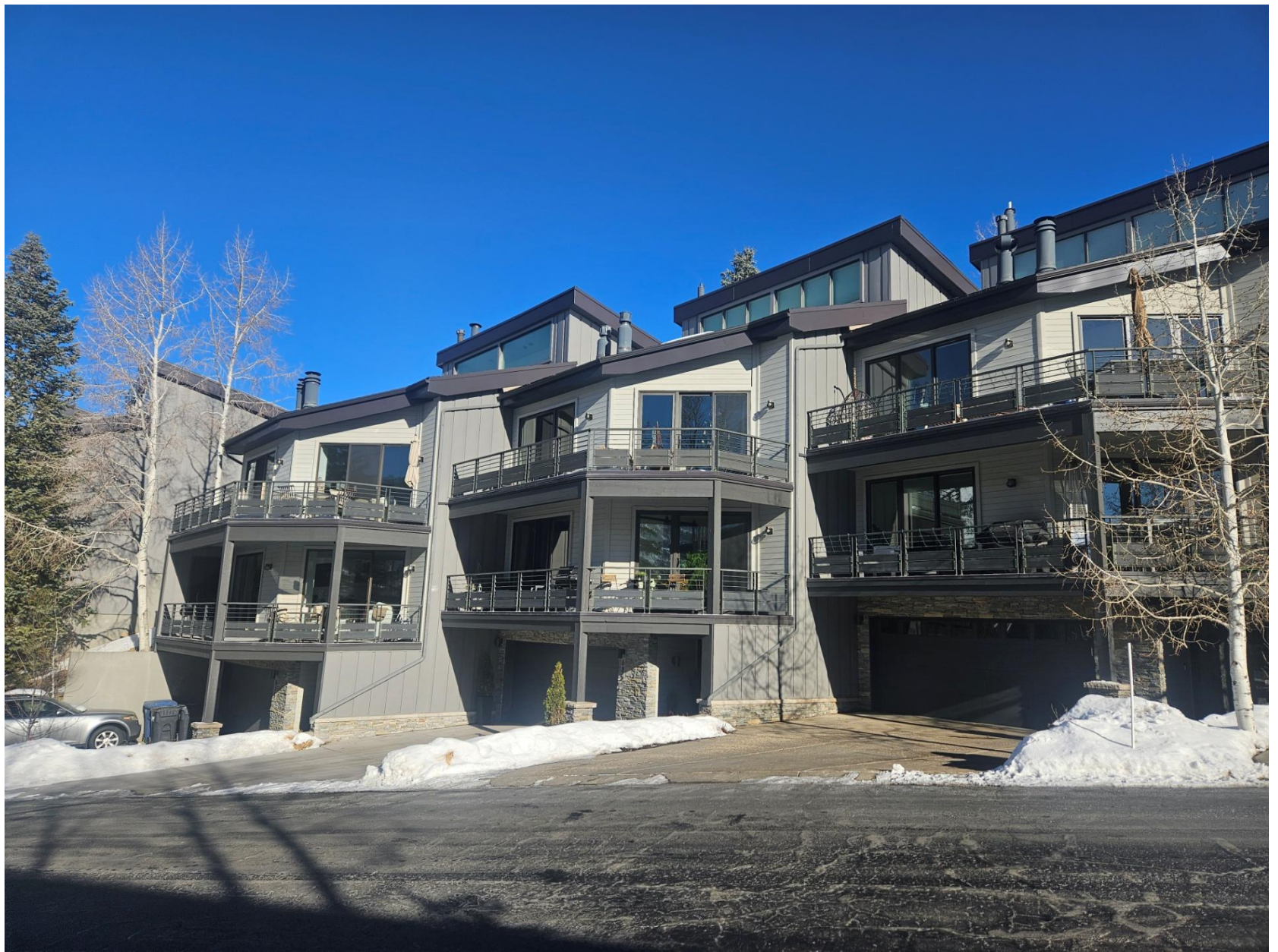
685 Saddle View Way – Looking north
