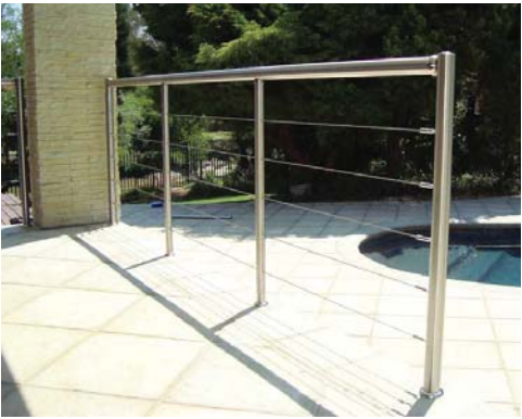
FENCING IMAGERY TENSILE CABLES AND STEEL CROSS BRACING
