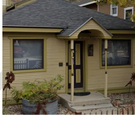
Existing wood posts.
