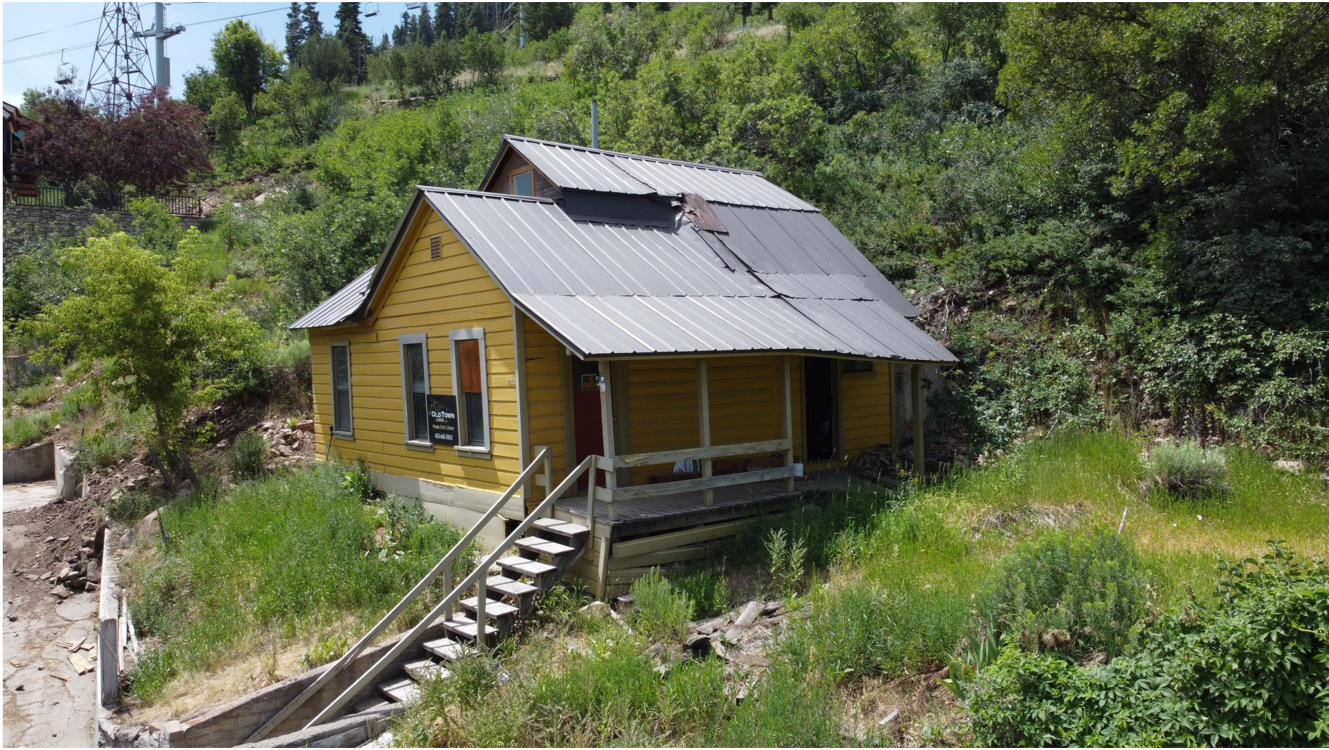
EXISTING HISTORIC ROOFING METAL
