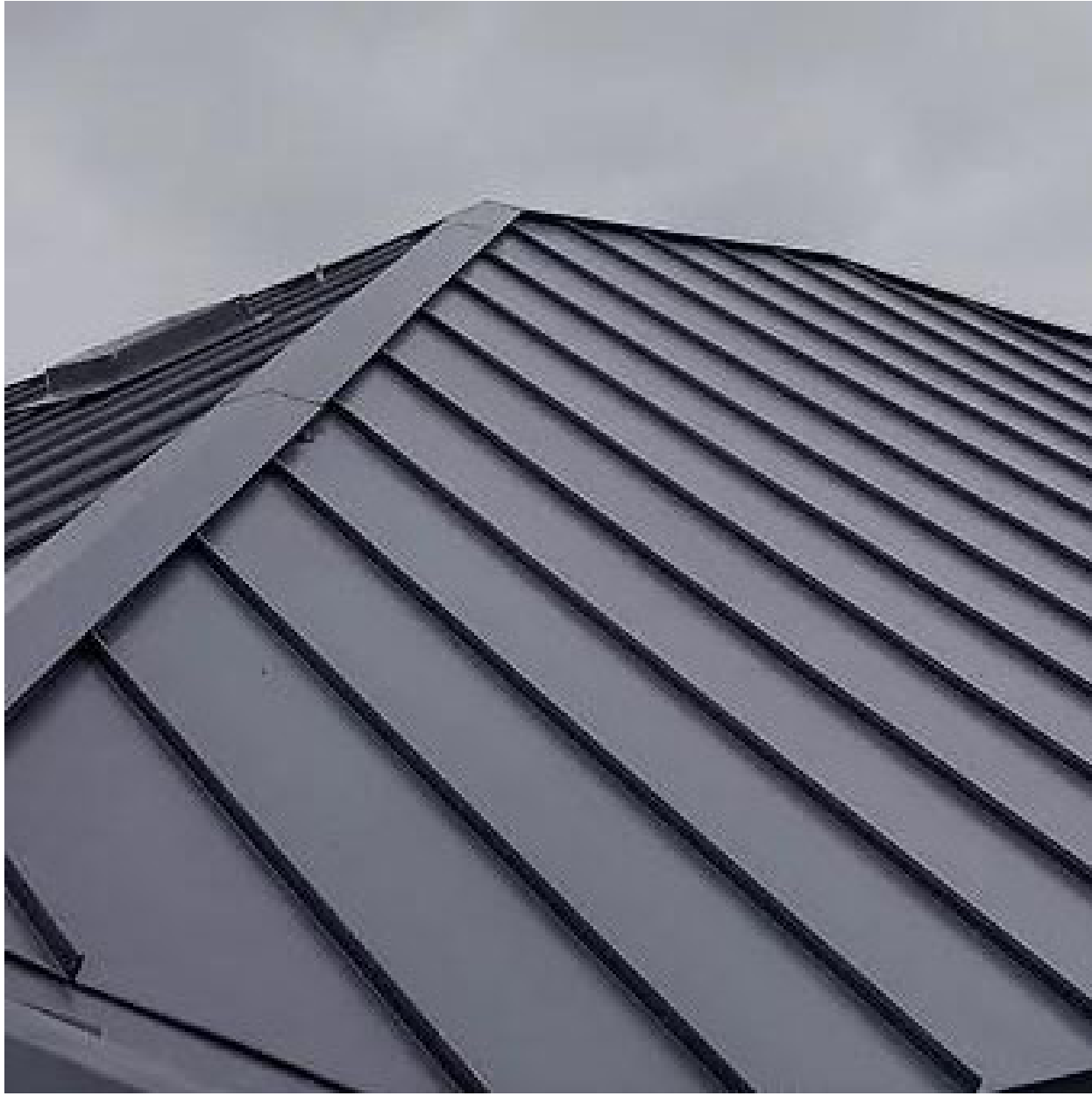
ADDITION STANDING SEAM ROOF
