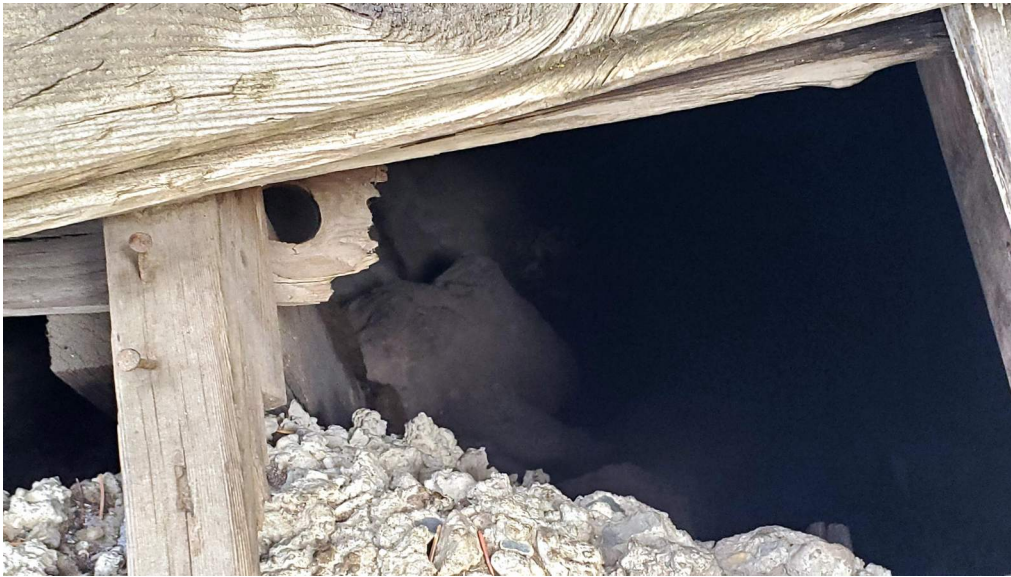
PHOTO #2 - FRONT DECK/ FOUNDATION STRUCTURE
