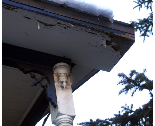
Upper Front Deck corner post
