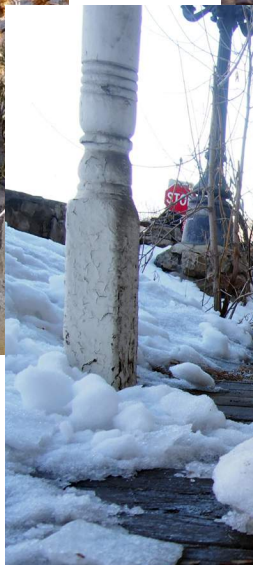
Base of Front Porch Post
