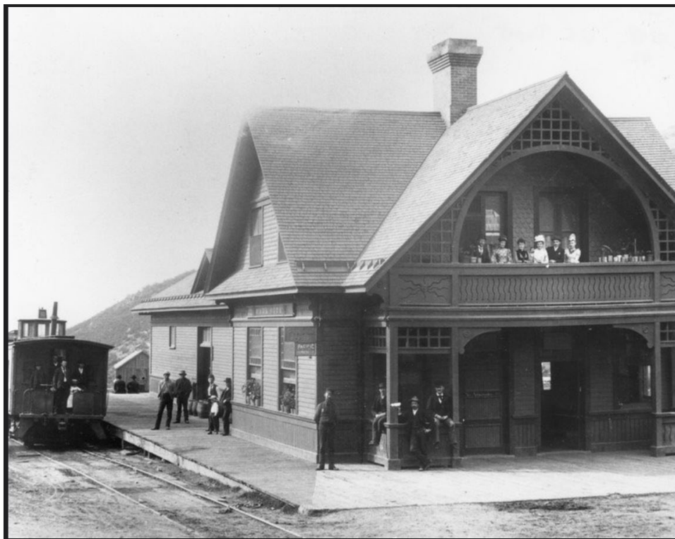
Figure A-9. A covered two-story porch on the Park City Union Pacific Depot, ca. 1910 (Park City Museum 2023).
