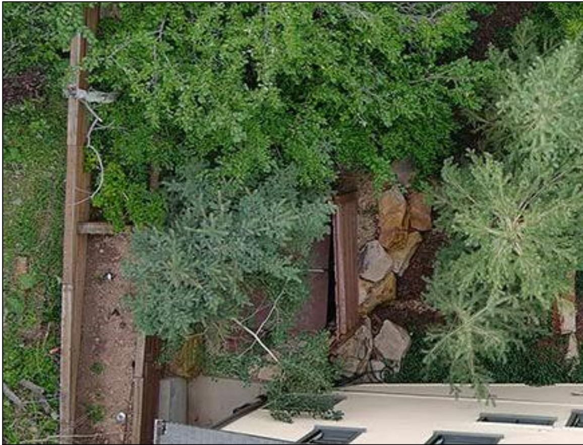
AERIAL OF EXISTING SPA AND RETAINING TO BE REMOVED
