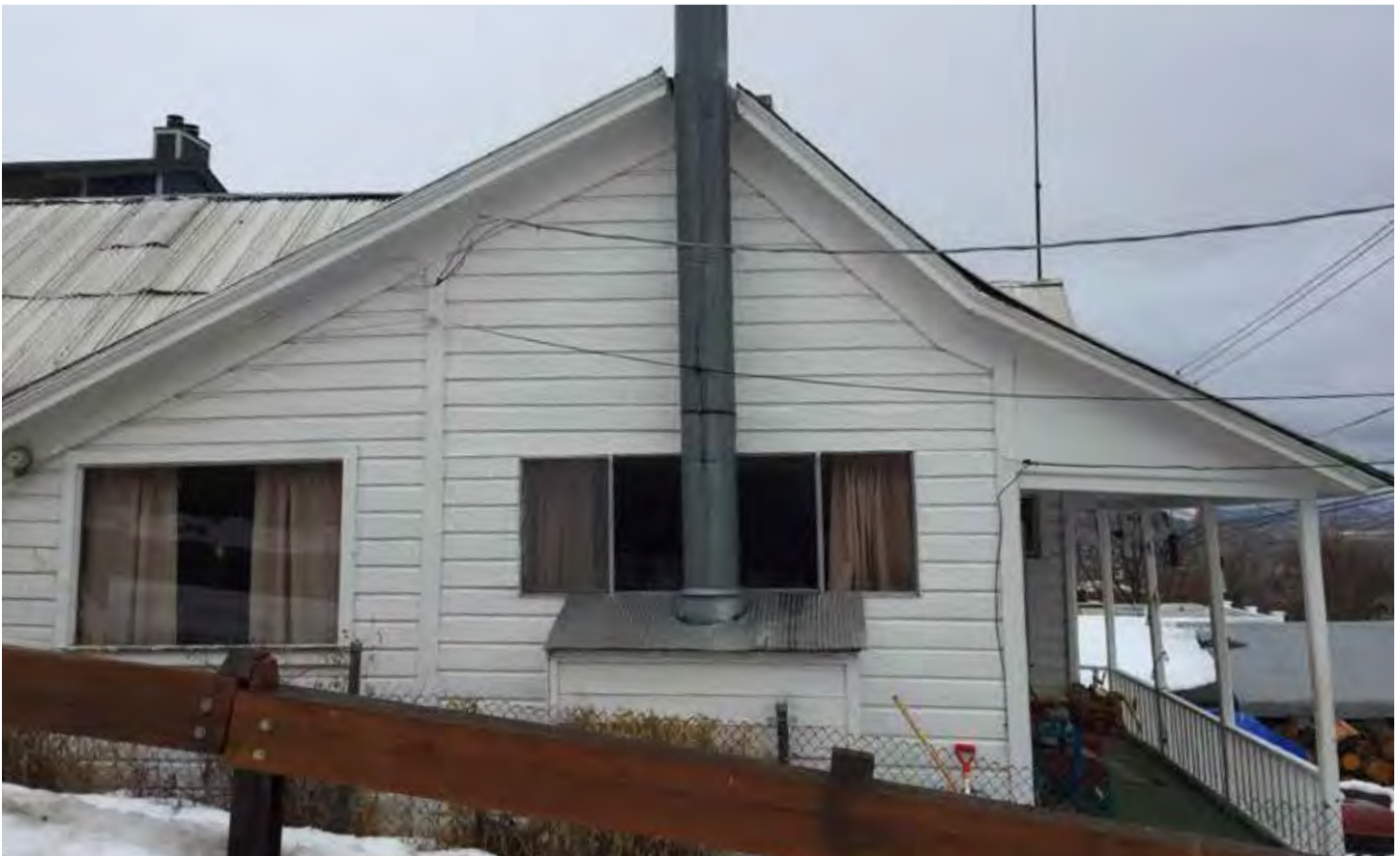
Photo #28: South Facade
