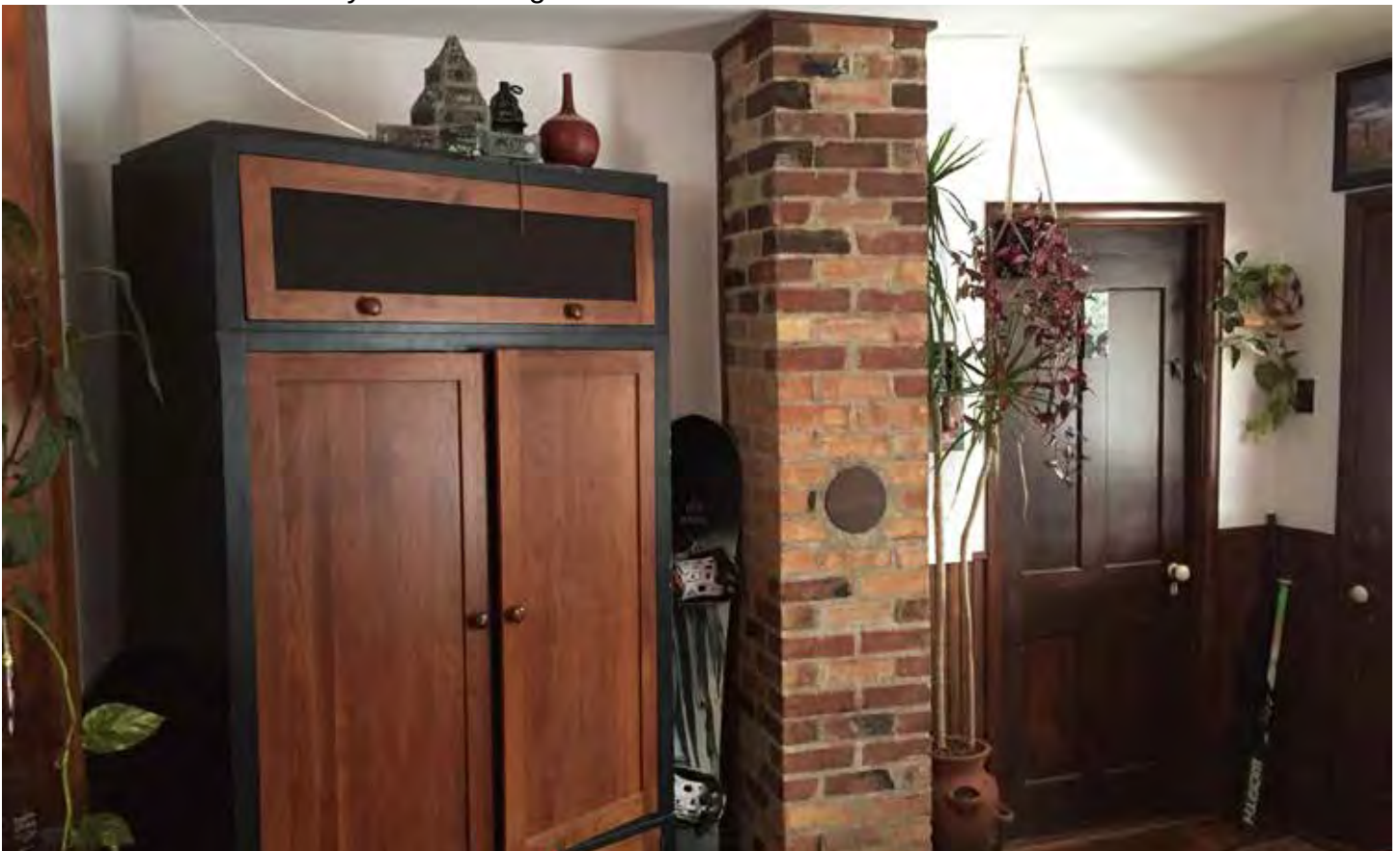
Photo #21: Front Chimney Within Living Room
