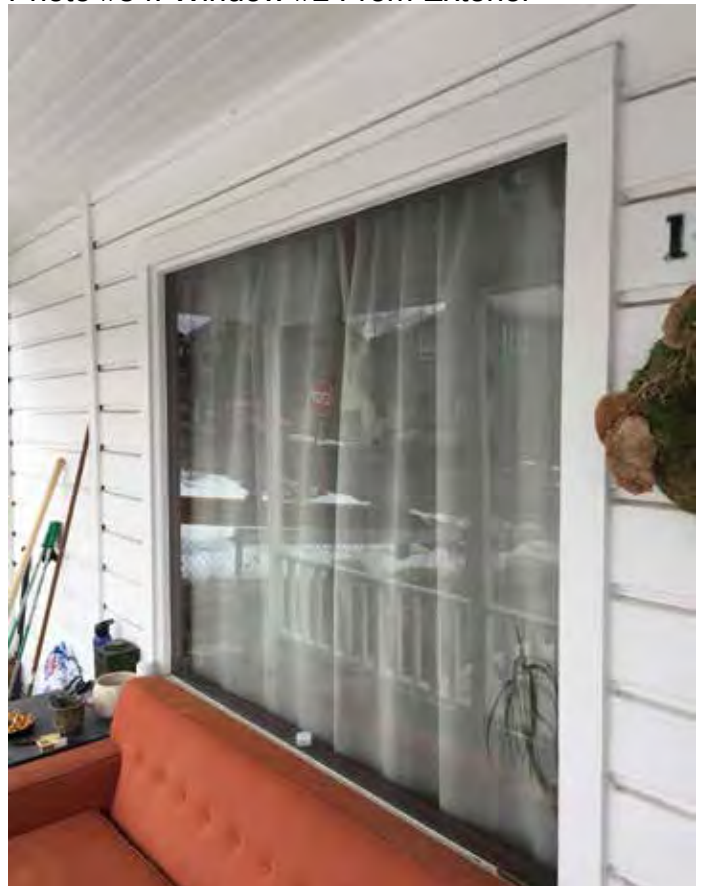
Photo #54: Window #2 From Exterior
