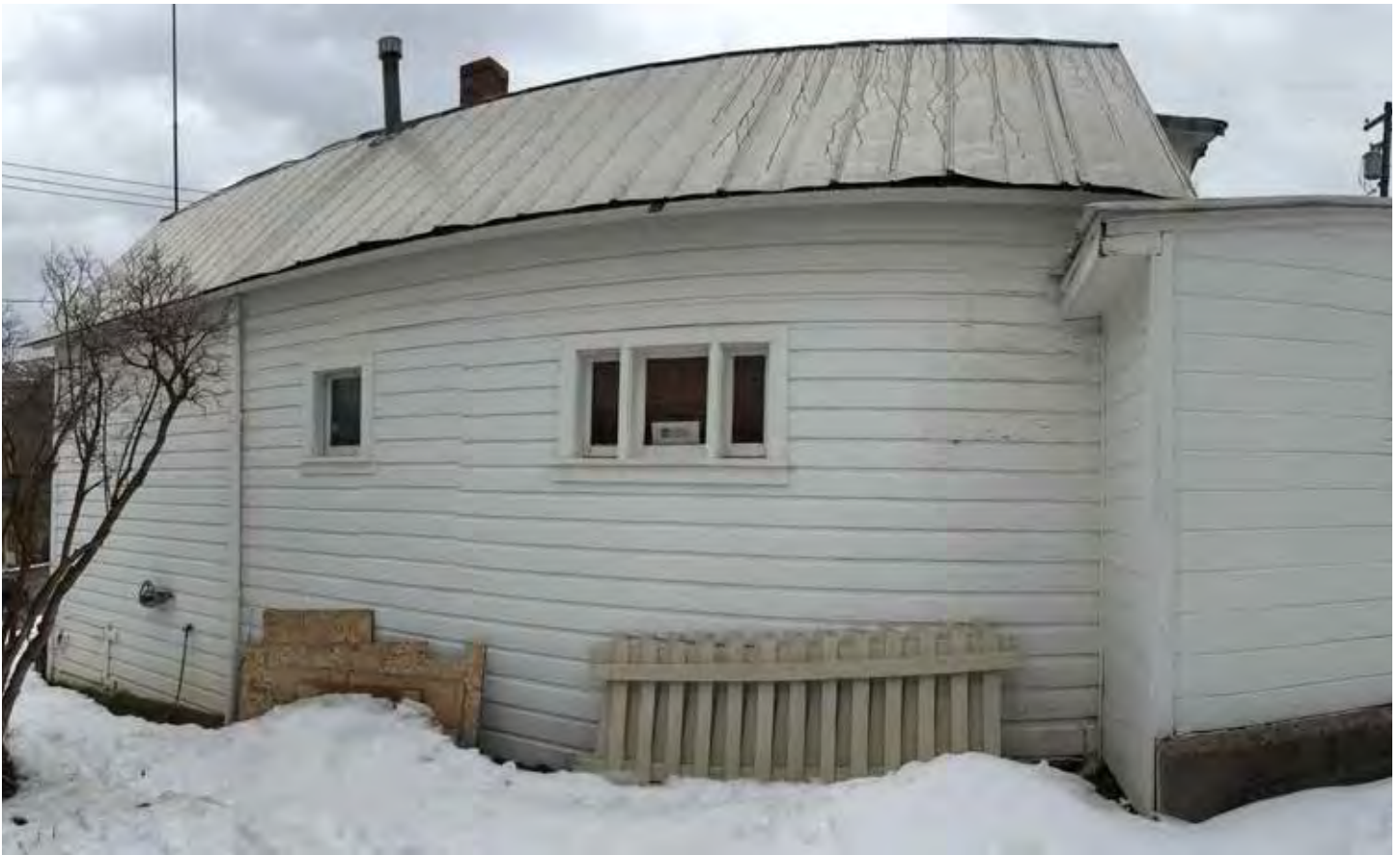
Photo #33: North Facade
