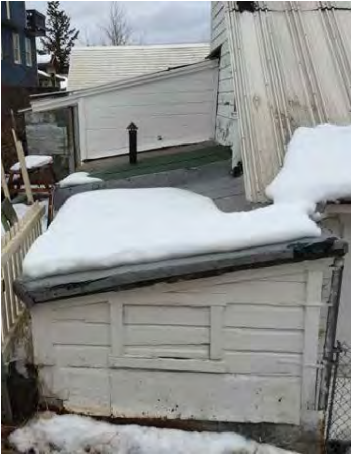
Photo #16: Roofs Over Coal/Storage/Rear Entry
