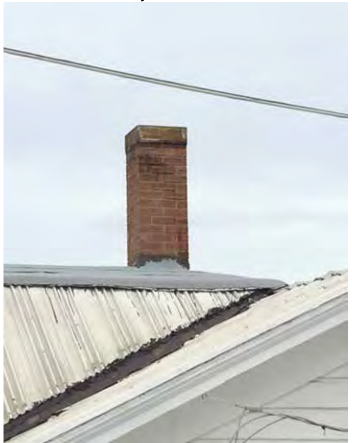
Photo #20: Chimney From South
