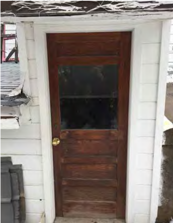
Photo #51: Door #2 From Exterior
