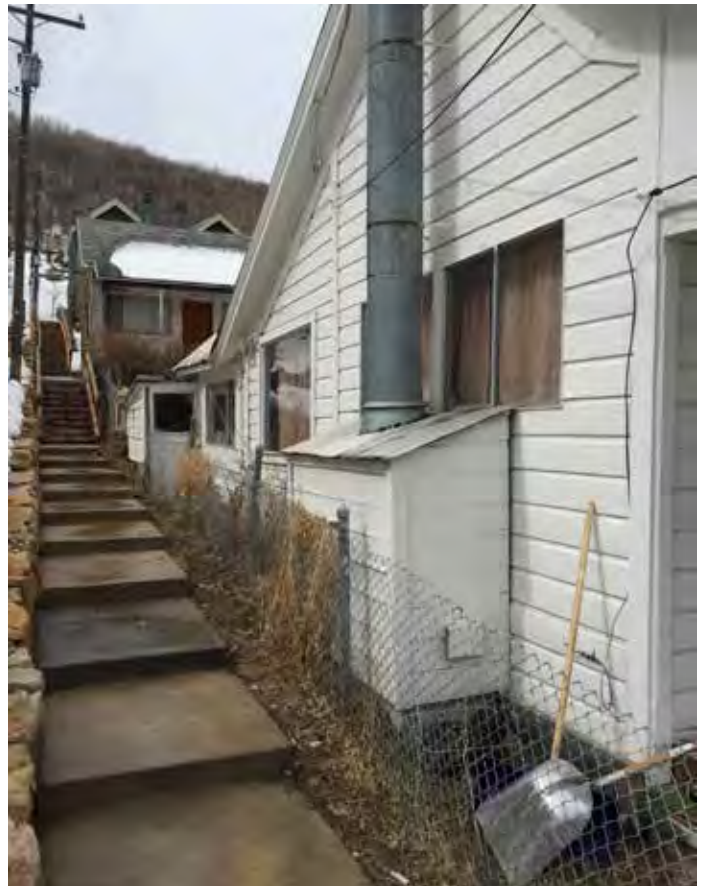
Photo #8: South Side Yard
