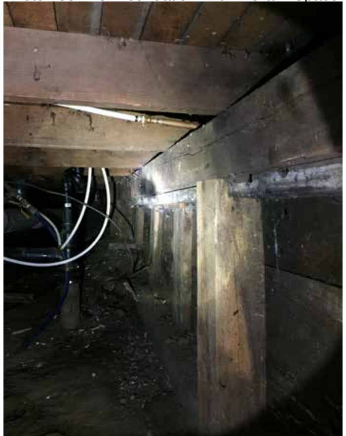
Photo #38: T.O. Foundation Within Crawl Space
