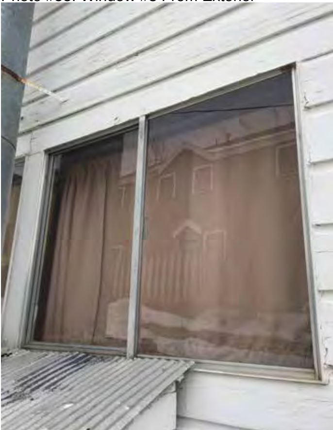
Photo #55: Window #3 From Exterior
