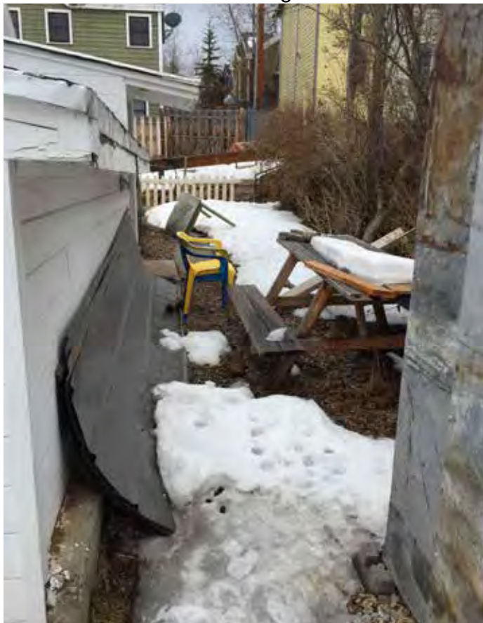
Photo #6: Rear Yard Grading
