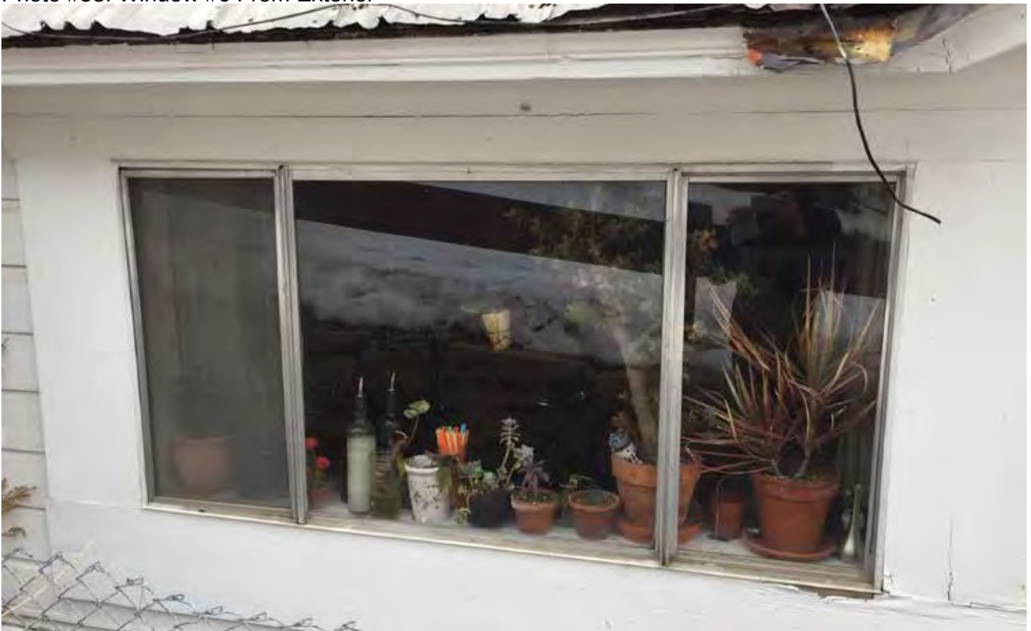
Photo #58: Window #6 From Exterior
