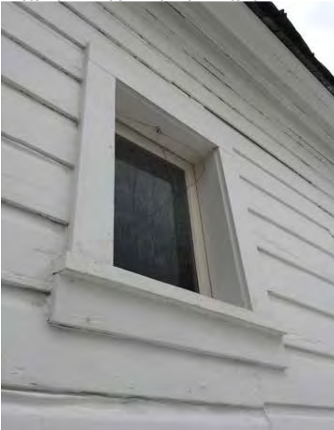
Photo #62: Window #10 From Exterior
