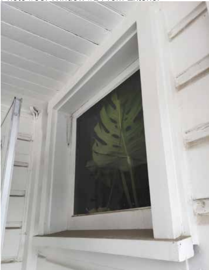
Photo #53: Window #1 From Exterior
