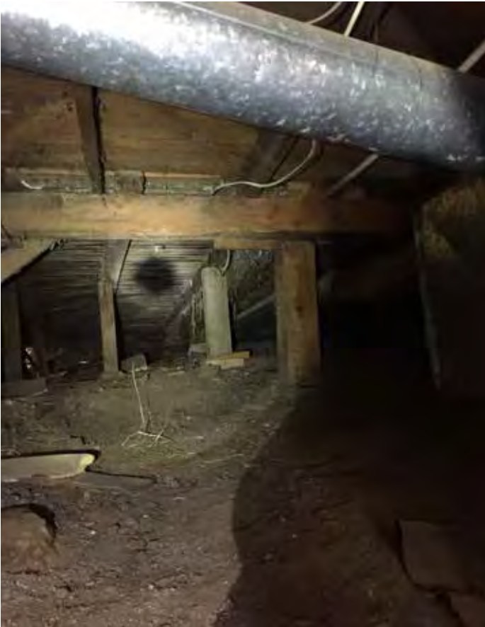
Photo #10: Posts & Beam Supporting Floor
