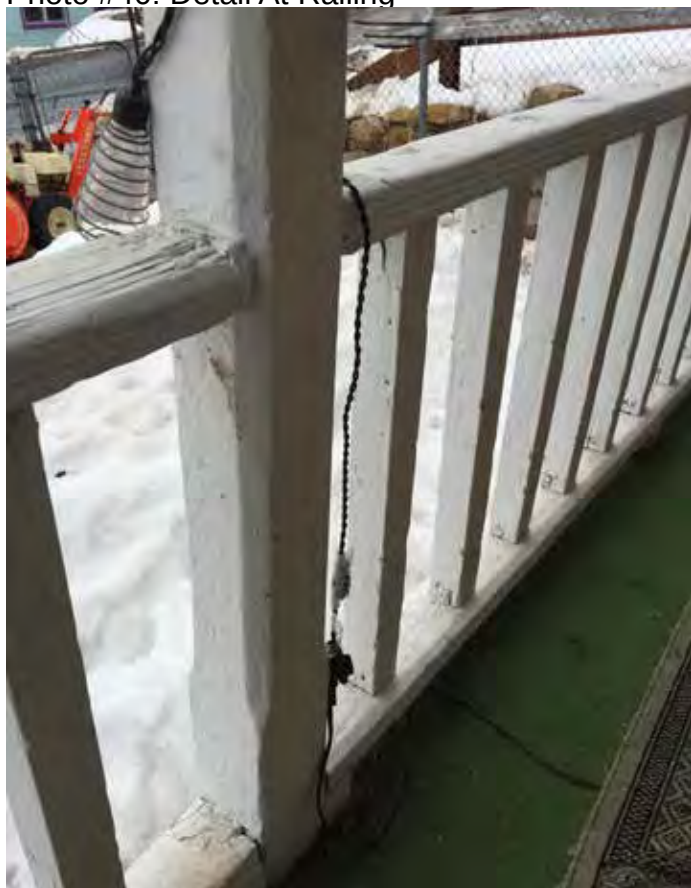
Photo #40: Detail At Railing
