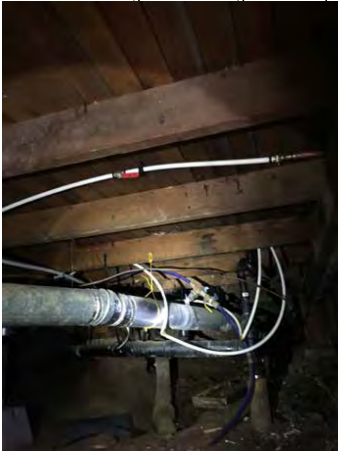
Photo #46: Ducting and Plumbing in Crawl Space
