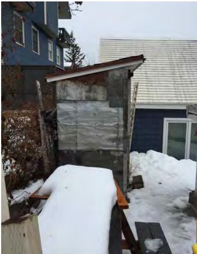
Photo #5: Shed Structure at Northwest Corner
