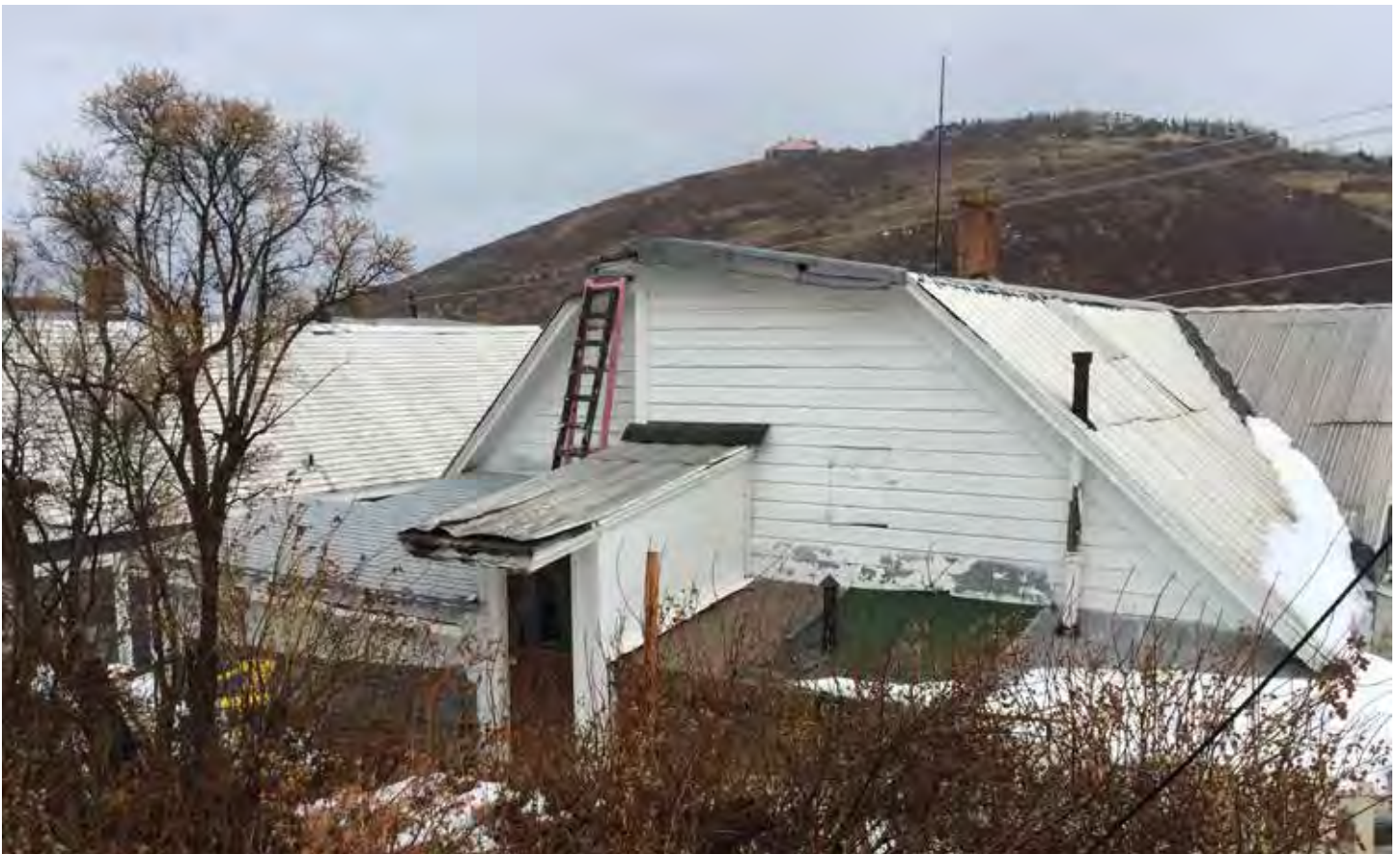
Photo #15: Roof From Rear With Overbuilds and Additions
