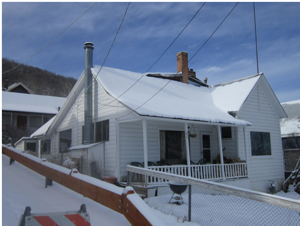
1003 Norfolk Avenue. Southeast oblique. November 2013.
