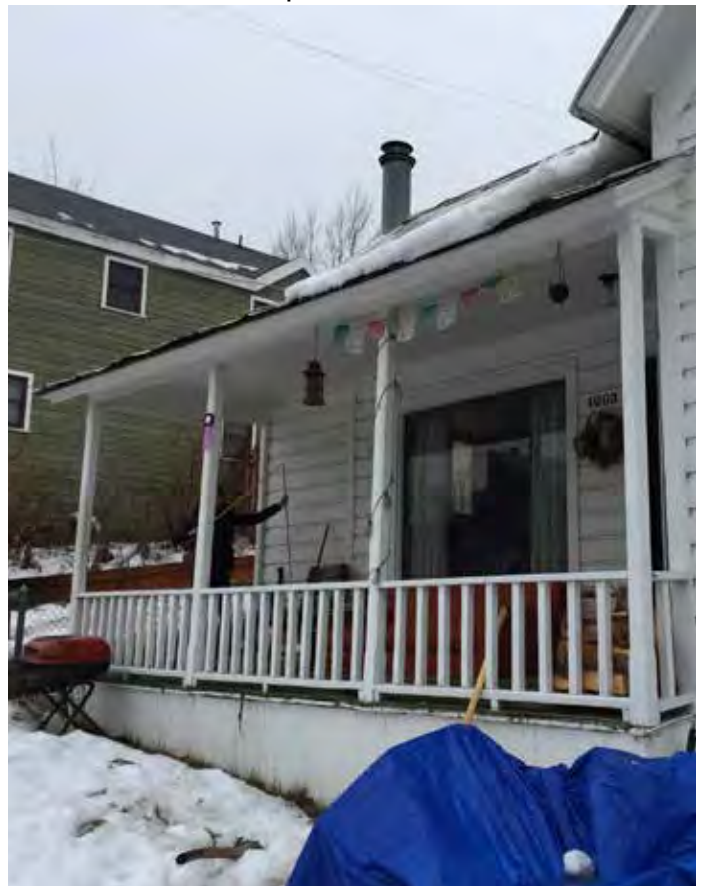
Photo #27: Close Up At Porch
