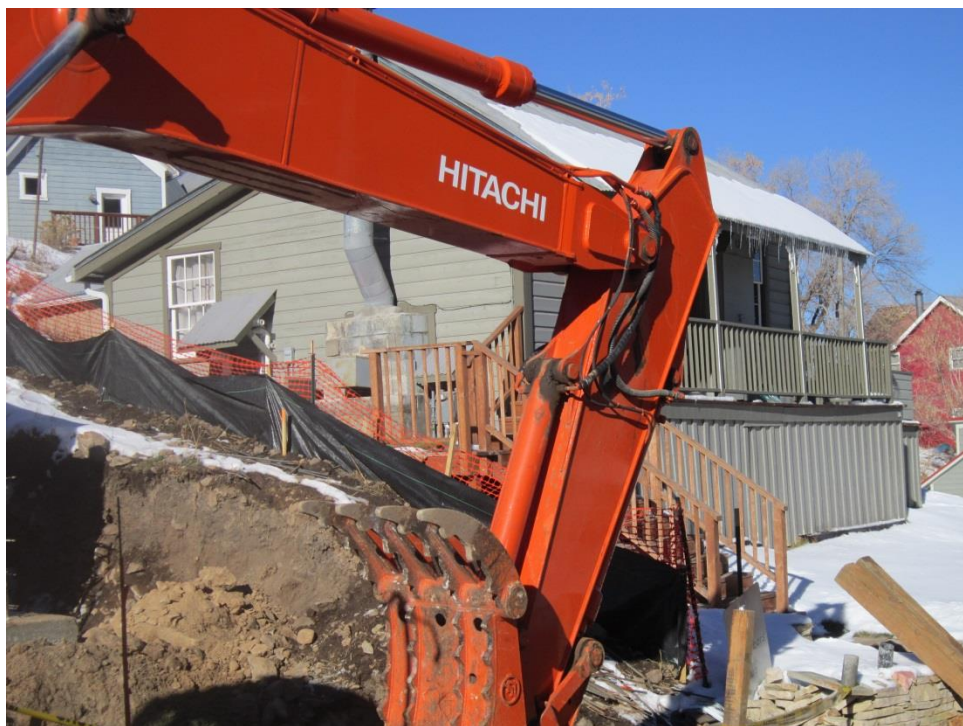
64 Chambers Avenue. Southeast oblique. November 2013.
