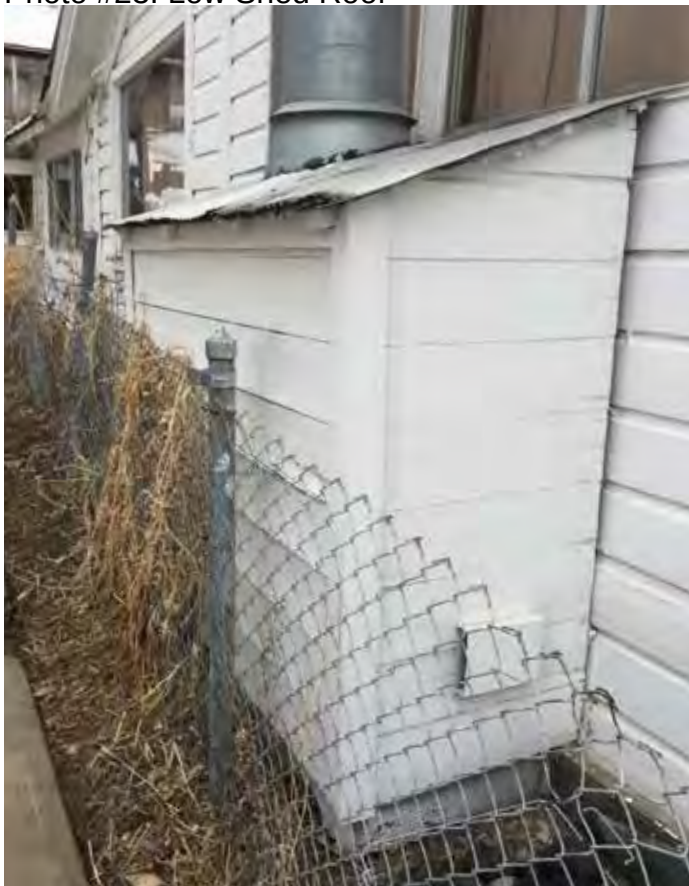
Photo #23: Low Shed Roof
