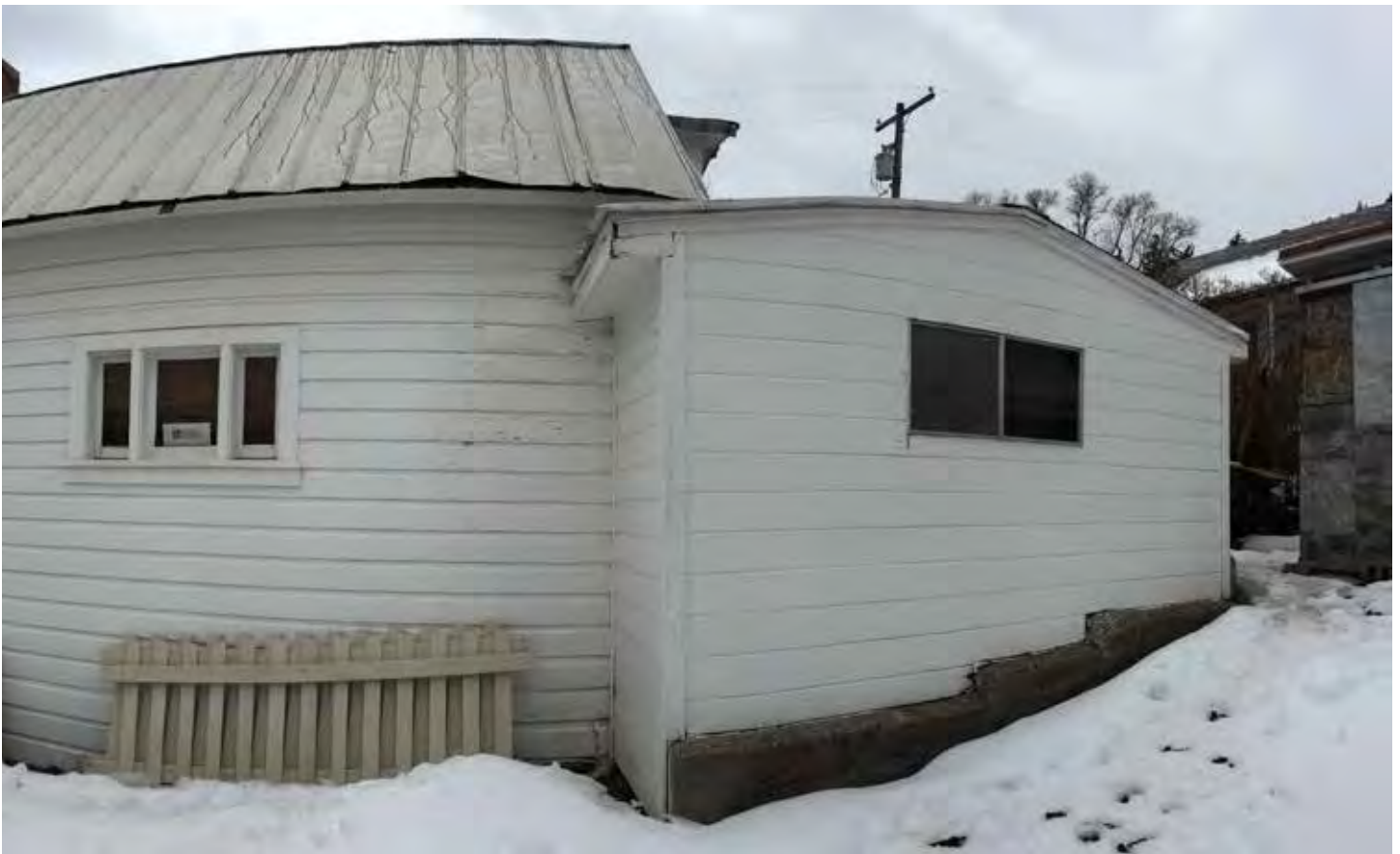
Photo #34: North Facade
