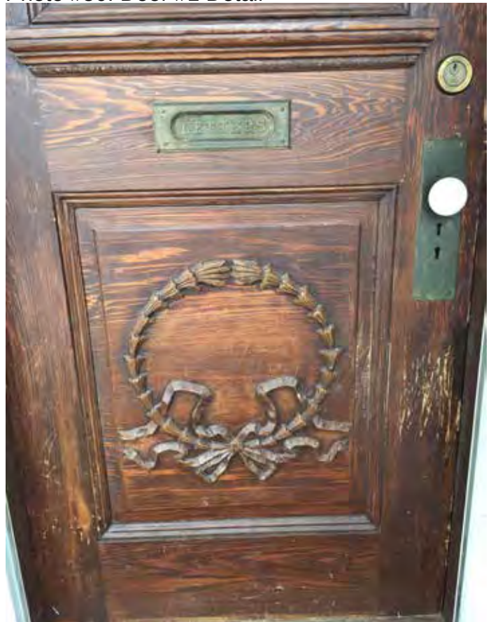
Photo #50: Door #1 Detail
