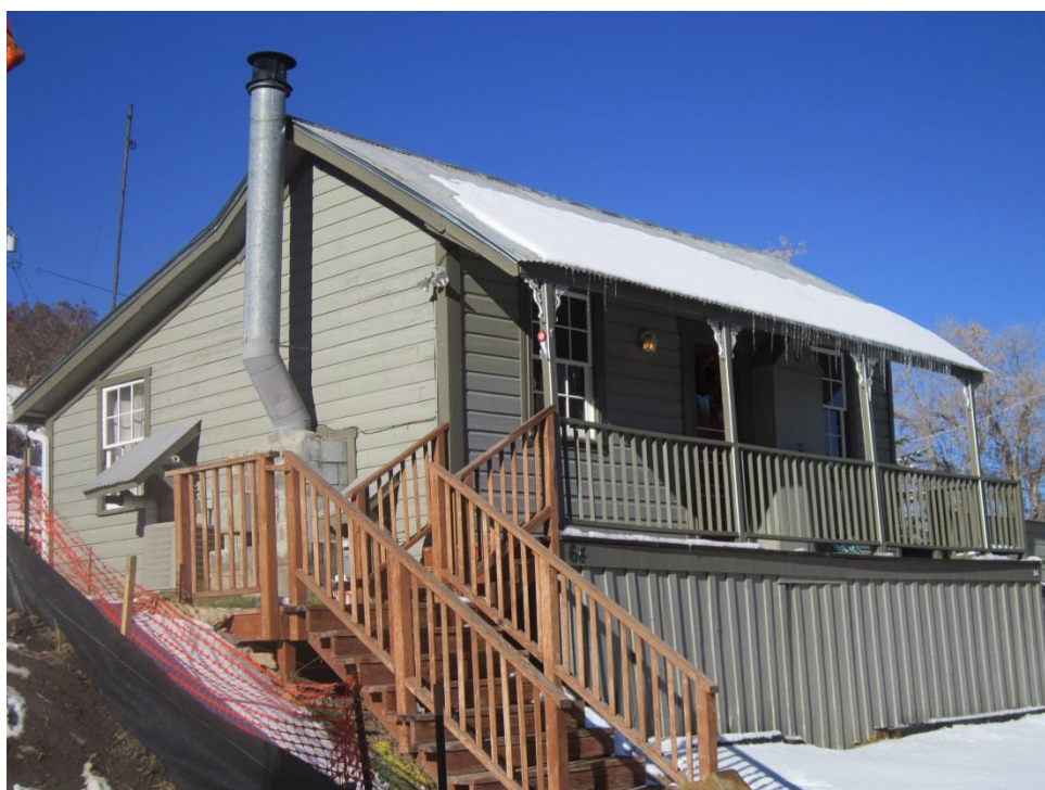
64 Chambers Avenue. Southeast oblique. November 2013.
