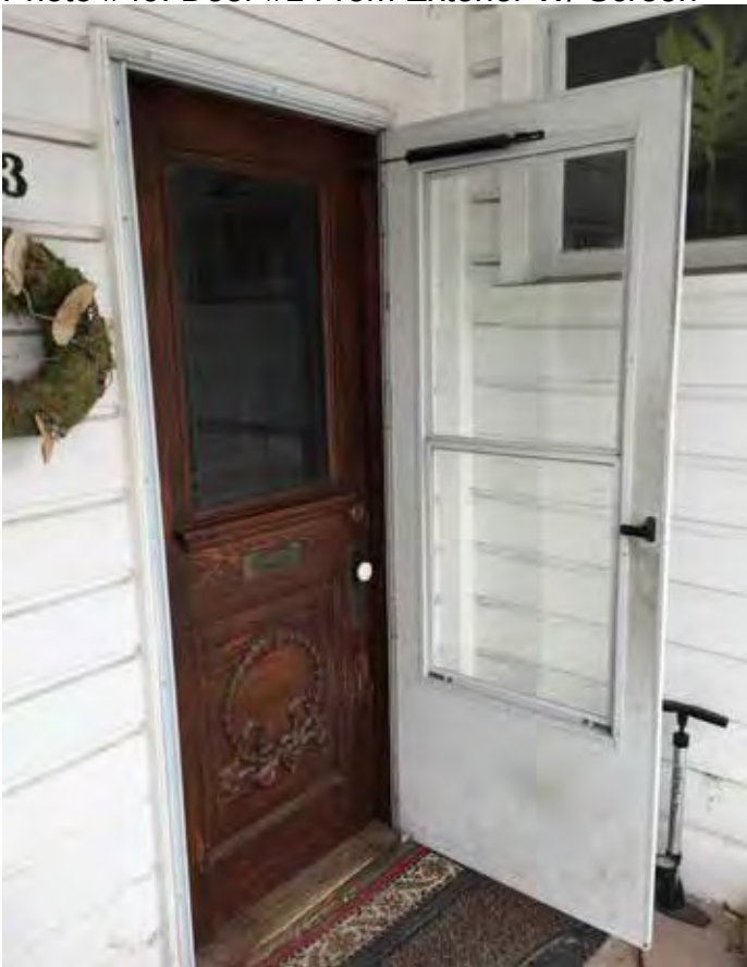
Photo #49: Door #1 From Exterior W/ Screen
