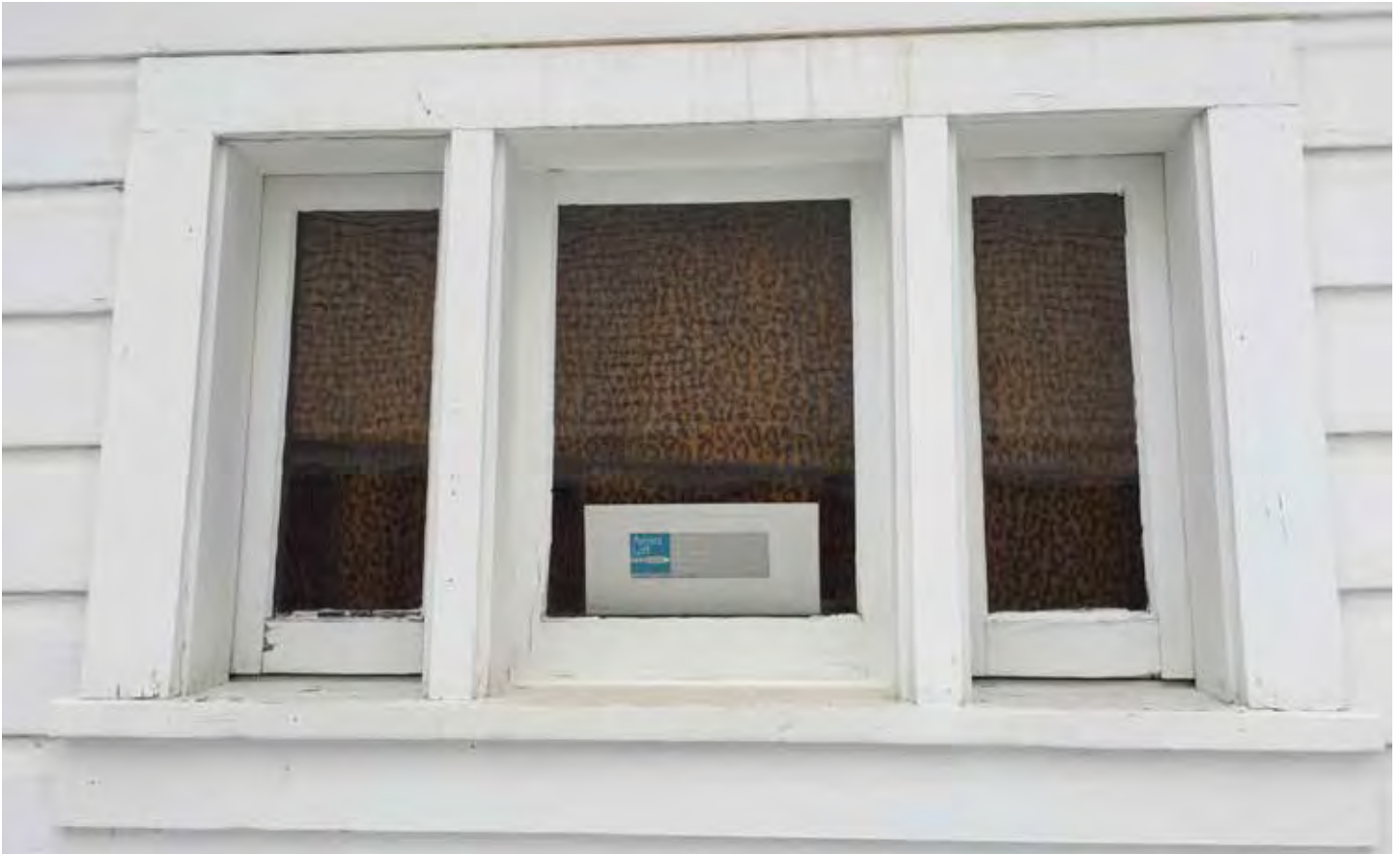
Photo #61: Window #9 From Exterior
