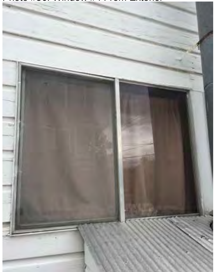
Photo #56: Window #4 From Exterior
