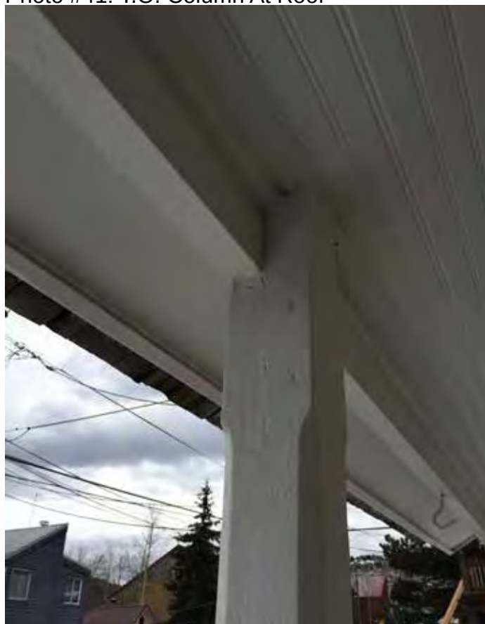
Photo #41: T.O. Column At Roof
