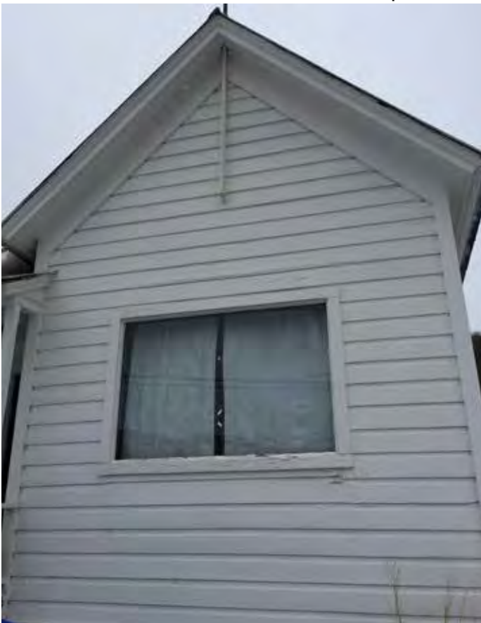
Photo #26: Gable Roofed Wall Close Up
