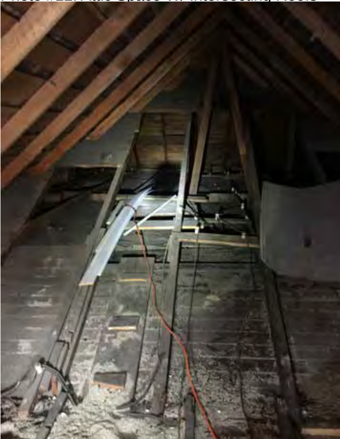
Photo #12: Attic Space W/ Intersecting Roofs
