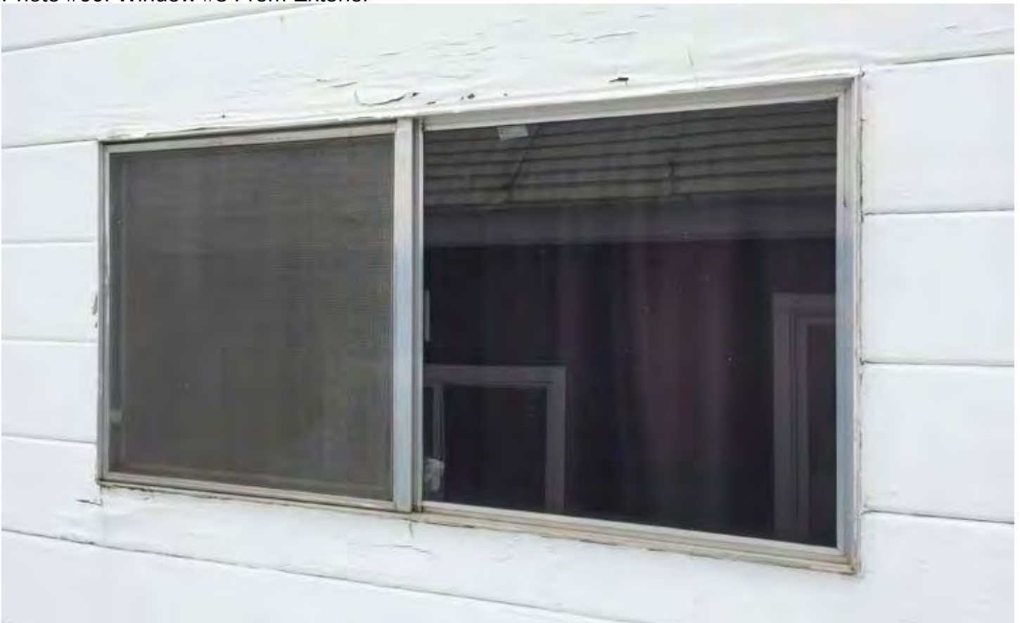
Photo #60: Window #8 From Exterior
