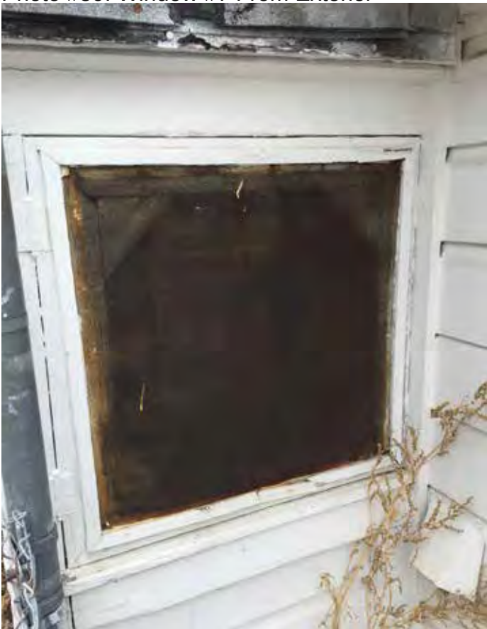
Photo #59: Window #7 From Exterior
