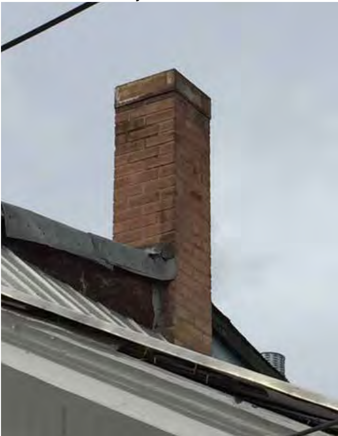
Photo #19: Chimney From Southeast
