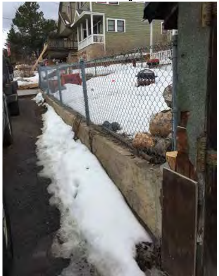
Photo #3: Concrete Retaining Wall & Fence
