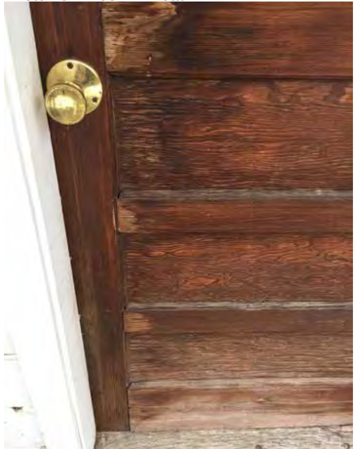
Photo #52: Door #2 Detail
