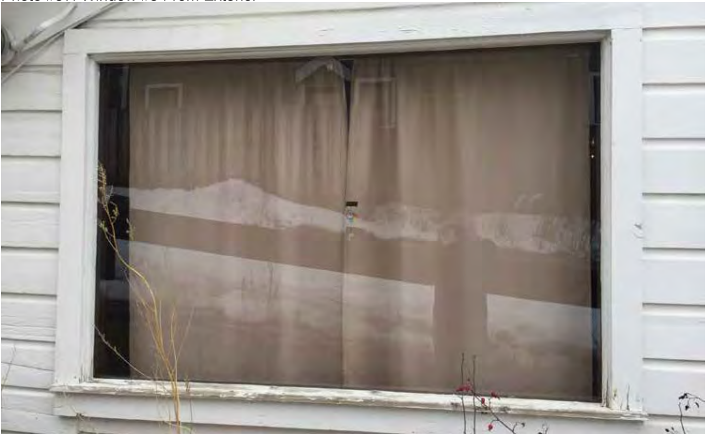
Photo #57: Window #5 From Exterior
