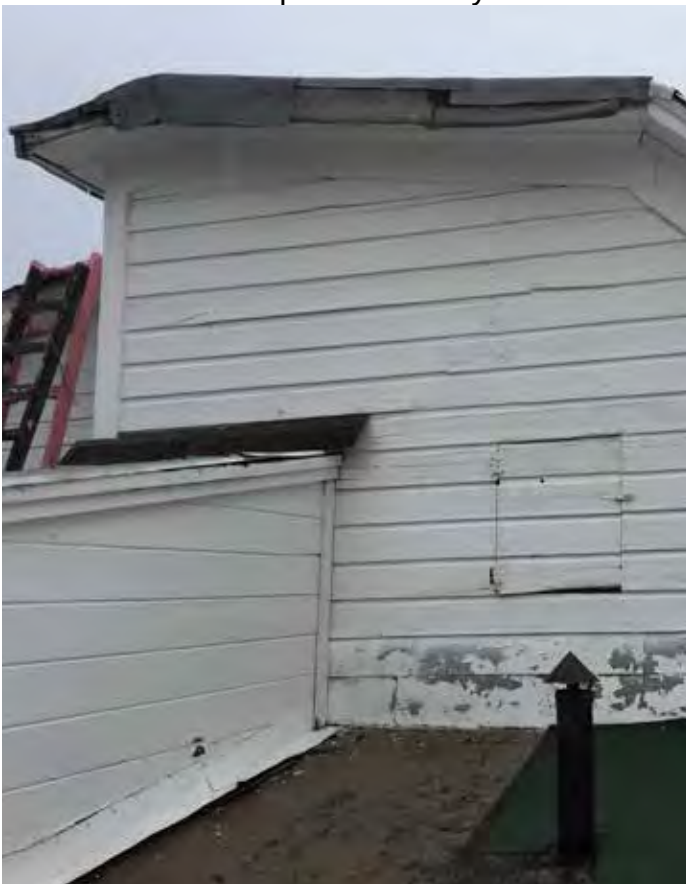
Photo #31: Close Up At Attic Entry
