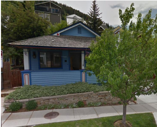
Figure 1: Photo of the Structure prior to construction
