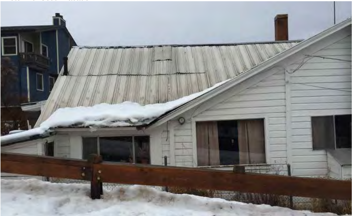
Photo #29: South Facade
