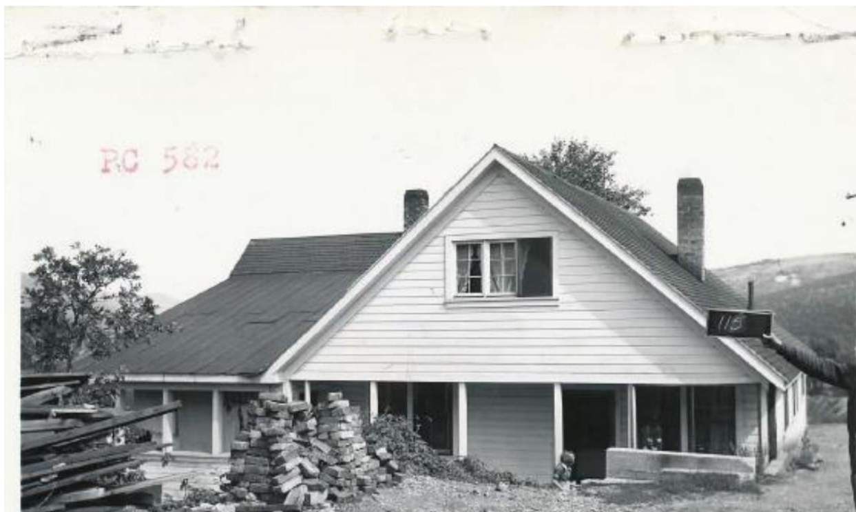
Figure 3: 1940s-era tax photo of 218 Sandridge Road, taken from the Historic Site Form.
