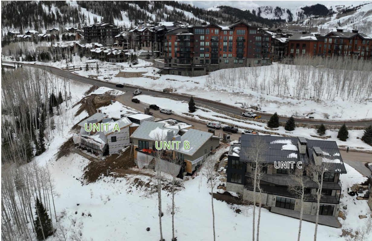
Figure 4: Applicant's Aerial View of Units A and B Looking Southwest
