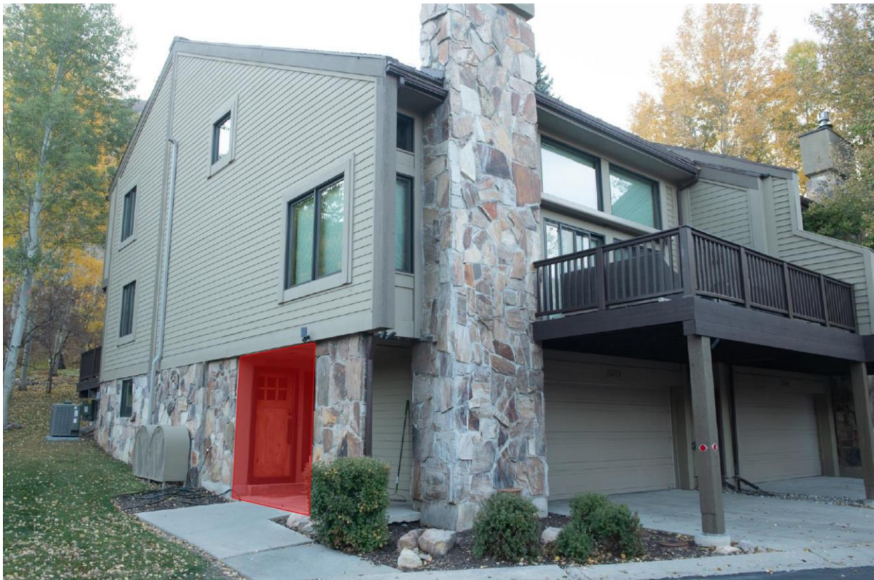
Figure 1: 2380 Good Trump Court viewed from the north. The area shaded in red is proposed to be enclosed and converted from limited common area to private ownership to create additional space in the entrance hall of the unit.
