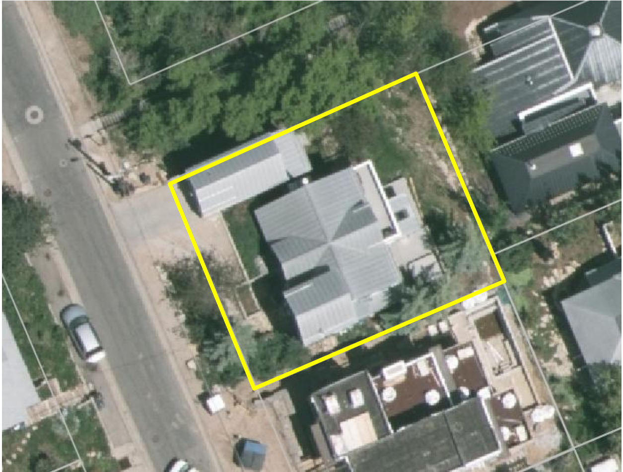
Image 1: Aerial view of 368 Woodside Avenue
