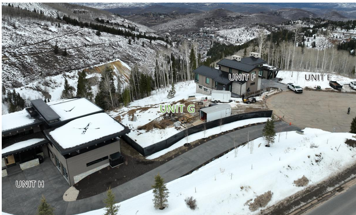
Figure 3: Applicant's Aerial View of Unit G Looking Northeast
