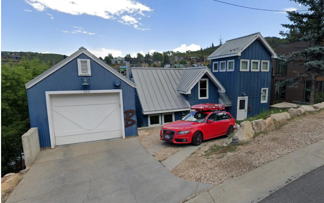
Image 2: Existing home at 364 and 368 Woodside Avenue
