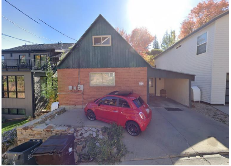
91 King Road viewed from King Road, image from Google.
