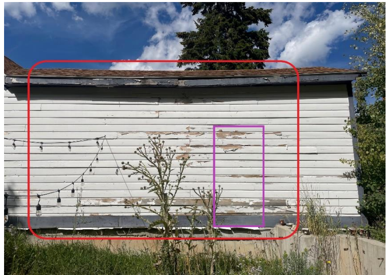
Figure 4: View of rear wall showing siding materials to remain as an interior accent wall (red) and proposed location of interior door (purple).
