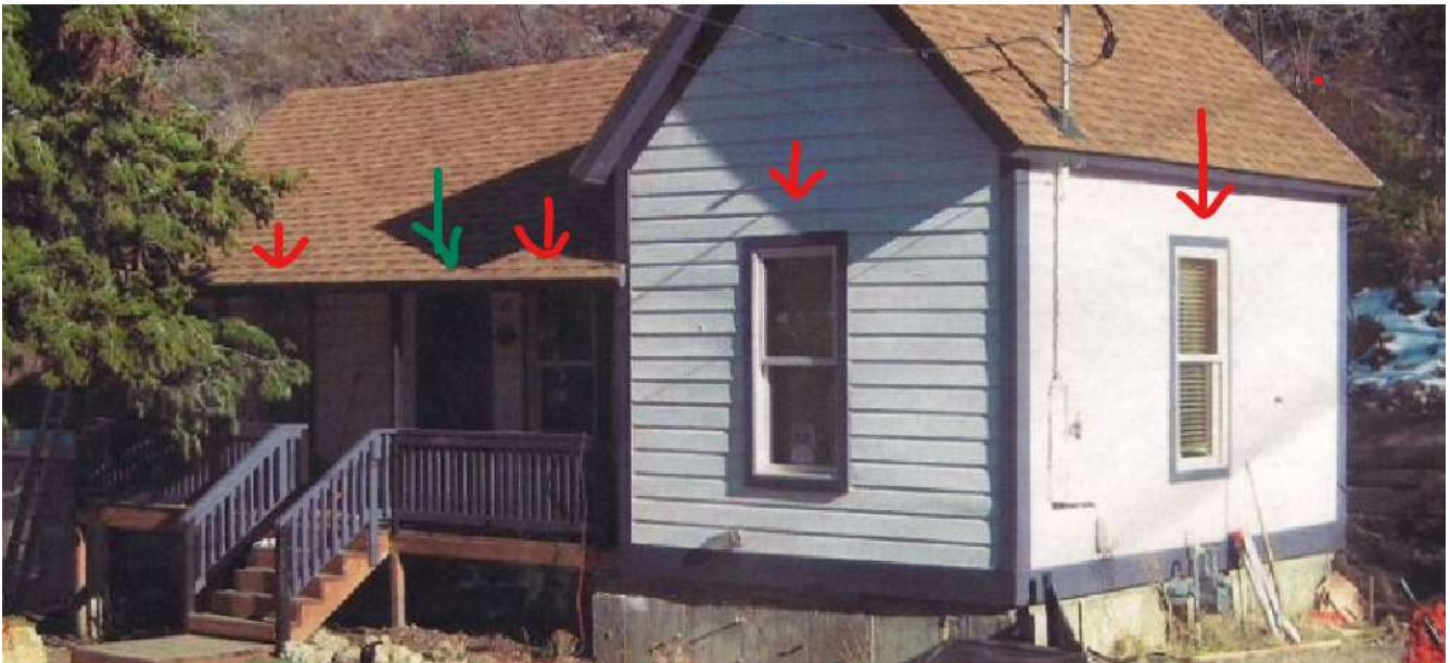
DOWNHILL SIDE ELEVATION WINDOW (MARKED IN RED) BELOW
