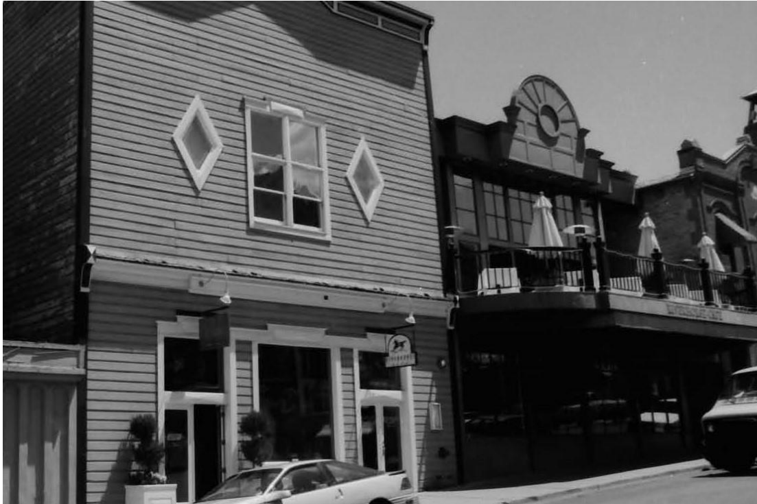
Figure 1: 1995 photograph showing the open balcony.
