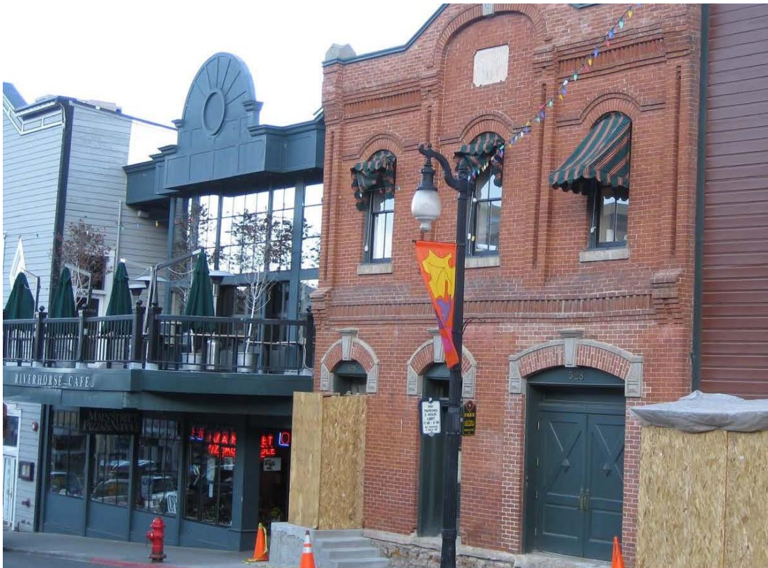
Figure 2: Photograph showing open balcony and neighboring Landmark Structure at 528 Main Street. Second story facade of building is shown to sit behind the facade planes of the abutting Landmark Structures.
