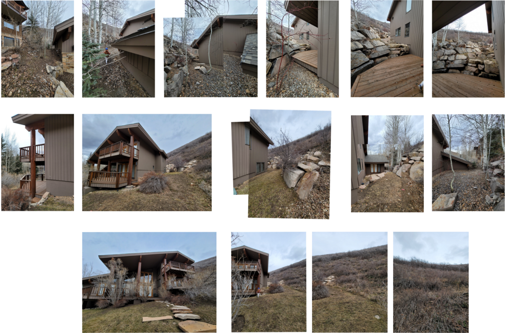
Figure 1: Site photos provided by Applicant.
