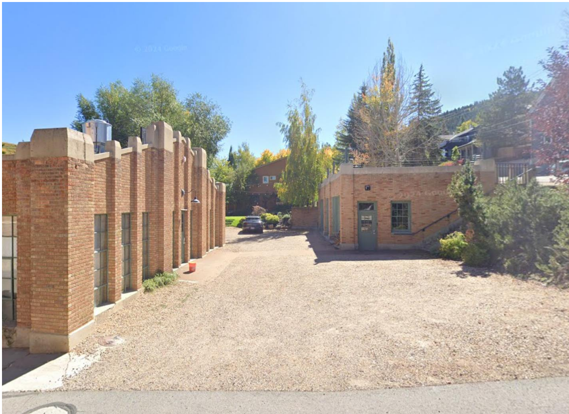
Figure 4: Rear portion of the property at 1167 Woodside Avenue, including a five-car garage (on the right) constructed in 1996.
