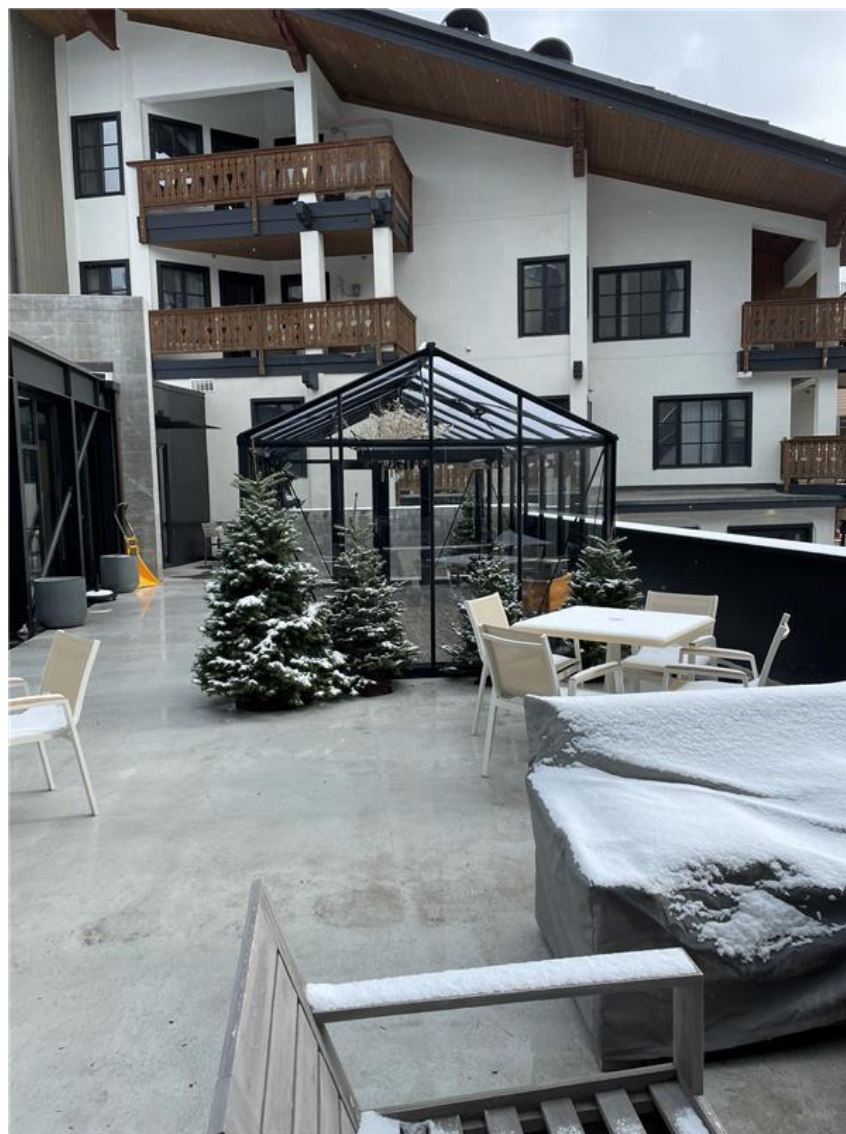
Figure 3: Constructed Temporary Structure Without Approvals (photo taken by Staff)
