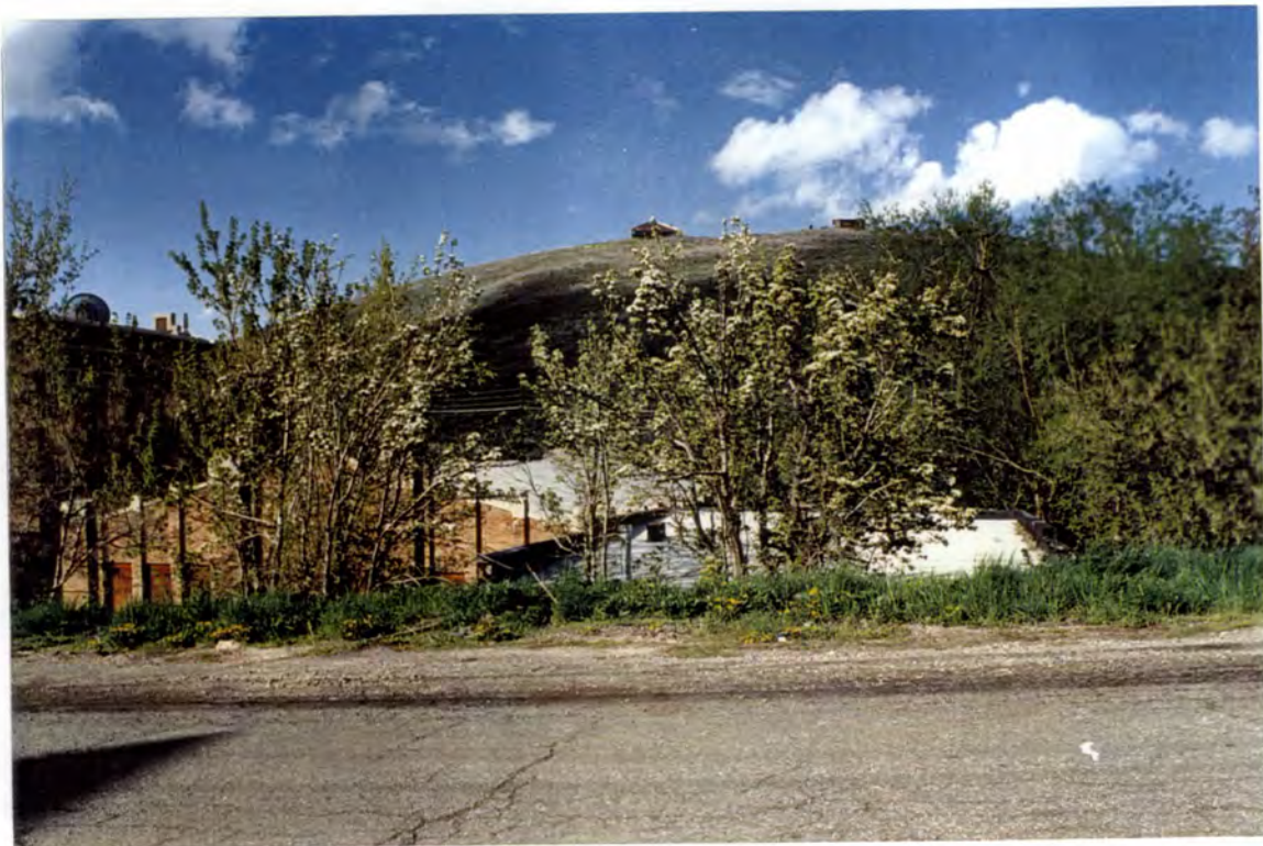
WEST FACADE (NORFOLK AVE)
