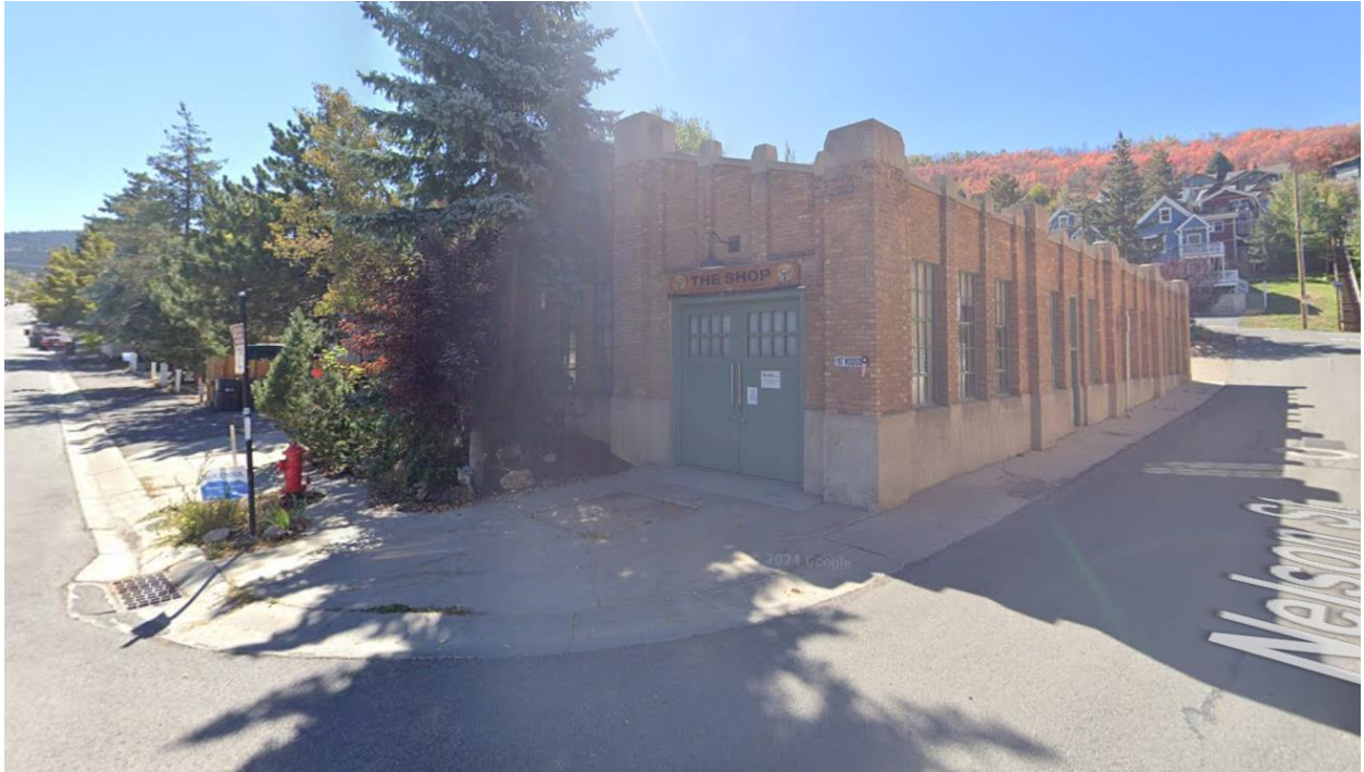
Figure 3: Front view of 1167 Woodside Avenue from the northeast corner of the property.
