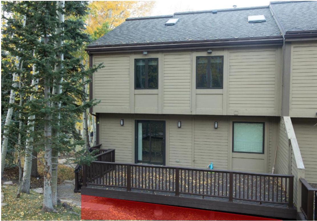
Figure 3: Rear view of 2366 Good Trump Court. The rear view of the unit would remain unchanged with the proposed Plat Amendment. The property owner proposes changes to a rear bedroom on the ground level of the unit, which is below grade at the rear of the site and occupies roughly the same space as the area highlighted in red.
