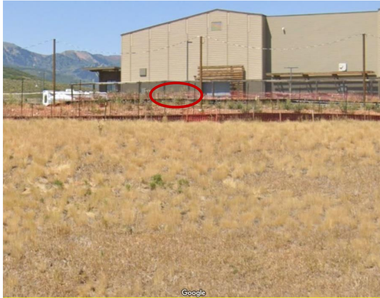
View of Bay 1 from I-40 taken from Google Street View. Approximate location of restroom trailer shown by red oval, indicating that at most the very top of the trailer will be visible.
