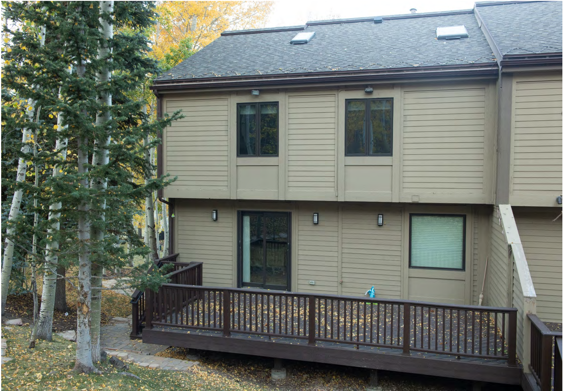
Queen Eshter Village No. 1 Unit 1 – looking Westerly
