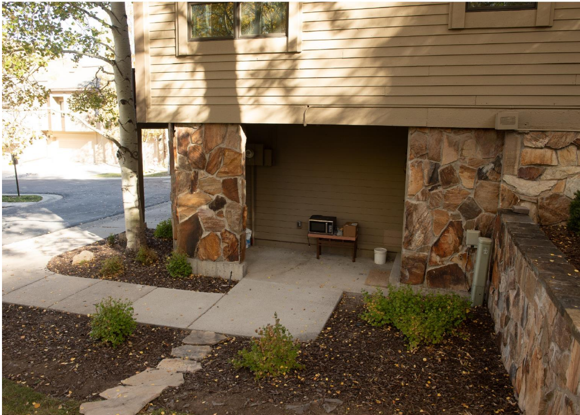
Figure 1: This 51-square-foot front porch at 2366 Good Trump Court is currently platted as limited common ownership area. The Applicant seeks a Plat Amendment to convert the area to private ownership and proposes to enclose the area to provide more space in the entrance hall of the unit.
