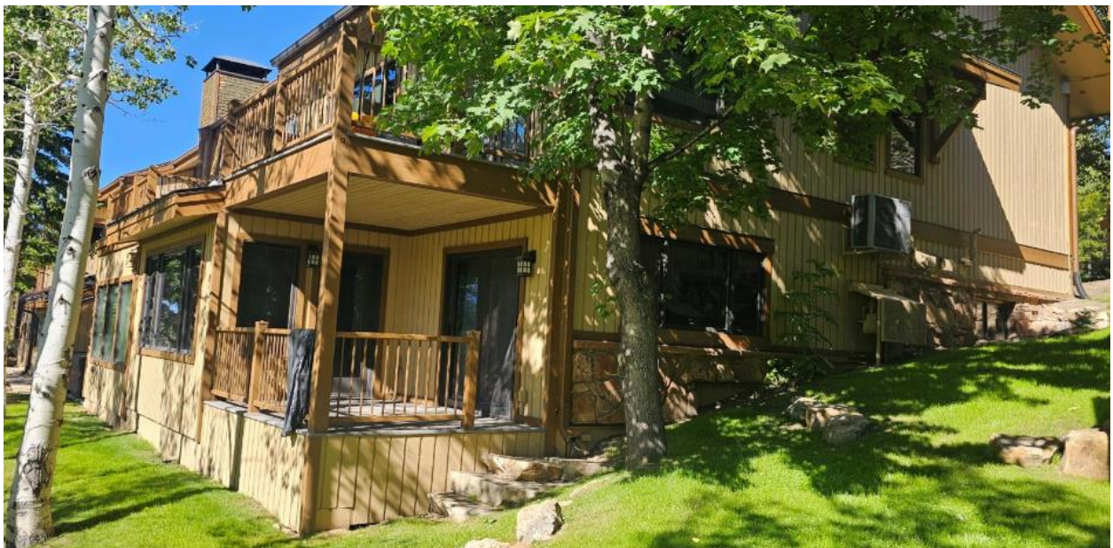
LITTLE BELLE CONDOMINIUMS UNIT 4 LOOKING NORTHEAST
