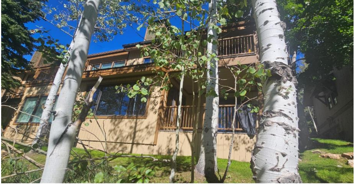
LITTLE BELLE CONDOMINIUMS UNIT 4 LOOKING EAST (BACK OF BUILDING)
