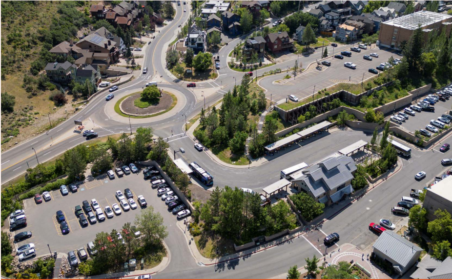
Before: Flagpole and North Marsac parking lots
