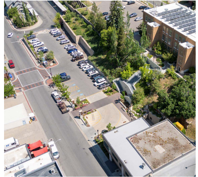
Swede Alley looking North. Photo from Park City Municipal Corporation.
