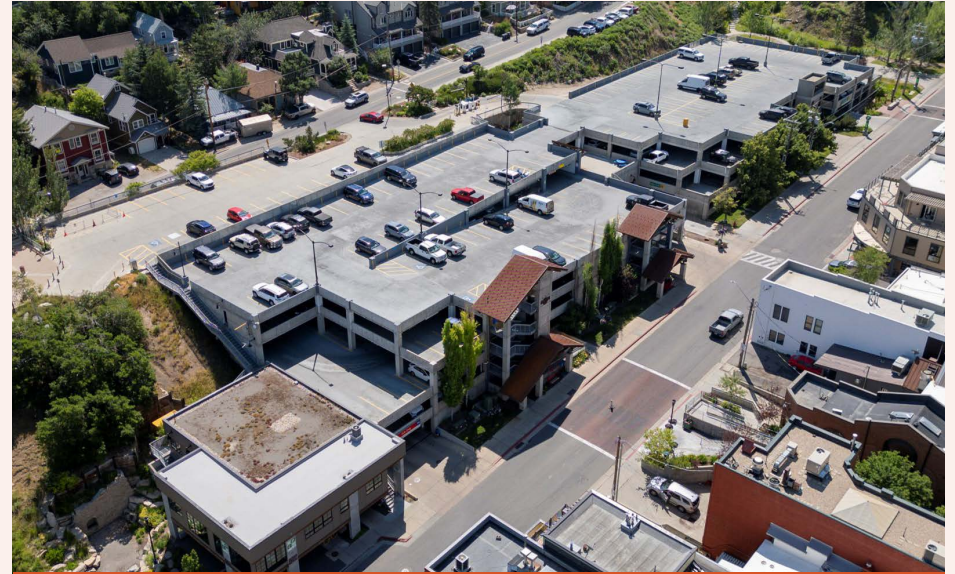
Before: China Bridge Parking Garage
