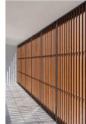
LOUVER SCREEN: THERMALLY MODIFIED WOOD
