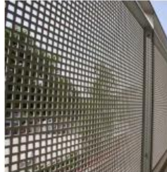
MECHANICAL SCREENING: PERFORATED METAL TO MATCH FASCIA
