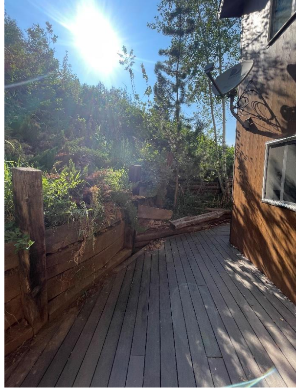
Figure 1 & 2: Applicant's photos showing existing failing wood retaining wall at 430 Deer Valley Loop.
