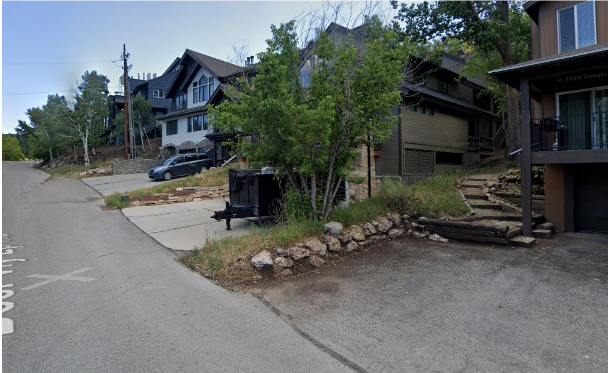
Figure 5: Google Maps screenshot showing existing stacked stone and concrete retaining walls at nearby properties along Deer Valley Loop Road.
